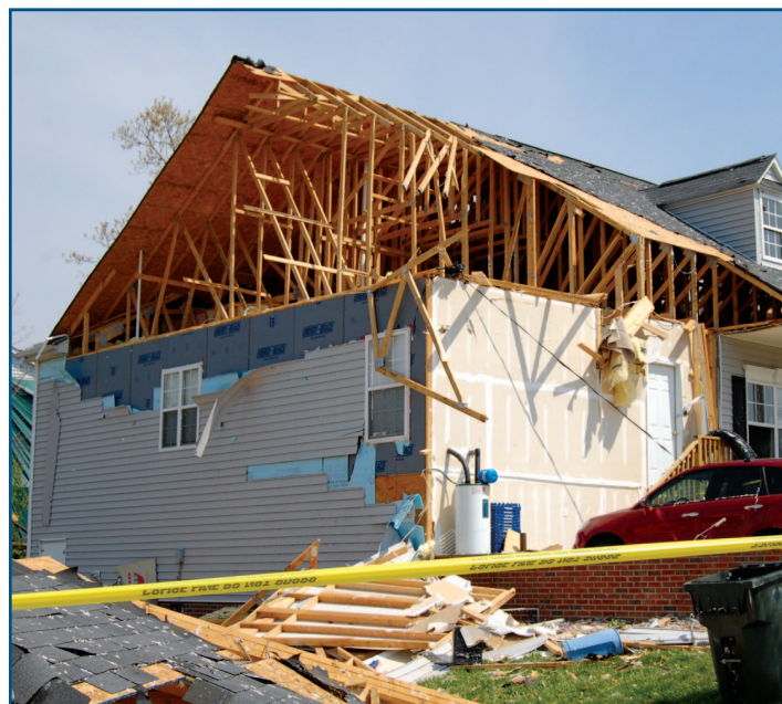
Figure 1: A house that lost large sections of the roof and the garage due to internal pressurization.
