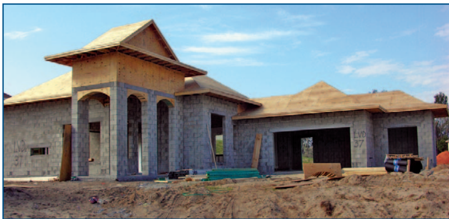
CMU was used for the exterior walls at this house under construction (New Smyrna Beach, FL).
