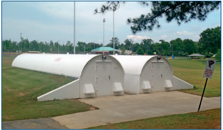
View of a partially below-grade community safe room (Brookwood, AL).
