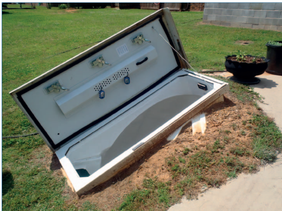
View of a pre-fabricated safe room that serves a residence (Tuscaloosa, AL).
