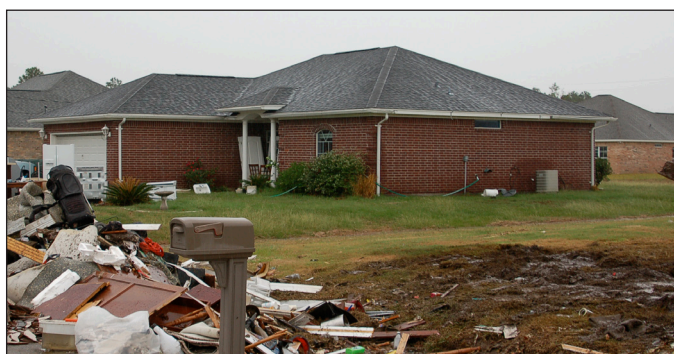
Figure 1. Bridge City, TX, homes were flooded during Ike, even though they were constructed outside the SFHA and in Zone B. The flood level was approximately 4' above the closest BFE.
