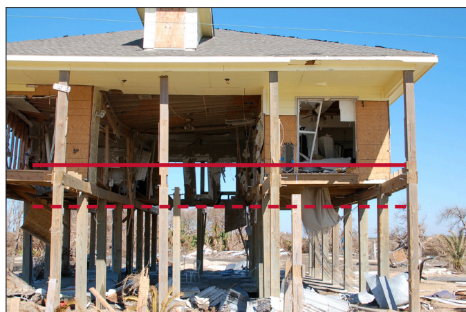
Figure 2. Bolivar Peninsula, TX, V-zone house constructed with the lowest floor (bottom of floor beam) at the BFE (dashed line). The estimated wave crest level during Ike (solid line) was 3 to 4' above the BFE at this location.
