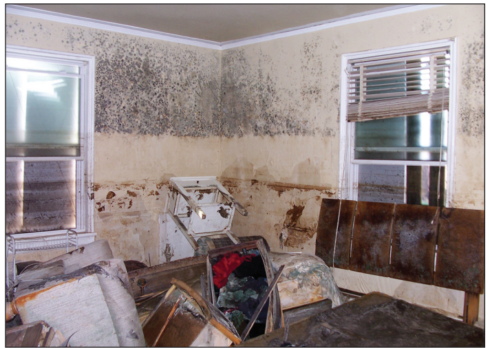
Figure 6. Other concerns when flood levels rise above the lowest floor are mold and biological/chemical contamination. These may render an otherwise repairable building unrepairable, or will at least make the cleanup, restoration, and repairs much more expensive and time-consuming.
