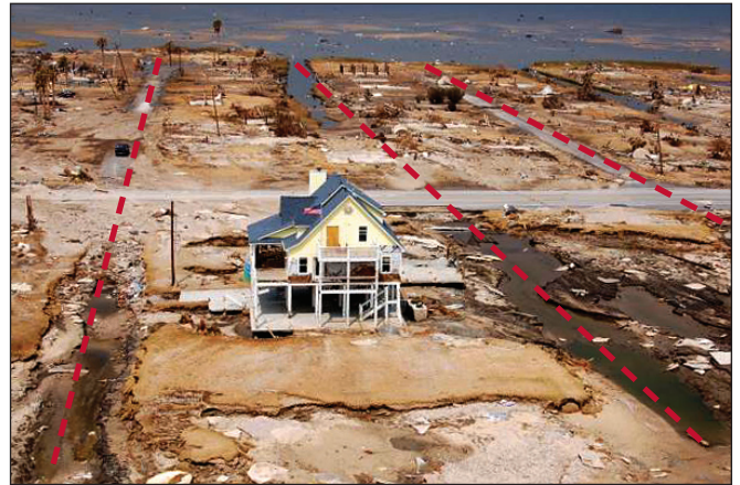
Figure 9. Linear scour and erosion patterns aligning with canals and roads (Bolivar Peninsula, TX, Hurricane Ike).
