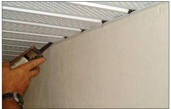
Figure 4. Applying dabs of sealant.
