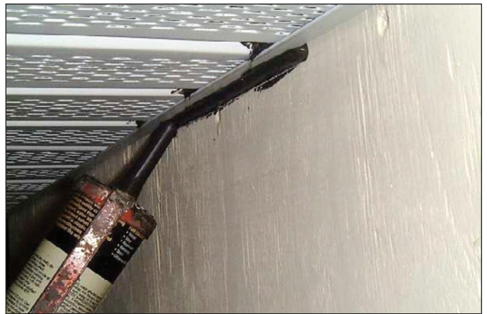
Figure 3. Applying a bead of sealant. (Note: Black sealant was used so that it would be visible in the photograph. Normally a matching sealant color would be used.)
