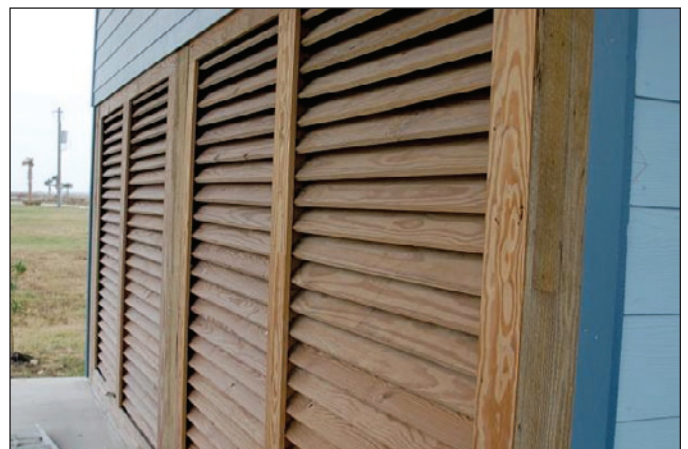
Figure 1. Wood louvers installed beneath an elevated house in a V zone are a good alternative to solid breakaway walls.
