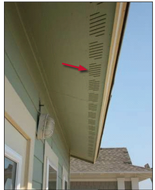
Figure 6. Fiber cement soffit with ventilation slots (red arrow).
