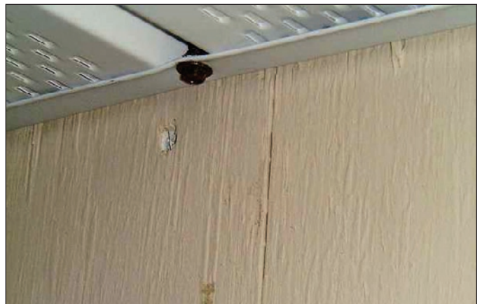
Figure 5. Screws through wall channel.
