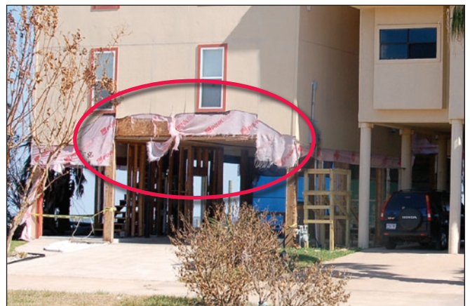
Figure 3. NFIP-compliant breakaway wall construction.
