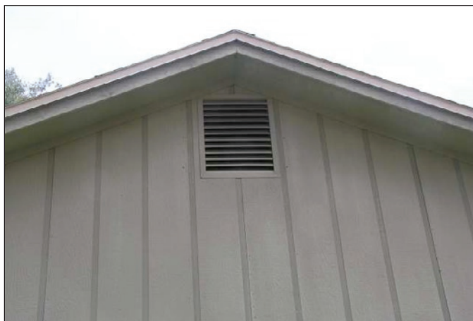
Figure 9. Gable end vent.
