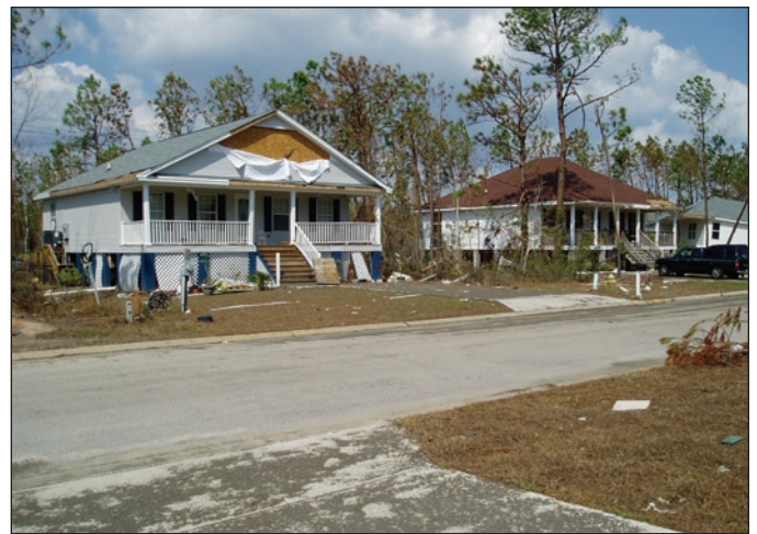
Figure 10. The site on the left is mapped Zone AE, and lies directly along the Gulf of Mexico shoreline. Limited obstructions to waves indicate the site could be classified as a Coastal A zone. The site on the right is over 1/2 mile from the Gulf shoreline, is mapped as Zone AE, and has a base flood stillwater level sufficient to support >1.5' wave heights – but obstructions to waves (e.g., trees and other buildings between the site and the shoreline) and distance from the source of flooding would indicate the area is not a Coastal A zone.
