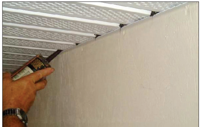
Figure 4. Applying dabs of sealant.
