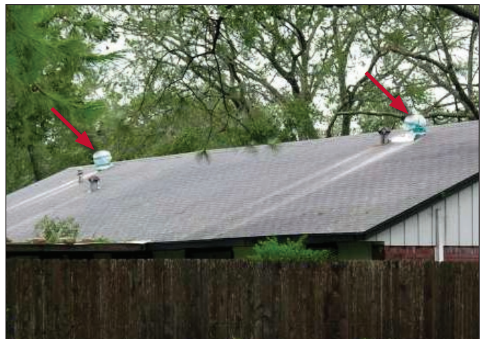
Figure 14. Plastic wrapped turbine.
