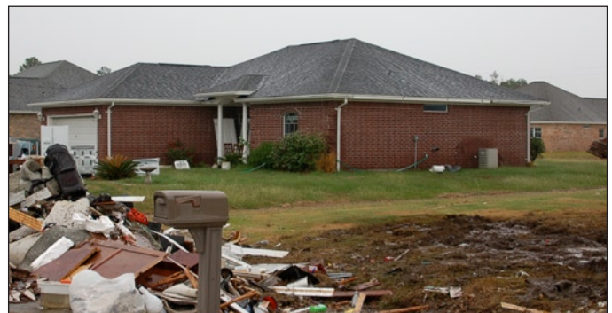
Figure 1. Bridge City, TX, homes were flooded during Ike, even though they were constructed outside the SFHA and in Zone B. The flood level was approximately 4' above the closest BFE.
