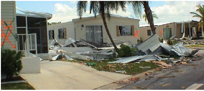
Glazing damage caused by windborne debris from nearby damaged homes and attachments.
