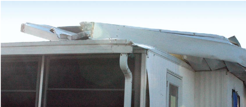
These photos show the failure of an attached porch roof. Uplift forces acting on the roof of the attached porch caused it to lift. When the roof lifted, it destroyed the porch roof and damaged the roof over the original home. Where open areas exist, as in the porch shown, the addition must resist uplift forces that act on the top and underside of the roof.
