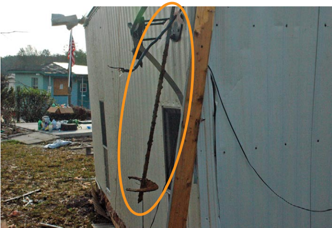
This 4-foot-long ground anchor with a 6-inch diameter helix pulled out of the soil. Soils in the area consisted of loose sands. Longer anchors with larger diameter helices would have been a better choice for this soil type. The anchor spacing at this home was approximately 10 feet.
