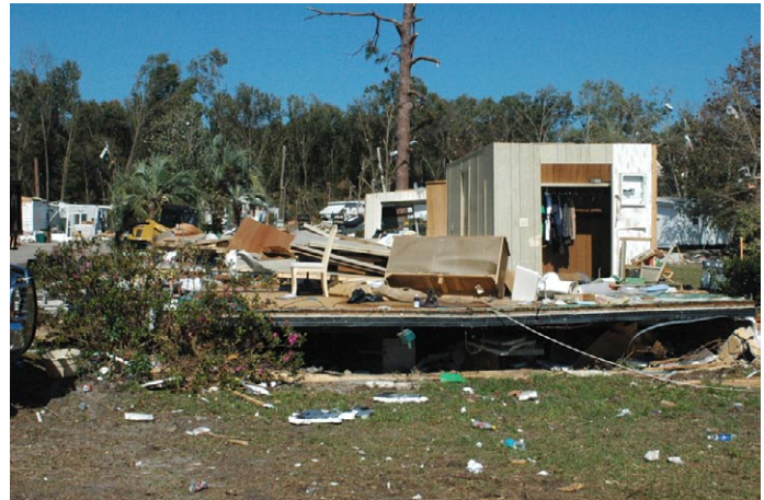
This home, constructed before 1976, was destroyed in the February 2007 tornadoes.
