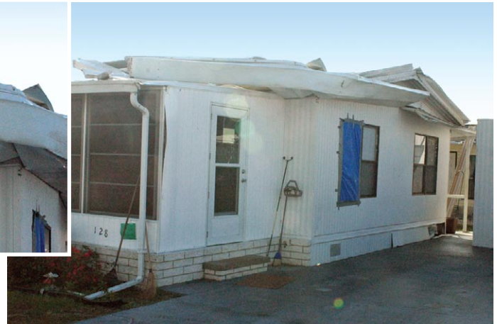
These photos show the failure of an attached porch roof. Uplift forces acting on the roof of the attached porch caused it to lift. When the roof lifted, it destroyed the porch roof and damaged the roof over the original home. Where open areas exist, as in the porch shown, the addition must resist uplift forces that act on the top and underside of the roof.
