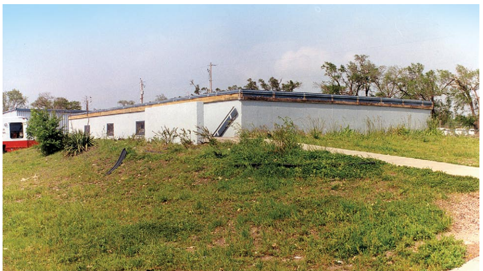
View of a partially below-grade community shelter at a manufactured home community (Wichita, KS).
