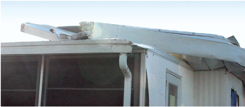
These photos show the failure of an attached porch roof. Uplift forces acting on the roof of the attached porch caused it to lift. When the roof lifted, it destroyed the porch roof and damaged the roof over the original home. Where open areas exist, as in the porch shown, the addition must resist uplift forces that act on the top and underside of the roof.
