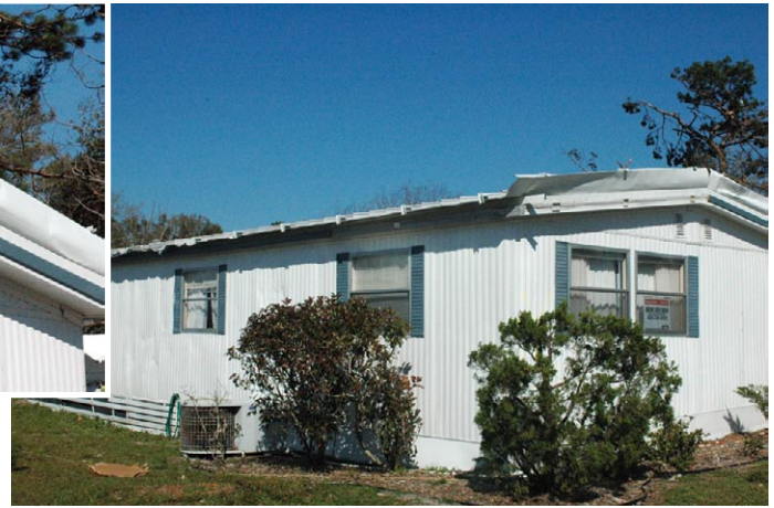
These photos shows the failure of a “reroof.” Uplift forces at the edges of the roof caused portions of the added roof to lift and peel off the manufactured home.
