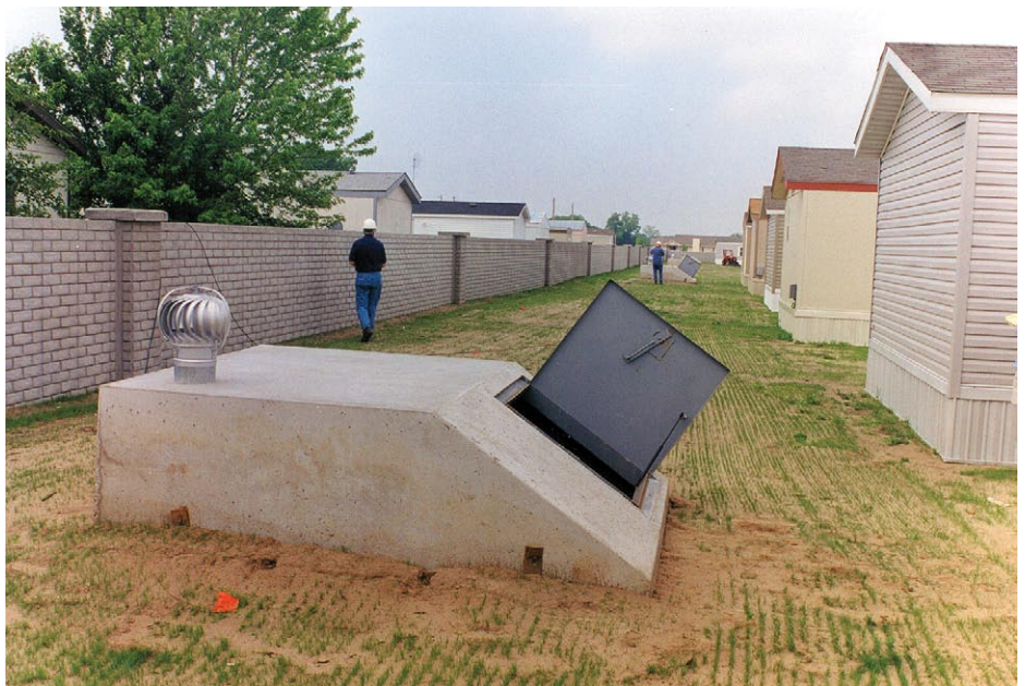
View of a pre-fabricated shelter that serves a few manufactured homes (Wichita, KS).
