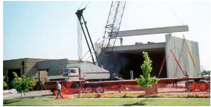
Community storm shelter being constructed to FEMA 361 criteria in Wichita, Kansas.
