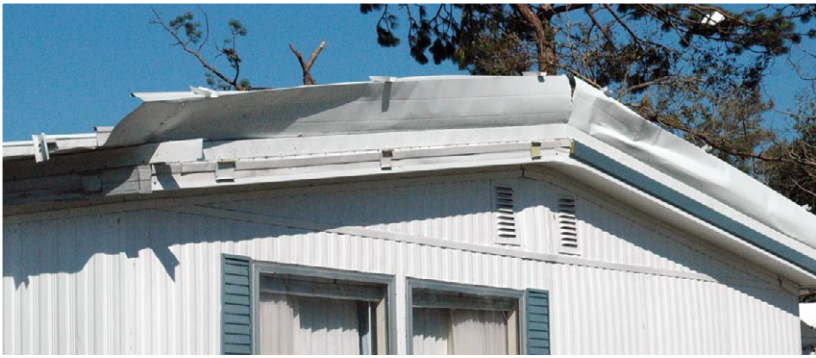
These photos shows the failure of a “reroof.” Uplift forces at the edges of the roof caused portions of the added roof to lift and peel off the manufactured home.
