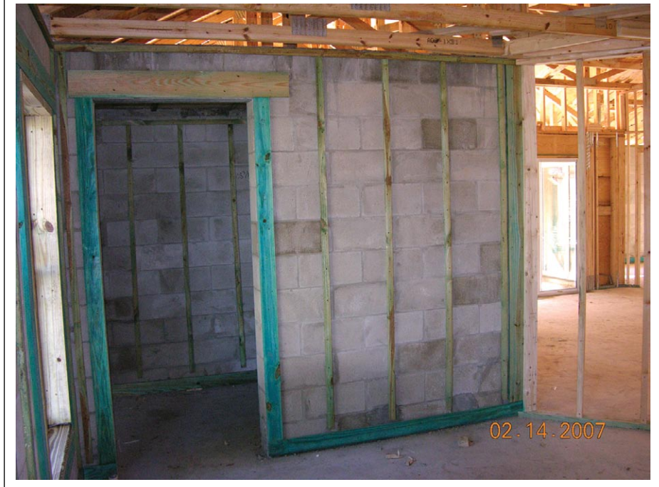
View of an in-residence shelter under construction. Steel reinforced and fully grouted CMU surround the shelter space (New Smyrna Beach, FL).
