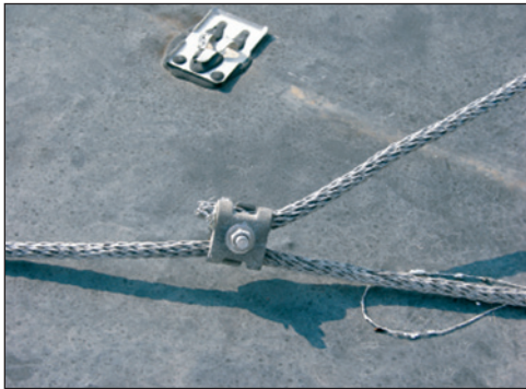
Figure 8. To avoid free ends of connectors being whipped around by wind, bolted splice connectors are recommended because they provide a more reliable connection.
