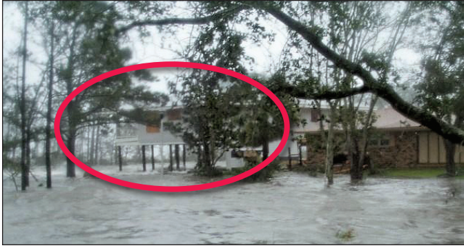
Figure 13. Pass Christian, Mississippi, home elevated on reinforced concrete columns in Zone A, with the bottom of the floor beam elevated approximately 9 feet above the BFE. Although Katrina flooding was approximately 4 feet above the top of the lowest elevated floor, the home sustained no structural damage. All other buildings in the vicinity were destroyed.
