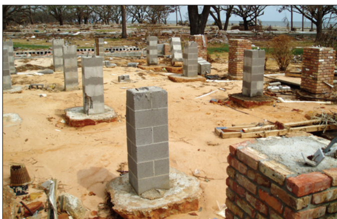
Figure 5. Hurricane Katrina damage to buildings in coastal Mississippi. The upper left, upper right, and lower left photos are of buildings that were close to the Gulf shoreline and subjected to storm surge above the floor and large waves striking the building walls. The lower right photo is of a building almost 1 mile from the Gulf, and subjected to storm surge flooding only.
