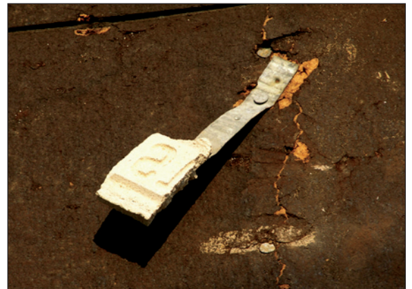
Figure 5. This tie was embedded in the mortar, but the bond was poor.
