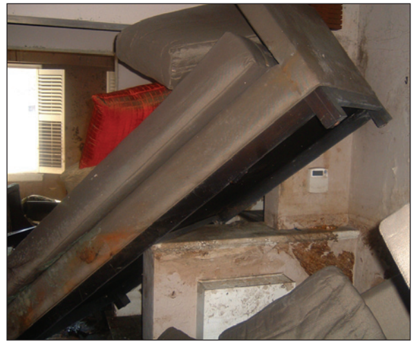
Figure 2. Furniture stacked by flood waters creates a safety hazard.
