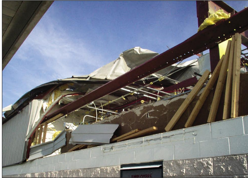
Figure 6-2. Failure of wood stud wall supporting wall panels above masonry wall (Charlotte County EOC)
