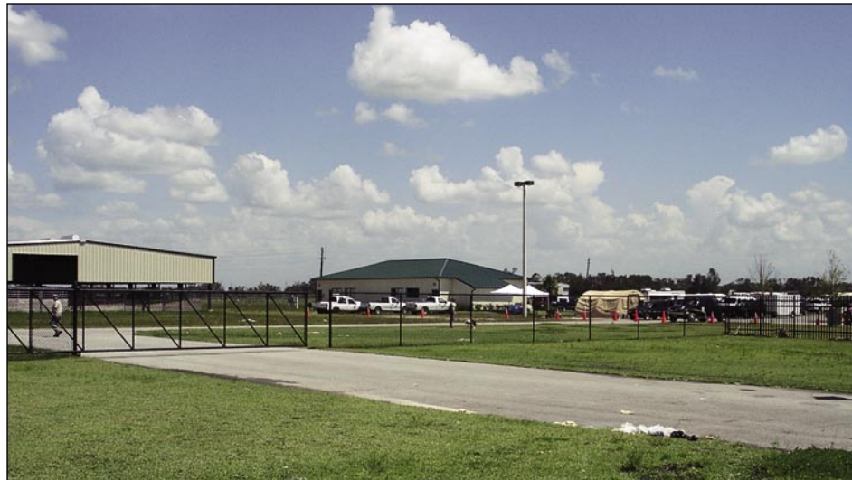
Figure 6-20. Pre-engineered metal buildings with minimal damage located near the Turner Agri-Civic Center (Arcadia)
