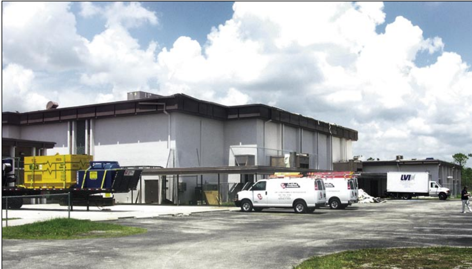
Figure 6-21. Exterior view of Port Charlotte Middle School showing both gymnasium area (tall section) and typical classroom (lower section, rear of photo)
