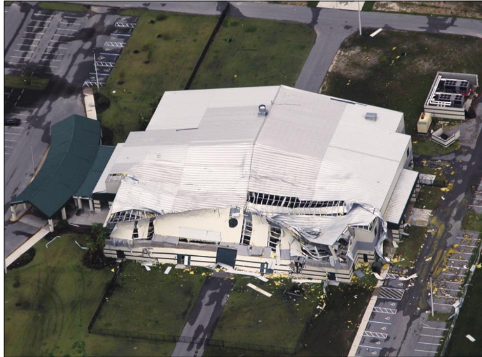
Figure 6-17. Aerial view of Turner Agri-Civic Center damage caused by Hurricane Charley (Arcadia)
