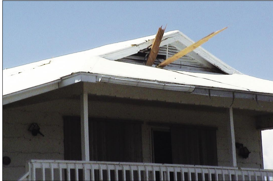
Figure 3-37. Impact of structural wood members in the gable end from a neighboring house (Pine Island)
