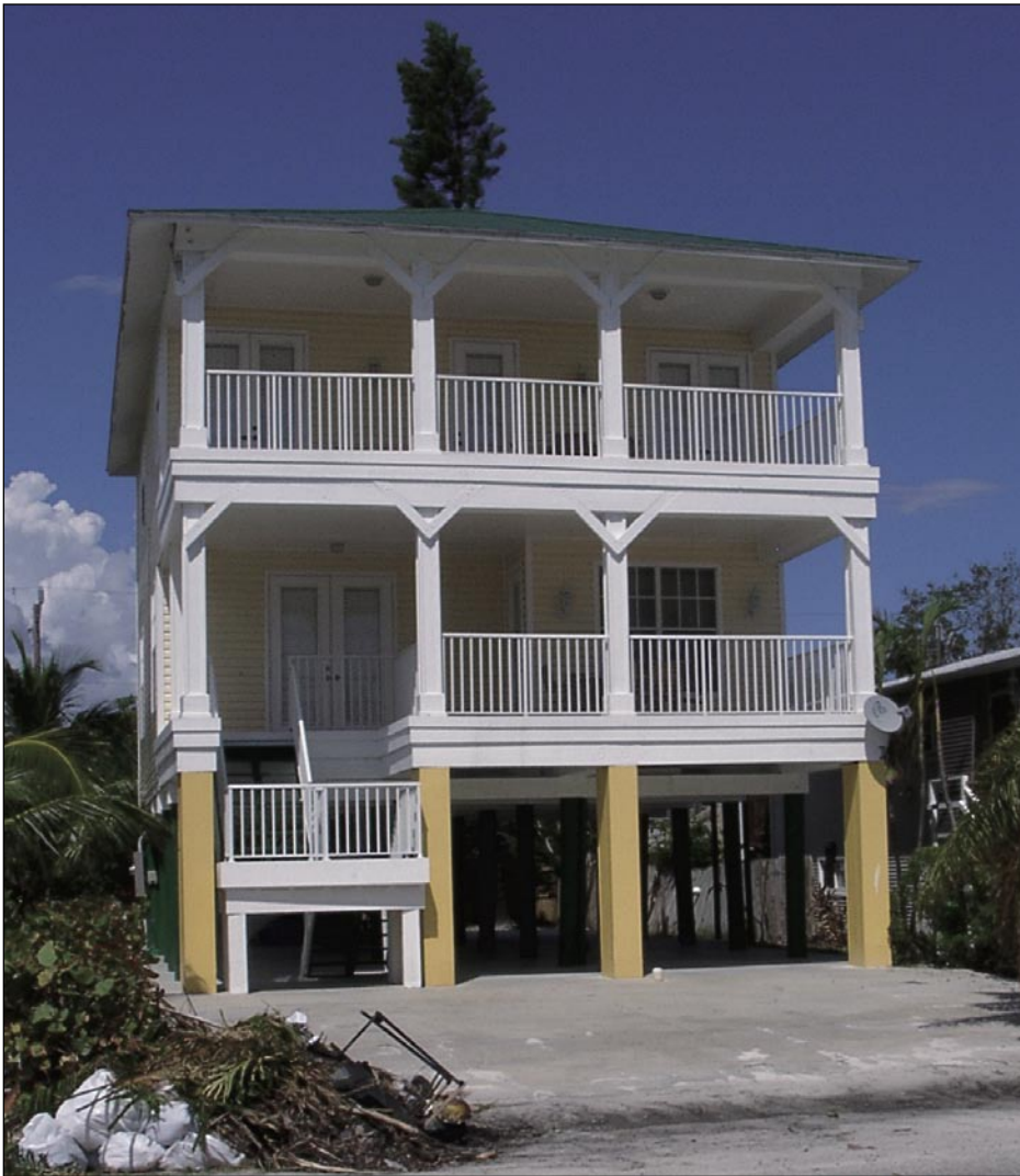
Figure 3-53. Newly constructed house elevated on piles sustained no storm surge damage (Fort Myers Beach)
