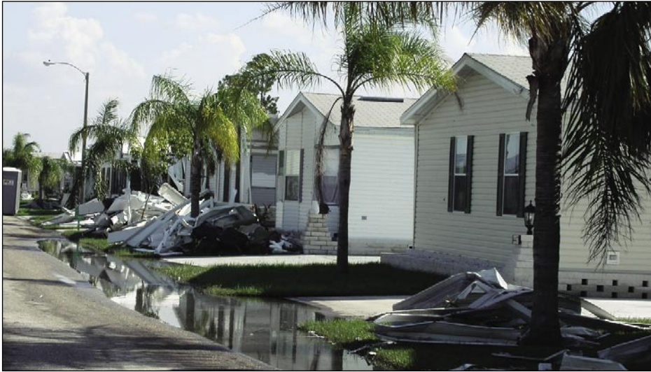
Figure 3-39. Typical metal roof panel and siding debris from failed accessory structures and manufactured homes that were stripped of siding resulting from accessory structures failure (Arcadia)
