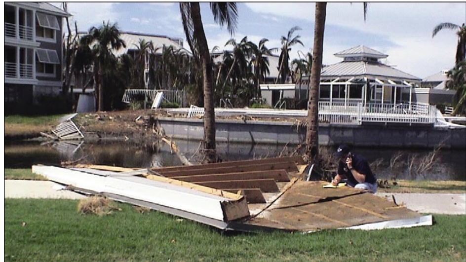
Figure 3-38. Large section of roof structure transported over 200 yards from its source (Captiva Island)
