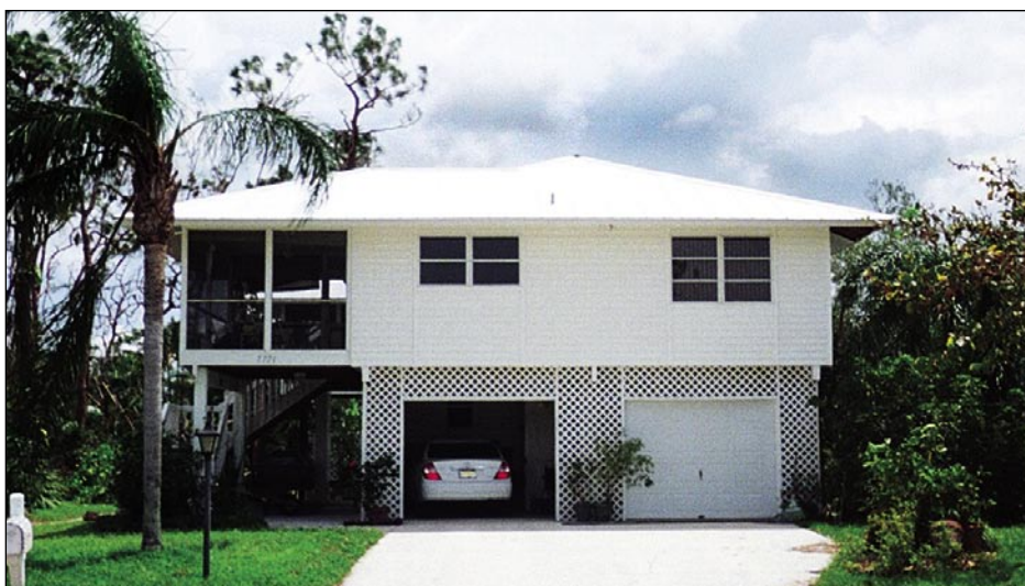
Figure 3-17. Typical pile-elevated residence with undamaged metal panel roof (coastal flood zone on Pine Island)
