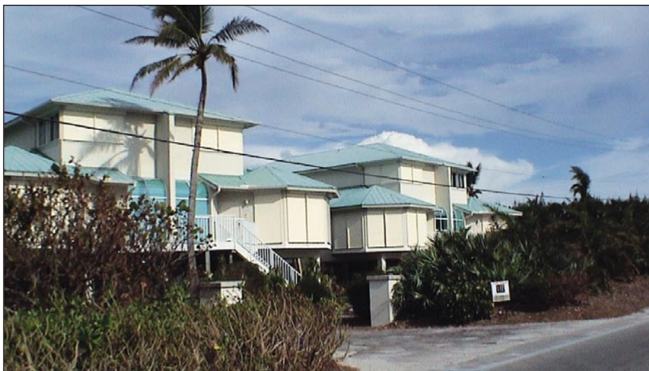
Figure 3-30. Newer house with storm shutters (Sanibel Island)
