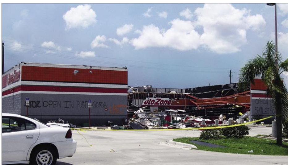
Figure 3-11. Damage to a pre-2001 FBC masonry building with steel joist roof framing and metal deck (Port Charlotte)
