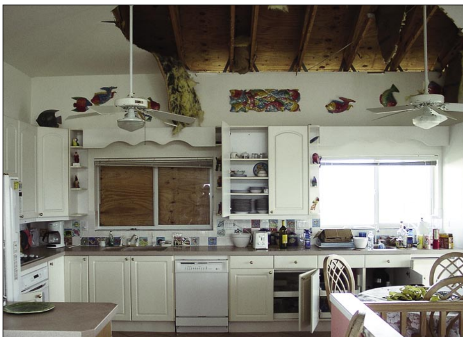
Figure 3-22. The drywall ceiling in the home shown in Figure 3-21 collapsed after becoming waterlogged and weakened by wind-driven rain that entered through the exterior soffit space. Plywood covers the opening of a window broken by windborne debris after the plastic shutters blew off (North Captiva Island).
