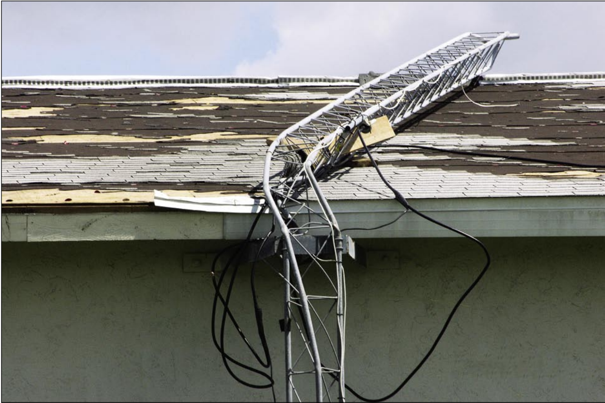
Figure 3-44. Fallen communications tower (Aqui Esta, east of Punta Gorda Isles)
