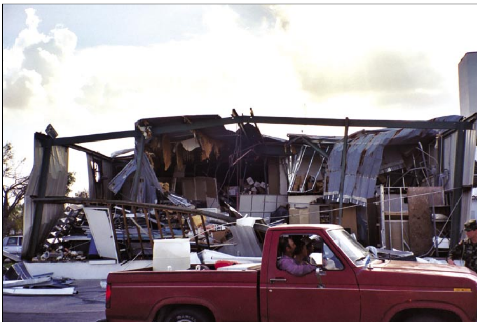
Figure 4-17. Completely destroyed pre-engineered metal building (Arcadia)
