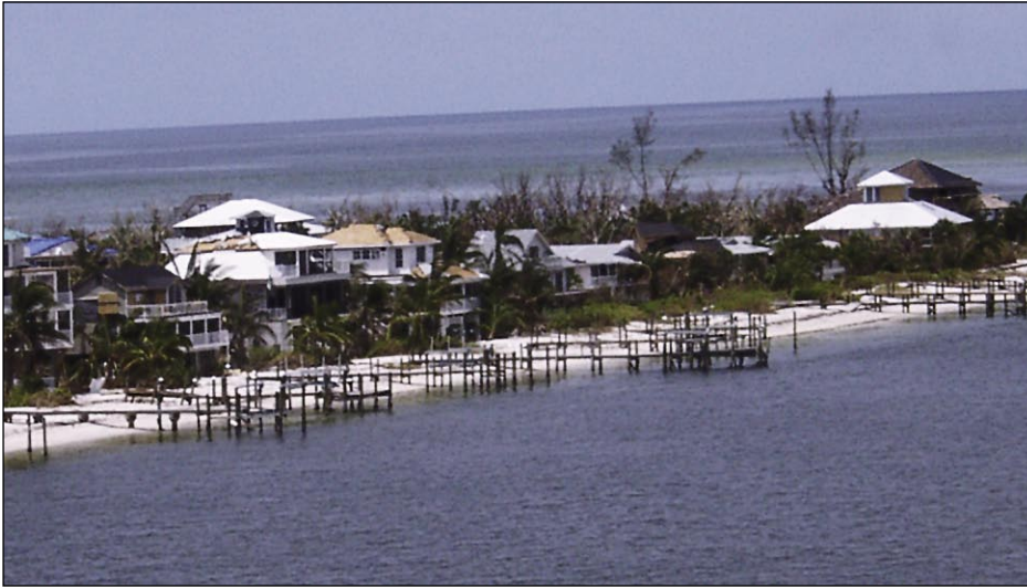
Figure 4-2. Newer single-family wood-frame residences that demonstrated good structural performance (North Captiva Island)
