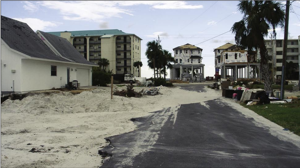
Figure 3-55. Storm surge caused scouring of the road and damage to the infrastructure (i.e., water main) (Fort Myers Beach)
