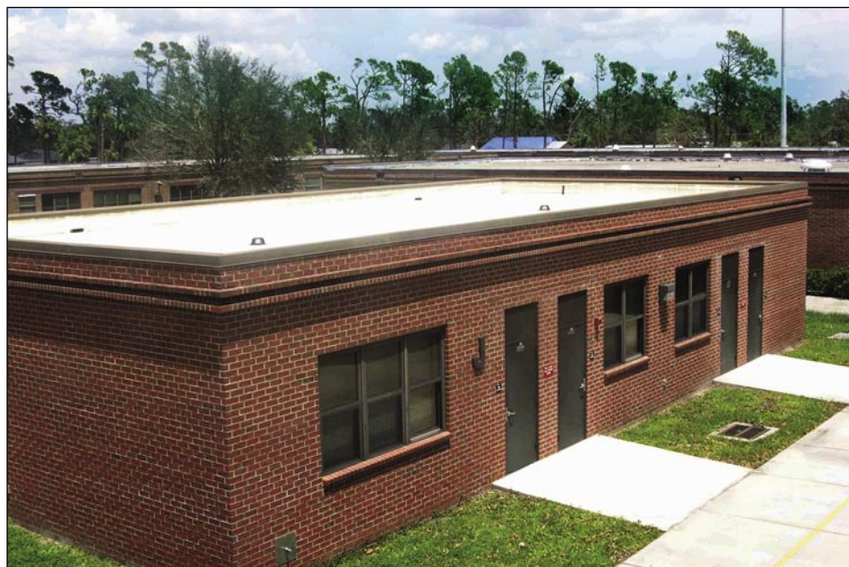
Figure 6-23. Exterior view of Liberty Elementary (Port Charlotte)
