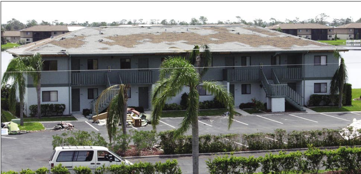
Figure 5-28. Re-covered apartment building (the newer shingles are grey and the older shingles are brown) (Deep Creek).
