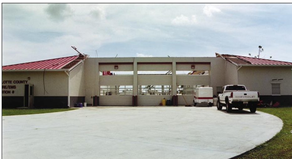
Figure 6-4. Overview of west side of Port Charlotte Fire Station No. 12
