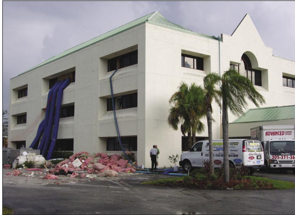
Figure 5-52. Medical office building (Port Charlotte).
