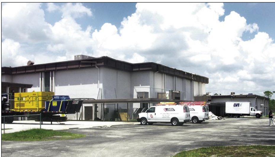
Figure 6-21. Exterior view of Port Charlotte Middle School showing both gymnasium area (tall section) and typical classroom (lower section, rear of photo)
