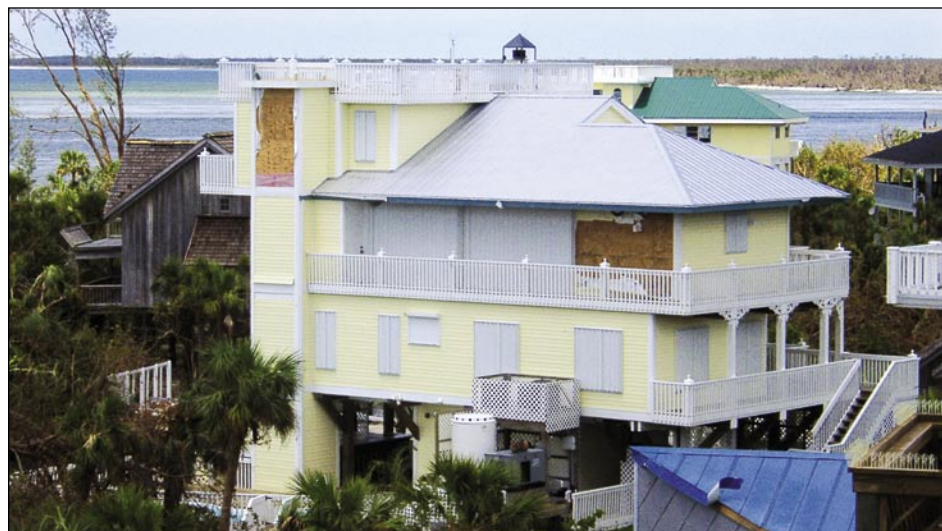
Figure 4-1. No structural damage was observed to new buildings built to the 2001 FBC standards (North Captiva Island).
