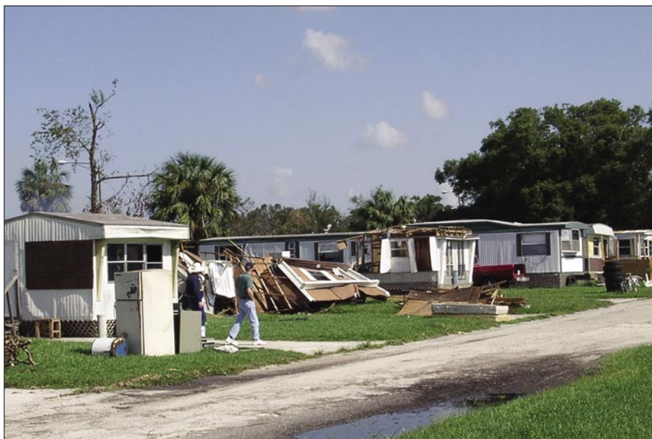
Figure 4-9. Pre-1976 HUD manufactured home sustained substantial damage (Bowling Green)
