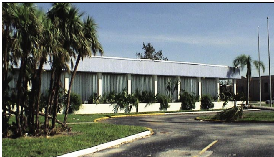
Figure 7-4. Exterior view of the galvanized shutters that protected the Charlotte County South Annex (Punta Gorda)
