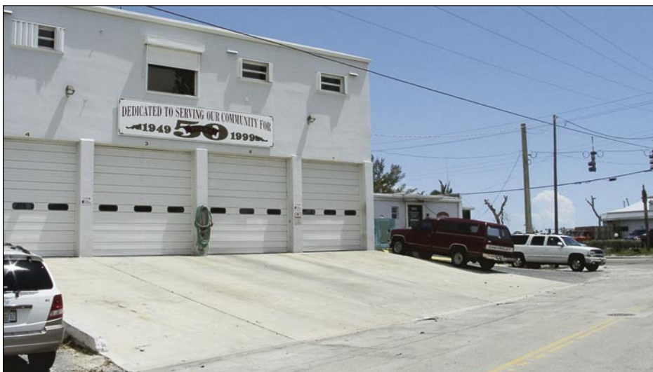
Figure 3-54. Fire station elevated on fill prevented any storm surge damage (Fort Myers Beach)
