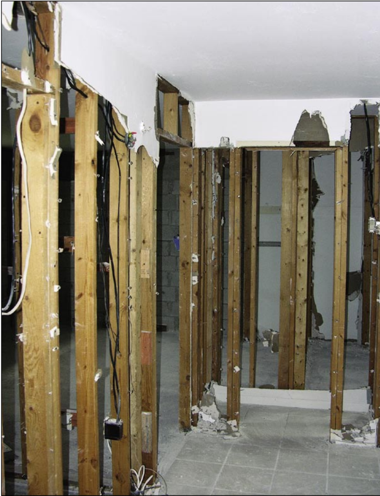
Figure 5-21. After the attic vent failed, water entered this residence. Wet carpeting and a substantial amount of wet gypsum board had to be removed (Punta Gorda Isles).
