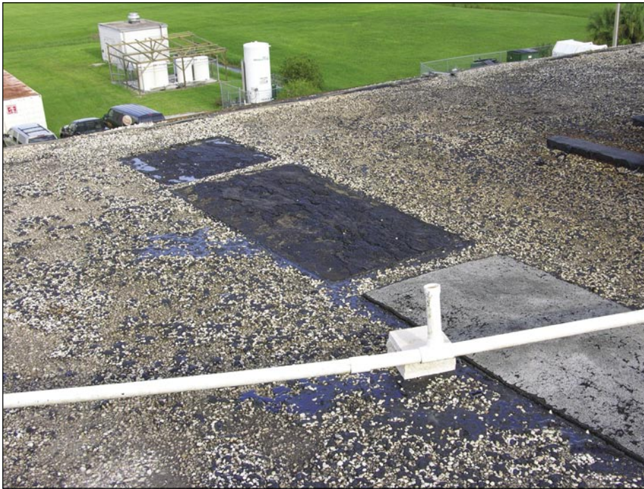
Figure 5-60. This view of the back side of the upper roof of a hospital (see Figure 6-8) shows that the missing gutter and asphalt plank walkway pad were blown away (Arcadia).
