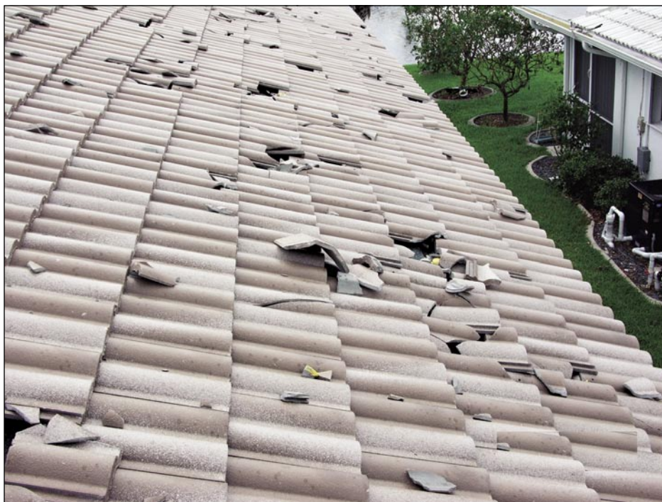
Figure 5-49. A view of the roof on the back side of the residence shown in Figure 5-41. Tiles (including a hip tile) from the front garage roof landed in this area and broke several field tiles (Deep Creek).
