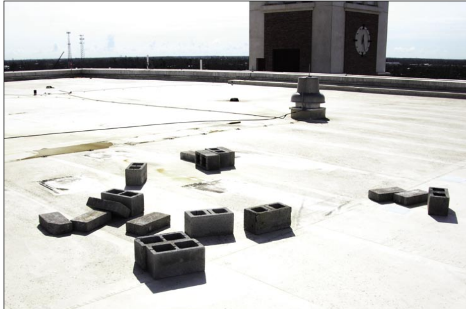
Figure 5-80. A satellite dish previously sat in this location. It was held down only with CMU and blew off the five-story building (Punta Gorda).
