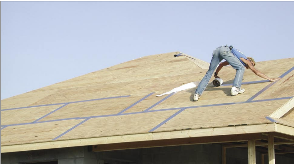
Figure 5-23. Installation of self-adhering modified bitumen tape at sheathing joints, as part of an enhanced underlayment system on a Fortified...for safer living™ house under construction (IBHS)
