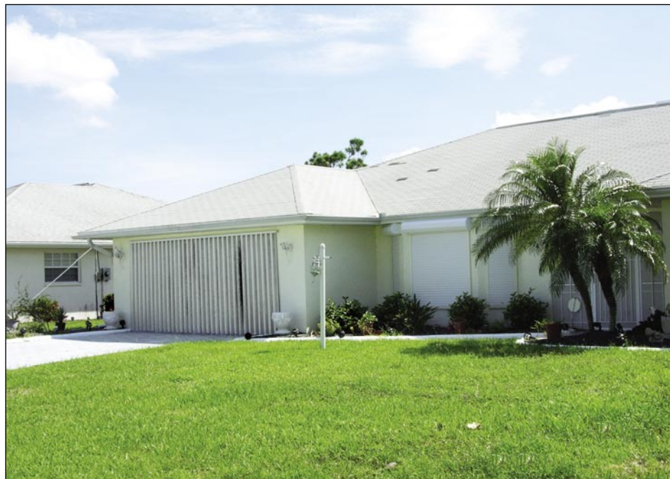
Figure 5-13. This house, which appeared undamaged from windborne debris, had roll-up shutters at the windows and metal panel shutters at the garage (Deep Creek).
