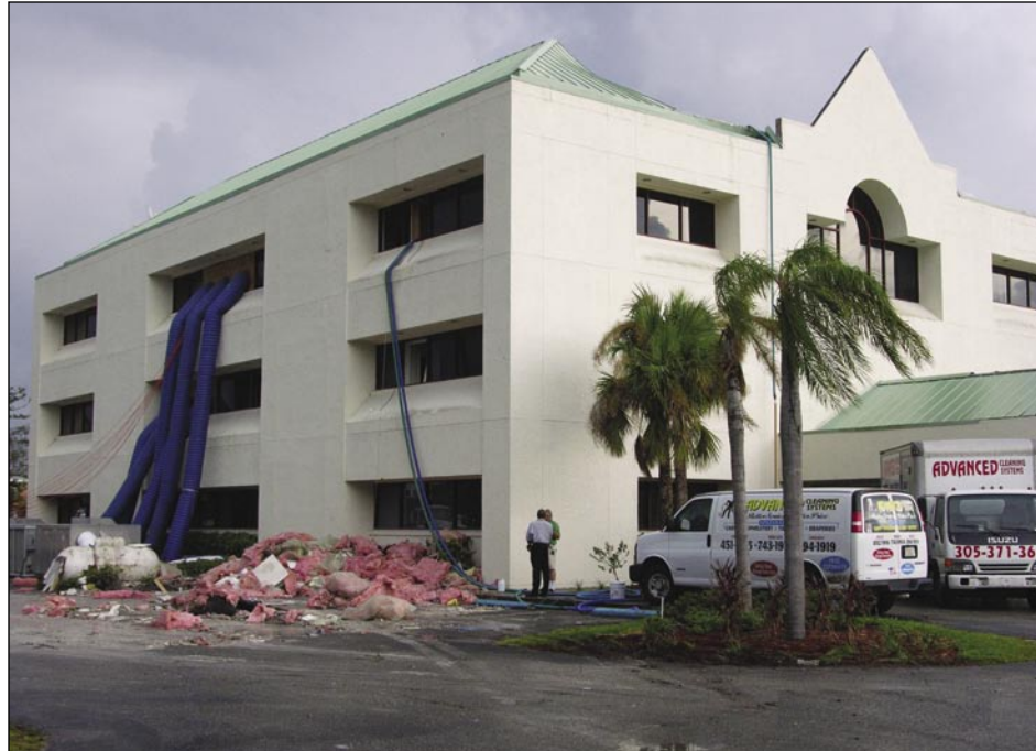
Figure 5-52. Medical office building (Port Charlotte).
