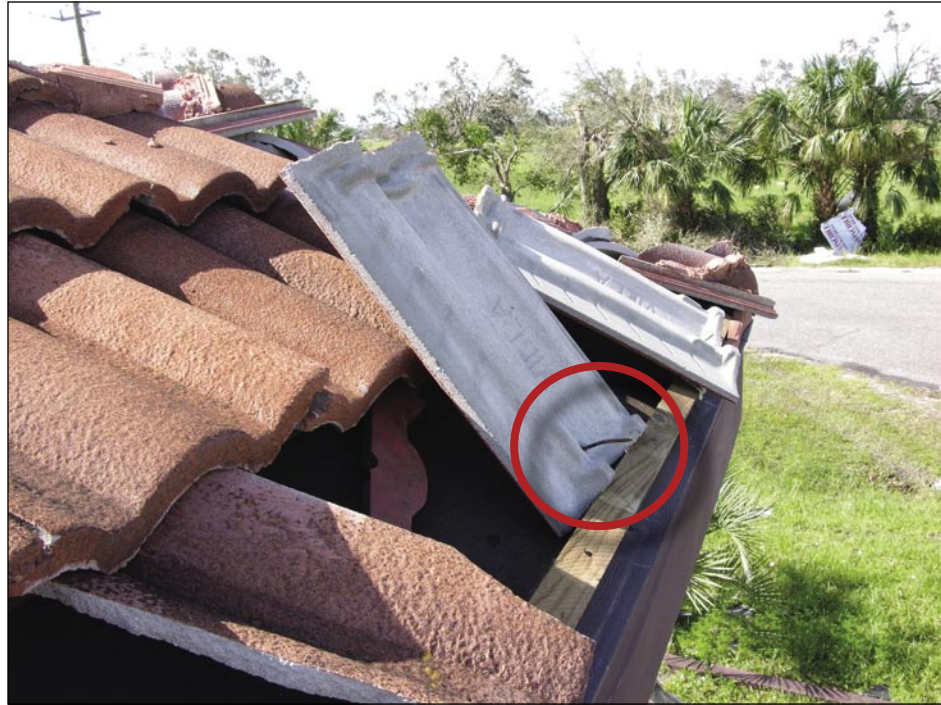
Figure 5-34. Each tile on this building was attached to battens with a single 3 1 / 8 -inch long smooth shank nail (Arcadia)
