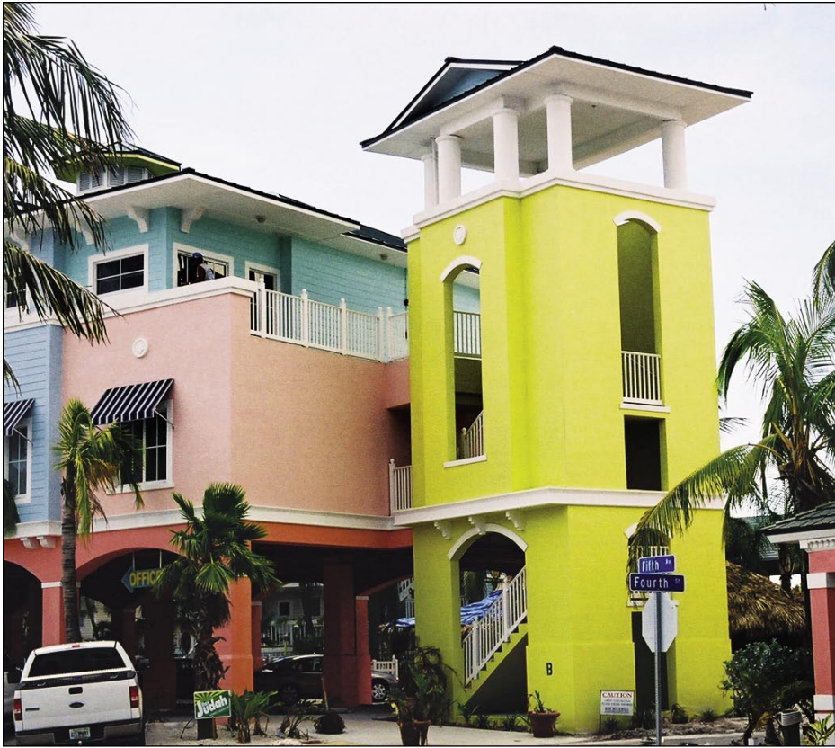
Figure 7-3. Exterior view of the elevated Lighthouse Resort Inn and Suites, which remained dry and undamaged after Hurricane Charley (Fort Myers Beach)
