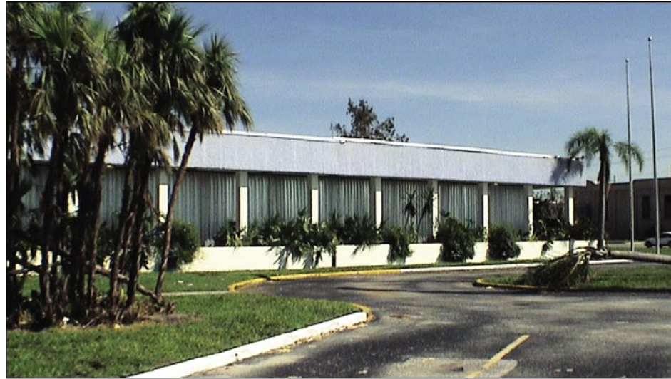
Figure 7-4. Exterior view of the galvanized shutters that protected the Charlotte County South Annex (Punta Gorda)
