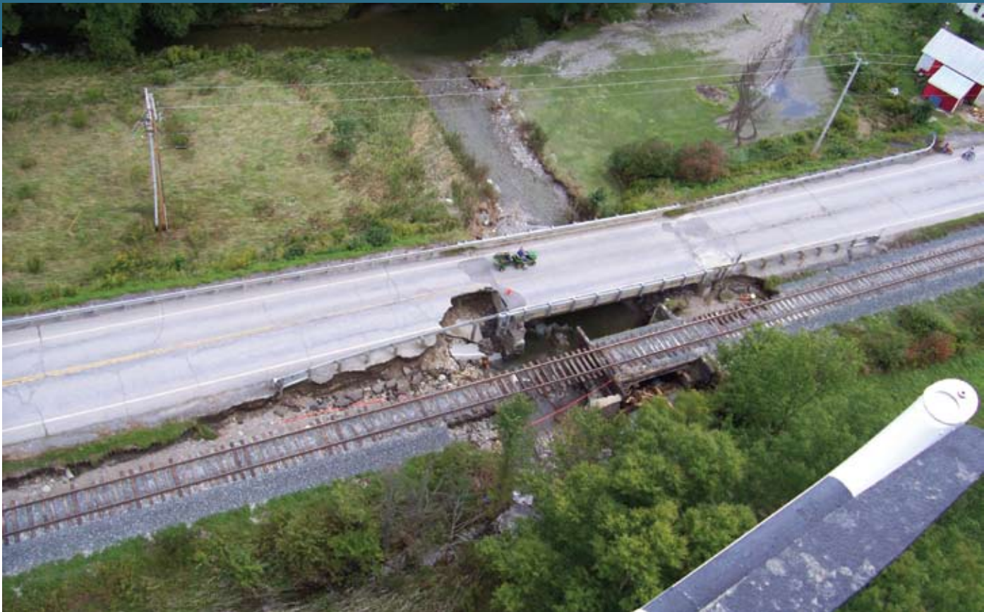
Photo courtesy of VTrans
