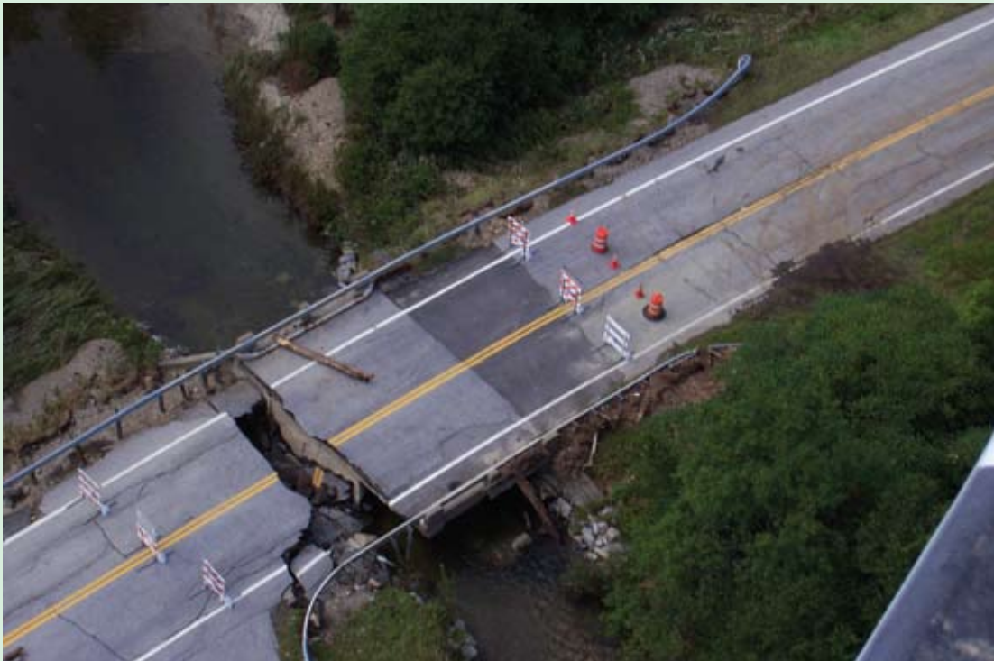
Photo courtesy of VTrans
