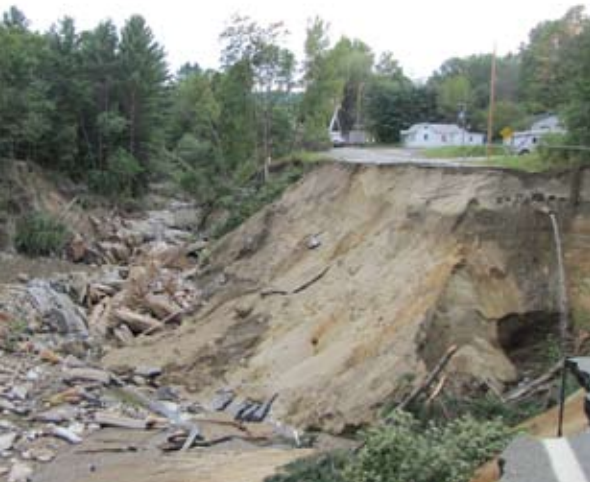
Photos courtesy of Southern Windsor County RPC
