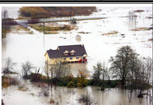
This Washington home is one of many built to NFIP standards that were not demolished by the 2007 Chehalis River flood.
