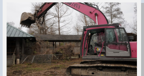
Audubon Nature Center Demolition
