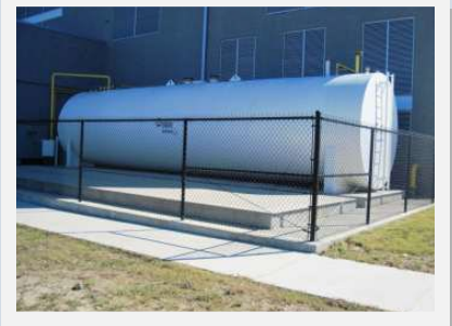
Women’s Hospital Fuel Tank
