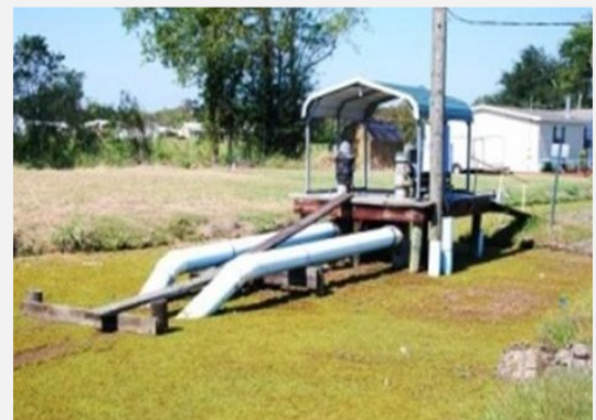
Assumption Parish Pumping Station
