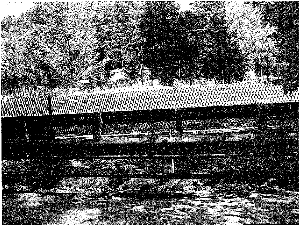
Photo 2. Overview of storm drain alignment from the EBMUD-Orinda water treatment plant looking towards the southeast onto Camino Pablo
