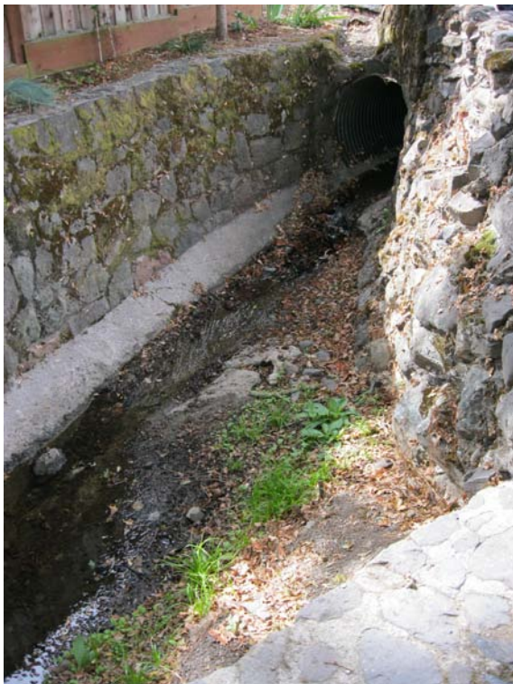
Orinda Stormwater Stytem – Drain pipe and original stone walls DPR 523L (1/95)
