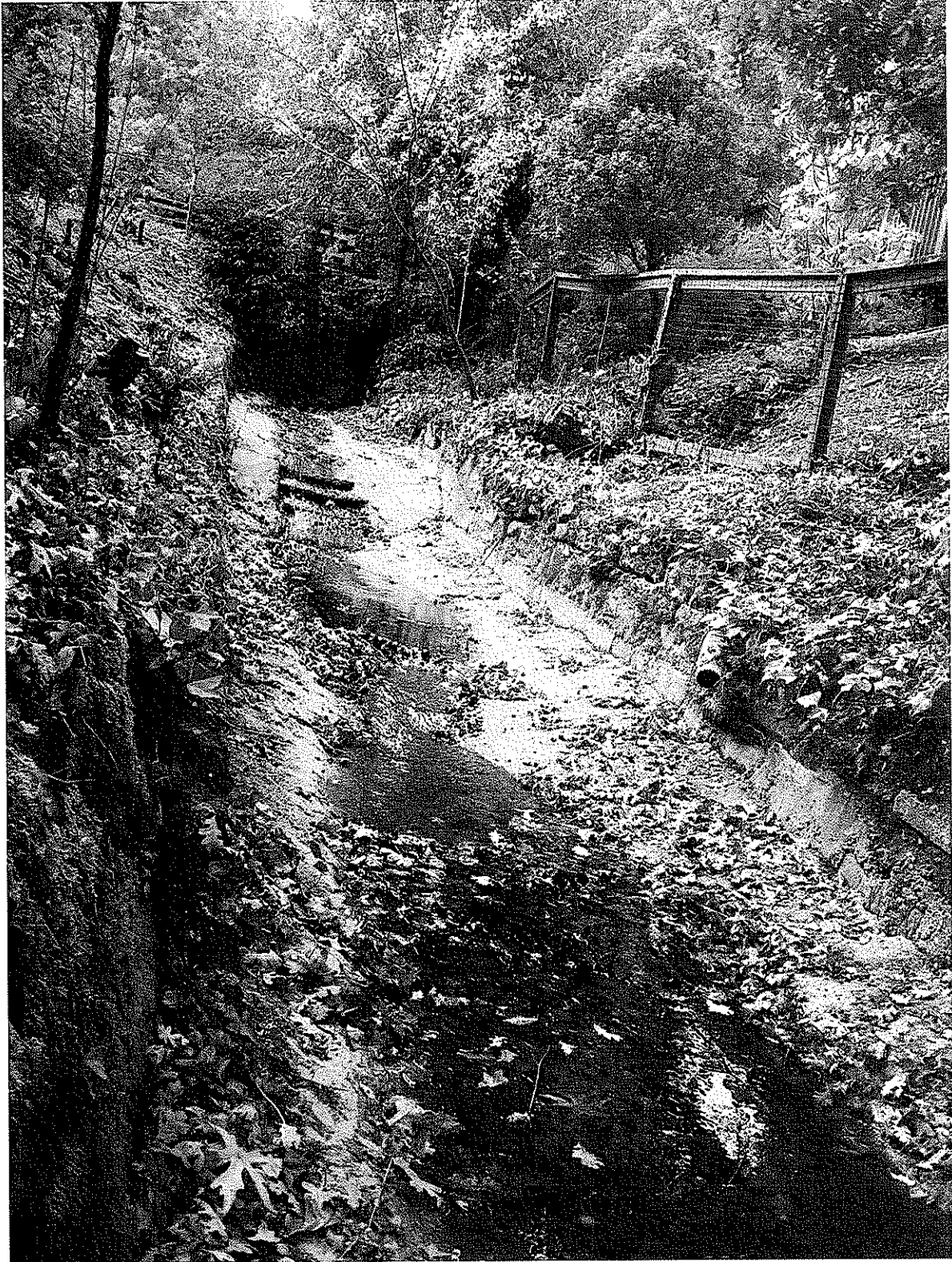
Photo 5. Overview of existing storm drain on North Lane
