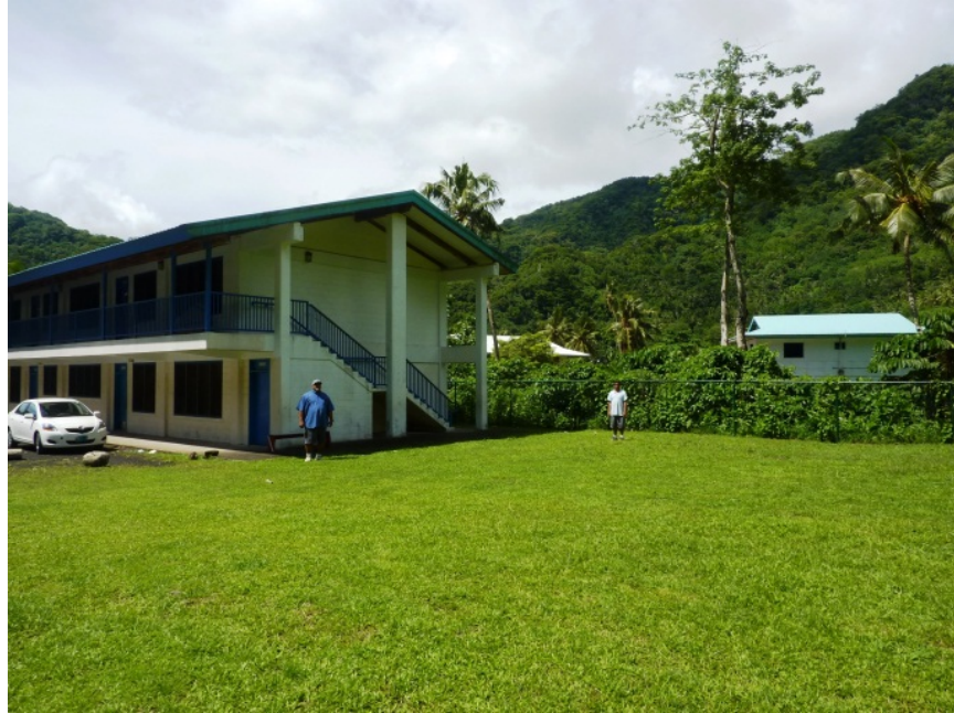
Image 4: View facing east to the proposed building site adjacent to the existing two-story classroom building. Men in photo are standing at the approximate location of the eastern corners of proposed building 400 feet from the shoreline.
