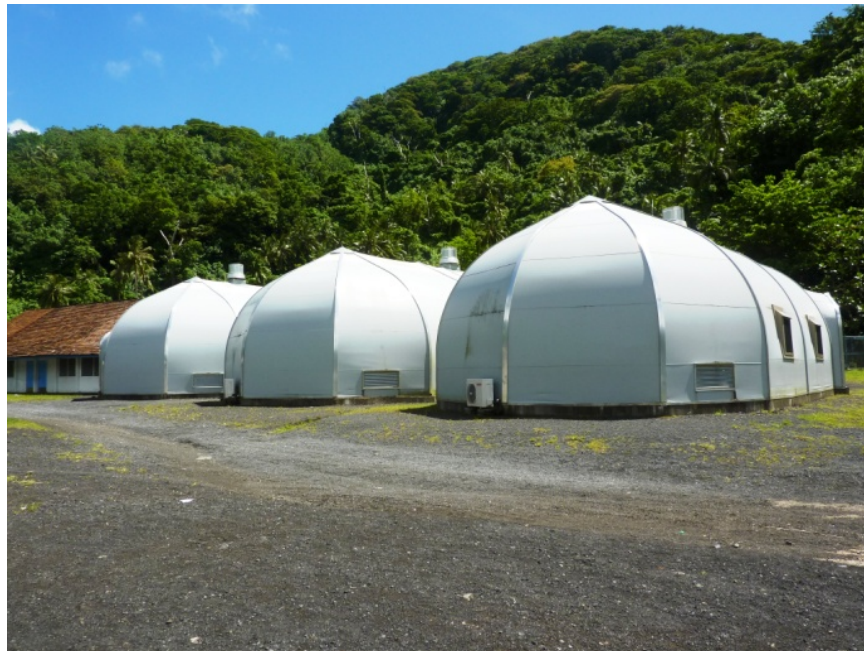
Image 3: Temporary structures were erected after the disaster to restore partial capacity.
