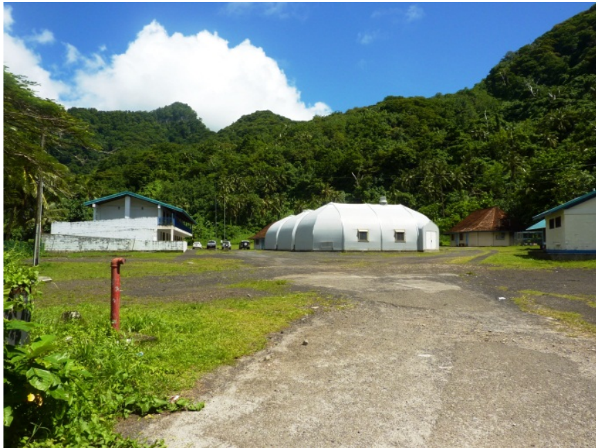
Image 2: View facing southwest shows the sites of the demolished structures in the foreground at left and right.
