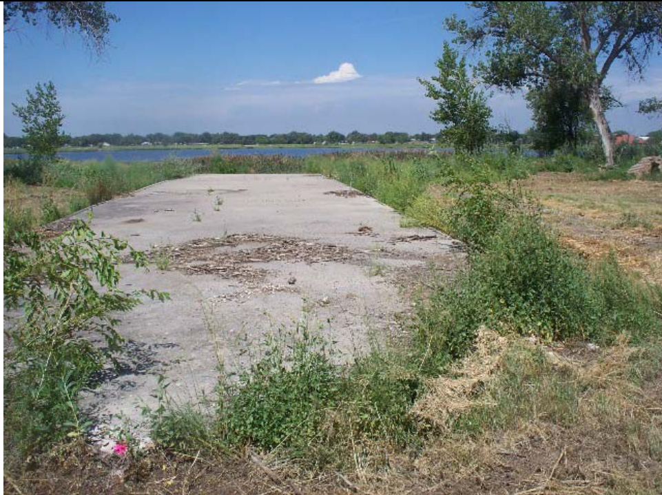
11. BOATHOUSE FOUNDATION (OUTSIDE OF PROPERTY DEVELOPMENT AREA)
