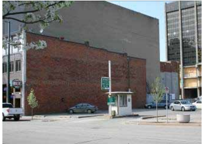
Photograph #2: View across 2 nd Avenue showing existing entrance of Lot 24/26.
