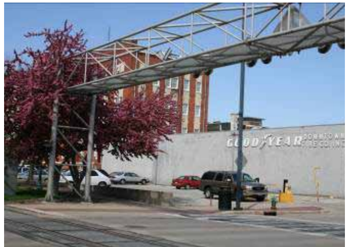
Photograph #4: View from intersection of 2 nd Avenue and Cedar River Corridor Trail of railroad adjacent to the Trail, northeast of the proposed project site.
