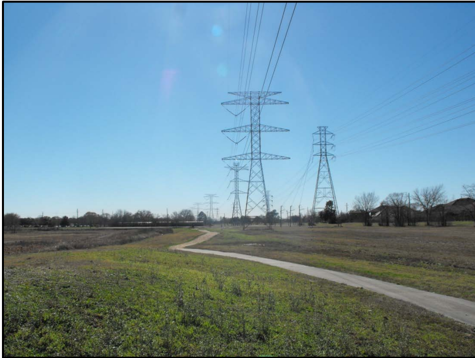
Facing south, this is a view of western portion of the project site. An electrical transmission easement is visible to the west of the site. The on-site detention basin is visible to the east.
