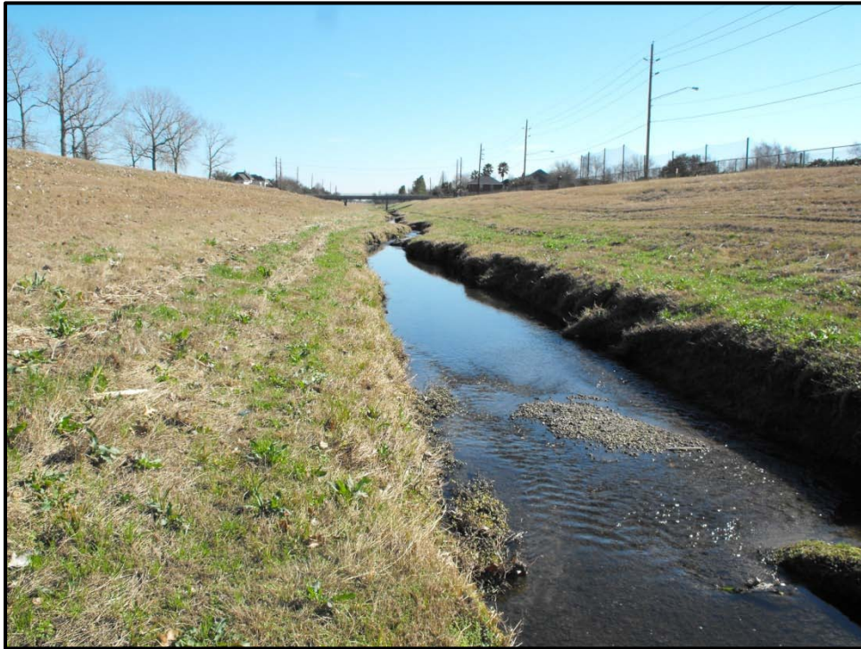
Facing east, this is a view of HCFCD E135-00-00 that is offsite and runs along the southern property boundary of the project site. The Rio Grande Drive Bridge over the drainage is visible in the distance.
