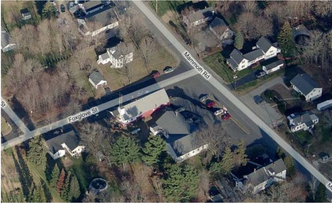
Photo 3. Bird's eye view of the existing North Fire Station (red building) looking toward the north. The station is in a residential area. The former Grange Hall (now used as a senior center) is located directly beside the station.
