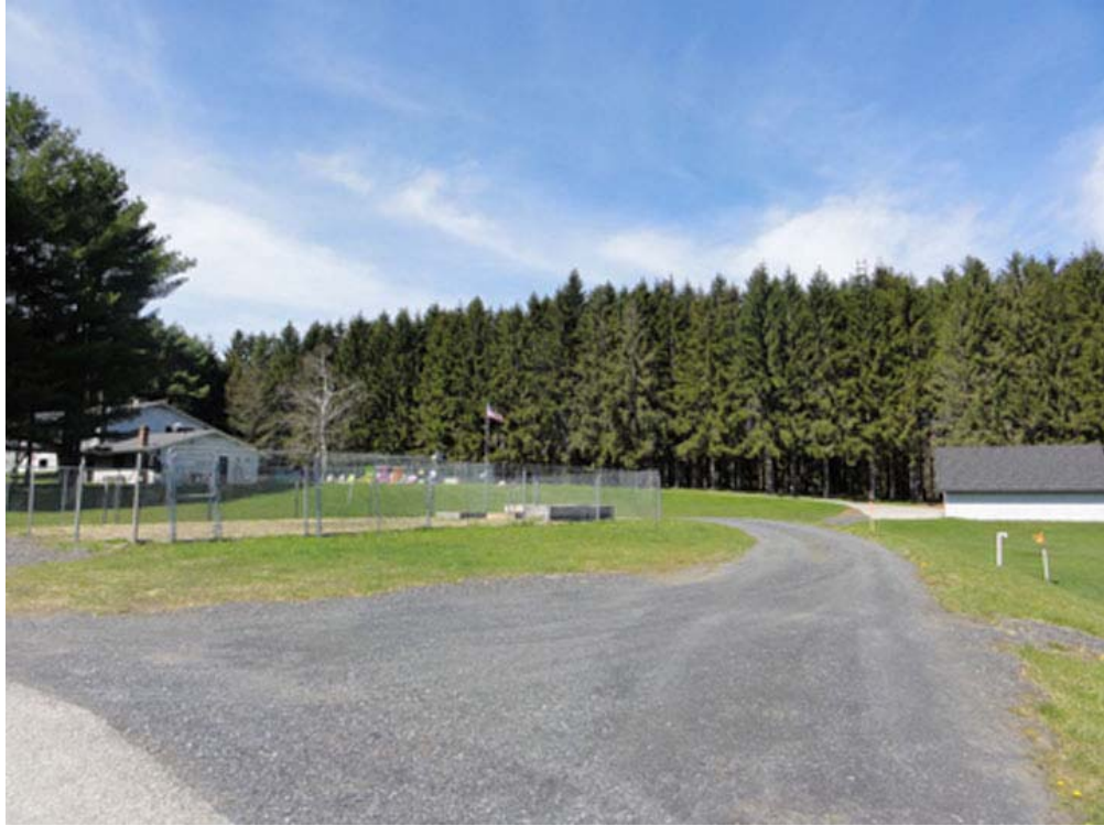
VELCO right-of-way looking southwest
