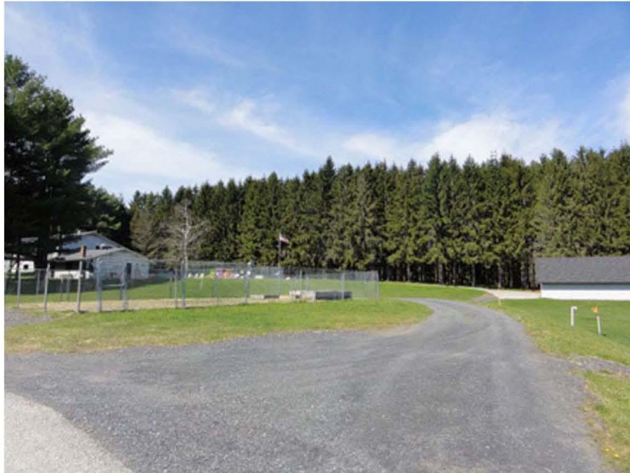
VELCO right-of-way looking southwest
