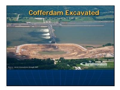
Before you can build the powerhouse, a cofferdam is constructed in the river and dewatered. In this case its size equals a football stadium 125 feet deep. Construction of the cofferdam began in May 2010. To build the "stadium", about 400,000 cubic yards of earth was excavated. The final portion of the excavation was blasting and removing weathered limestone to provide a solid foundation for the powerhouse. The total amount of time to complete the cofferdam was about 15 months.
