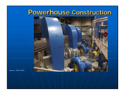
The newly constructed powerhouse downstream from the dam on Sawmill Creek housed the three new units. The old powerhouse was decommissioned, and a fourth unit was rehabbed with the recommissioning of the fish unit bypass. The fish bypass releases water to the creek to provide instream flow for salmon. The fish unit generates power from this required flow.
