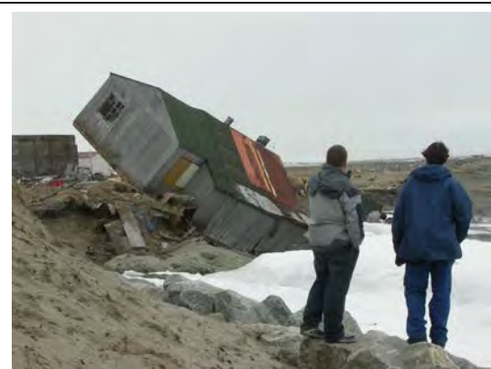
Figure 2-11. Damaged infrastructure in an Alaskan coastal community. This represents the juxtaposition of problems caused by increasing temperatures: permafrost melt destabilizing the ground combined with increased water temperature that reduces protective ice cover and allows waves to melt the base of permafrost bluffs and increase coastal erosion. Photo by Ned Rozell, Geophysical Institute/University of Alaska Fairbanks.
