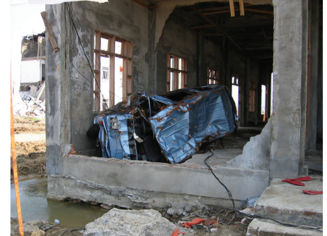
An automobile, carried by surging water during the December 26, 2005, Indian Ocean tsunami, lies crumpled in a building in Banda Aceh, Indonesia. (USGS photo/Guy Gelfenbaum)
