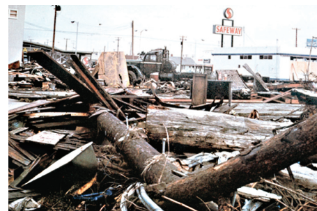
Crescent City, Calif., is heavily damaged following a tsunami generated in Alaska on March 28, 1964. (University of California-EERC photo)
