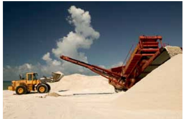
By adding sand to an eroding beach, beach nourishment can protect shorefronts against wave action and flooding.
