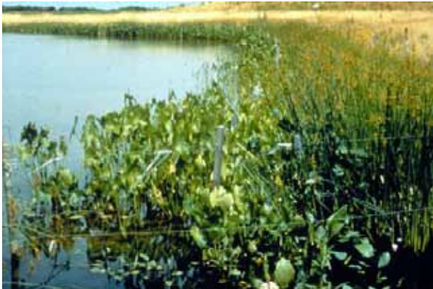
Detention basins can be designed to mimic natural ponds with gentle side slopes and native vegetation, which help prevent erosion and suspension of sediment and intercept pollutants from runoff.
