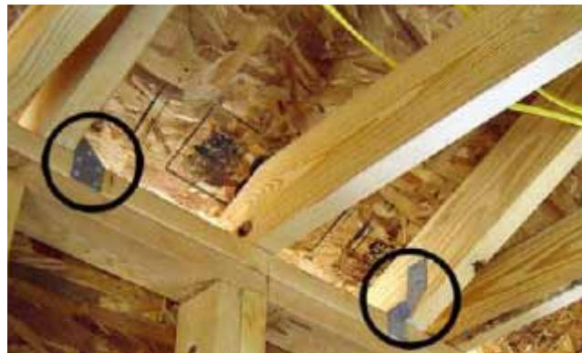
Hurricane clips help anchor roofs to their main structure to prevent detachment during severe winds.
