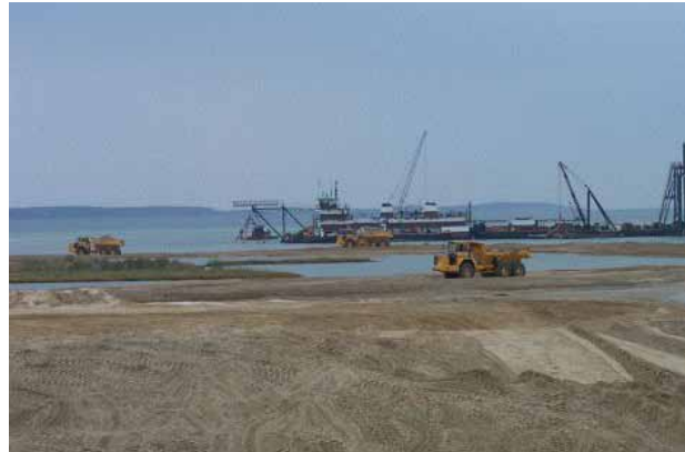
Restoration projects may entail placing and shaping sediment and planting vegetation, in addition to other activities, in order to rebuild degraded wetlands.
