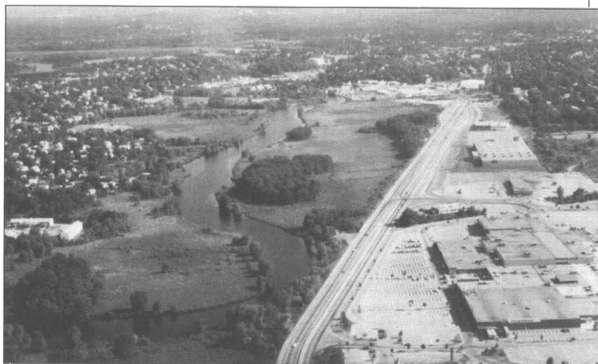
Charles River natural flood water storage area near Dedham, Massachusetts.
