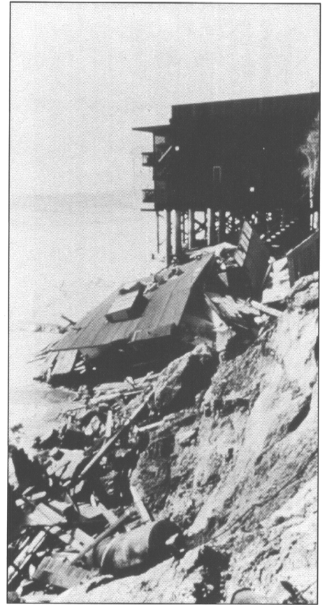
Natural coastal erosion can be greatly accelerated by wave action during storms and hurricanes. Combined with inappropriate construction in coastal areas, this natural process can result in disaster.
