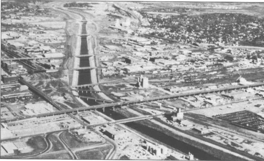
It has been estimated that 3.5 to 5.5 million acres of floodplain land had been developed for urban use by the late 1970s. In many cases, this change has resulted in greatly altered river corridors and adjacent lands. Channel modification, Sioux City, Iowa.
