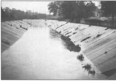
Storm drainage is a significant problem in many large urban areas, particularly if development has been rapid and not well planned. Drainage systems must be designed to handle infrequent, but potentially catastrophic, events.
