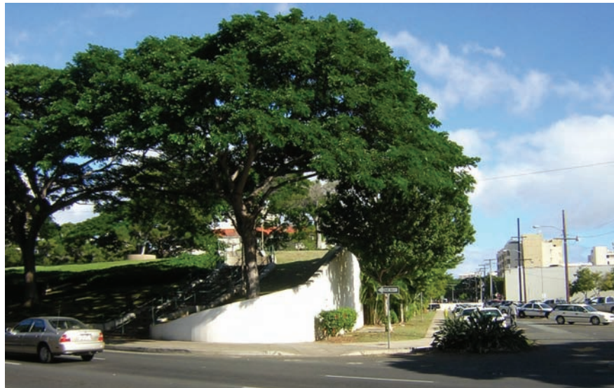
Figure 4-1 Soil berm combined with a community open space. Ocean facing walls can deflect incoming waves while sloped sides provide for quick access.
