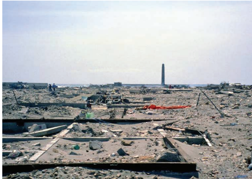
Figure 2-10 Total destruction of a group of wood-frame houses in Aonae Village, Okushiri, Island, Japan (1993 Okushiri Tsunami).
