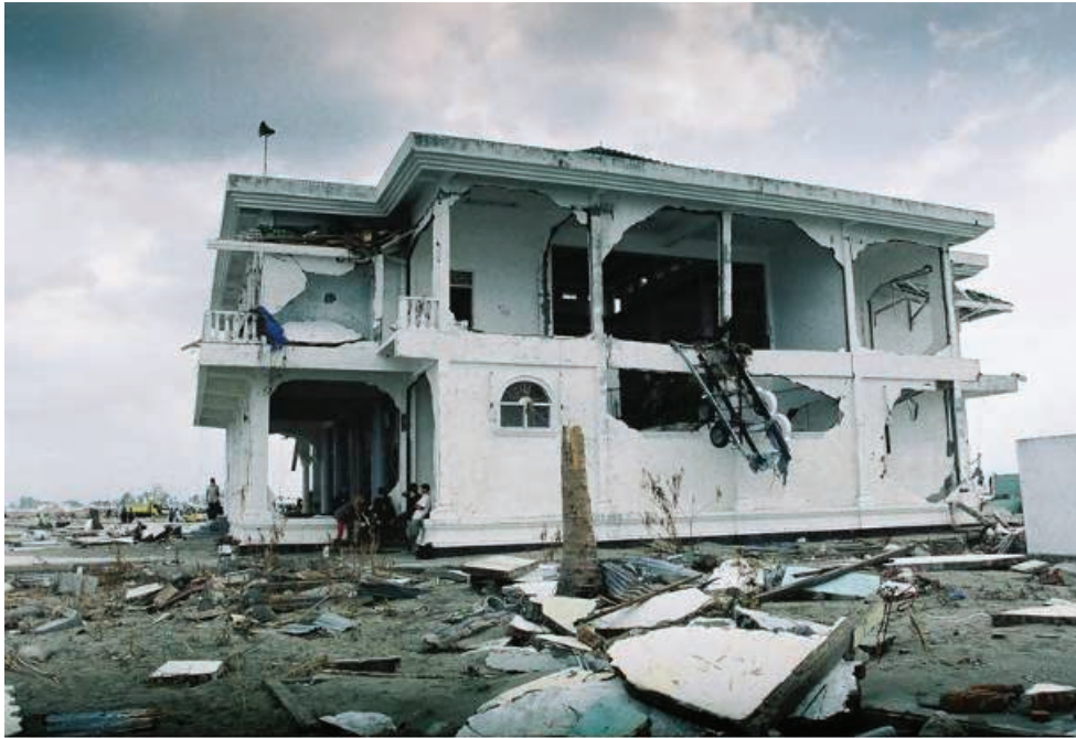
Figure 2-15 Example of surviving reinforced concrete mosque in Uleele, Banda Aceh (Photo courtesy J. Borerro)
