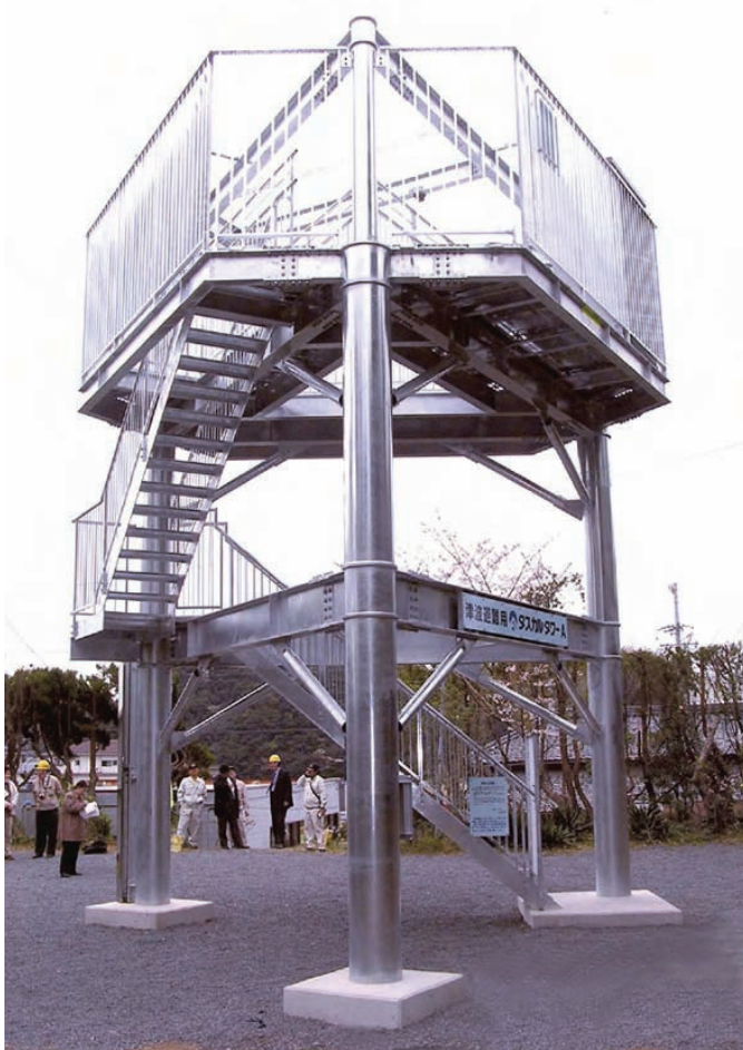
Figure A-1 Life-Saving Tower
