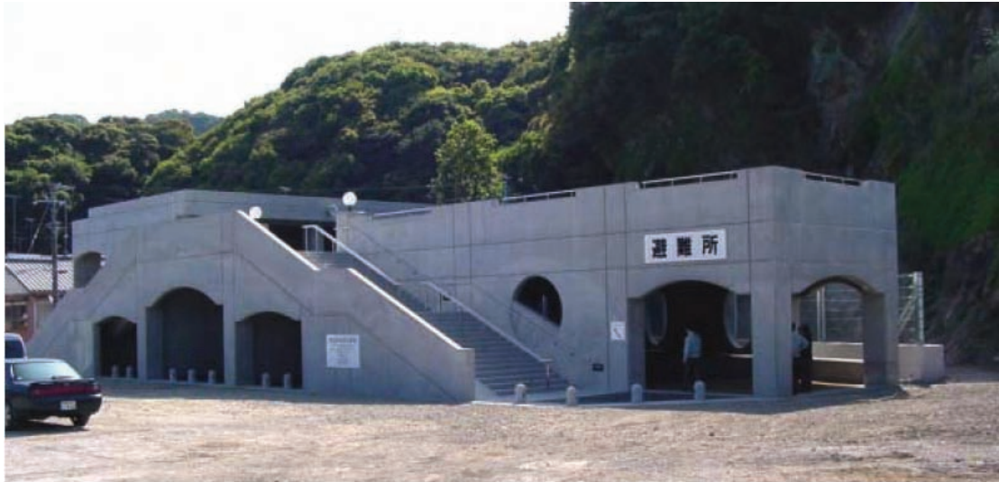
Figure A-4 Tsunami refuge in Kaifu, Japan.
