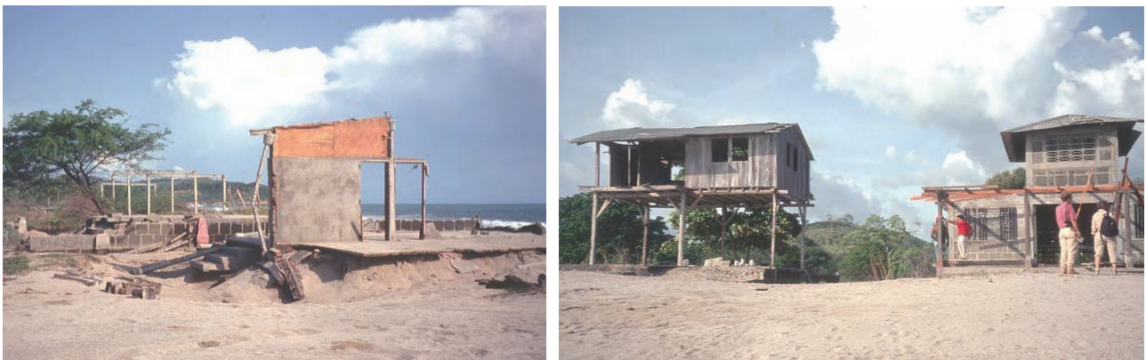
Figure 2-11 Beach houses with varying levels of damage in El Popoyo, Nicaragua (1992 Nicaragua Tsunami). All three houses are in the same vicinity.
