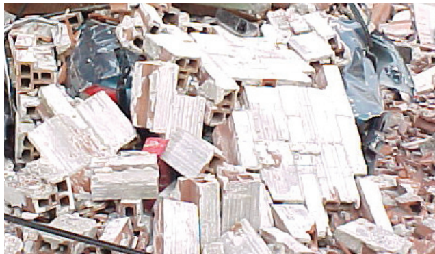
■ Figure 19. URM building damage, 2001 Nisqually, Washington earthquake.
