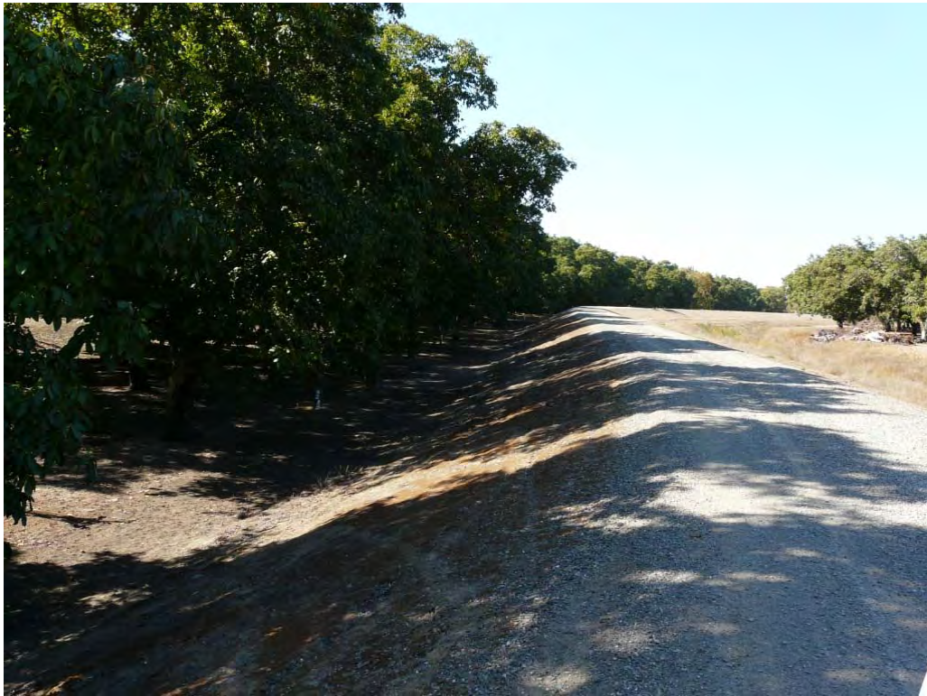
Acceptable Tree Maintenance: No limbs within 5' of the levee obstruct visibility or access
