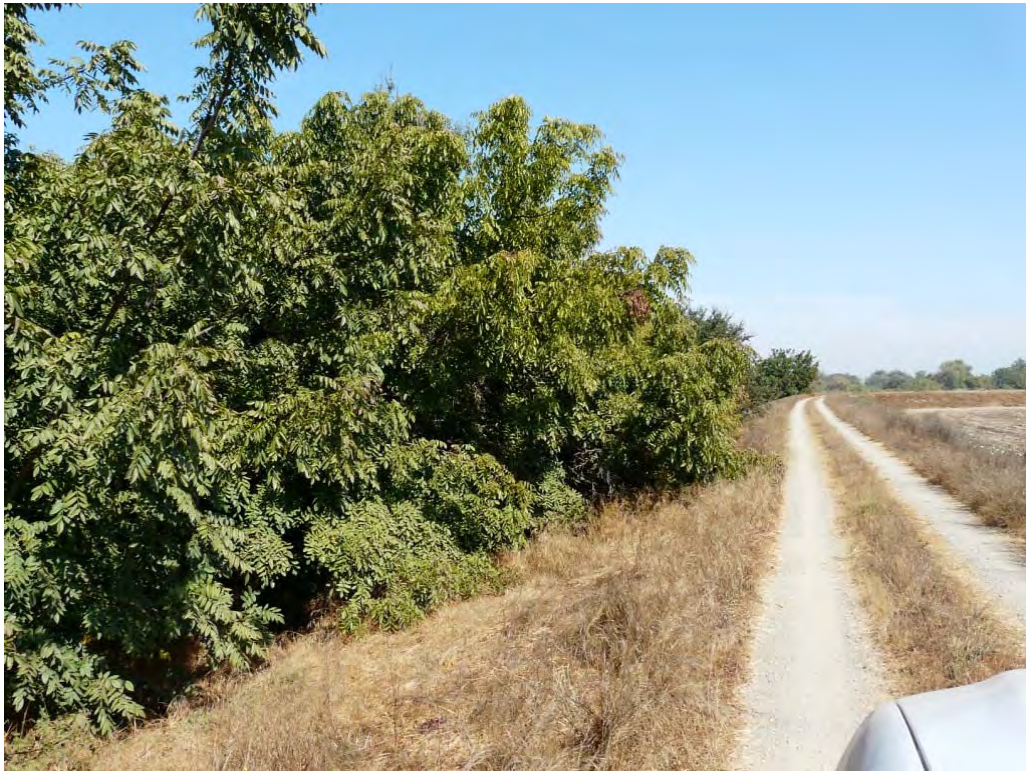
Unacceptable Tree Maintenance: Significant density of tree limbs completely obstruct visibility and access
