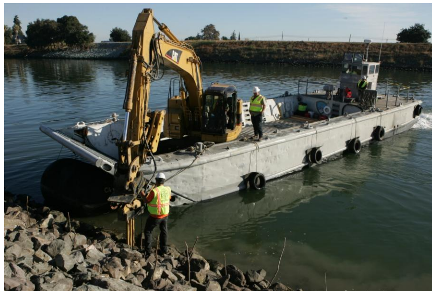
Photo 1: Stinger excavator on a barge
