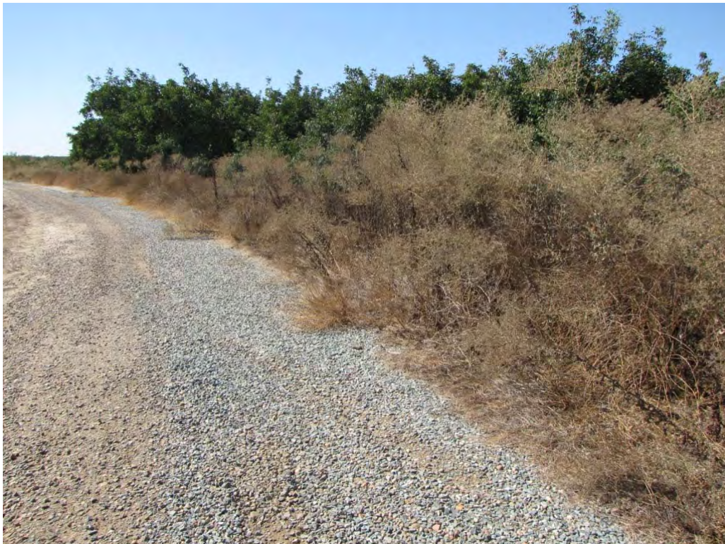
Unacceptable Maintenance: Grass or brush completely obstruct visibility and access
