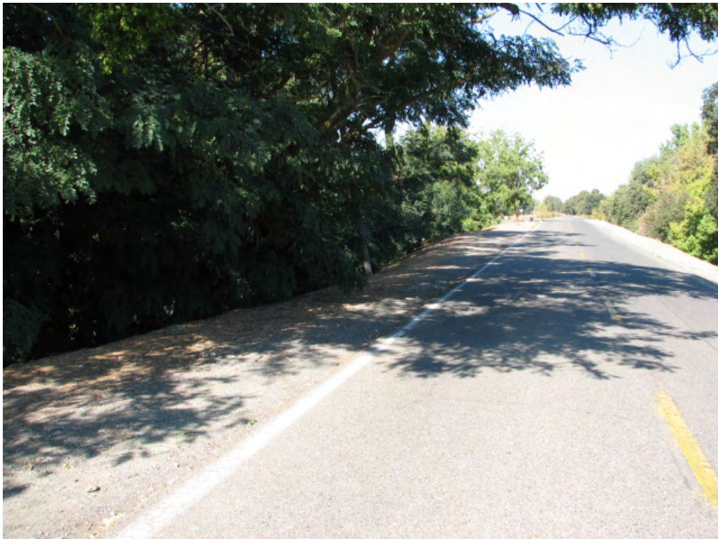
Minimally Acceptable Tree Maintenance: Moderate density of tree limbs partially obstruct visibility and access
