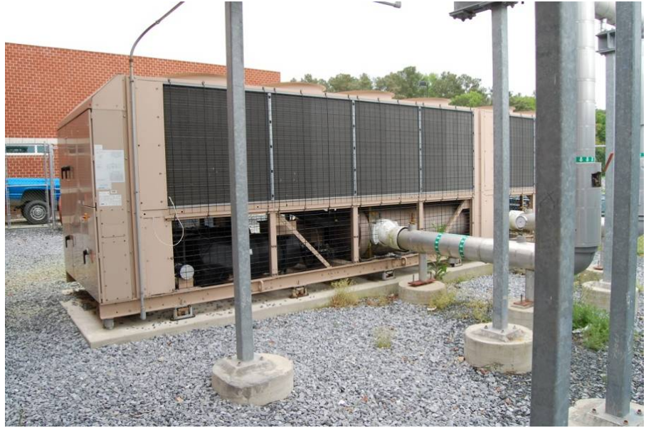
Figure 4-6 Air-cooled chiller.
