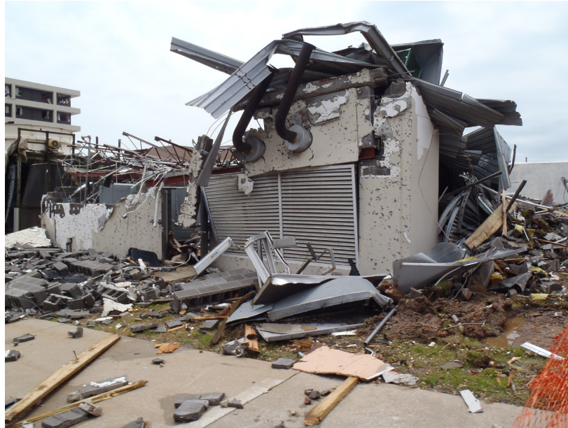
Figure 2-8 Steel deck/steel joist URM building housing the emergency generator and switchgear destroyed in the Joplin, Missouri Tornado (FEMA, 2012a).
