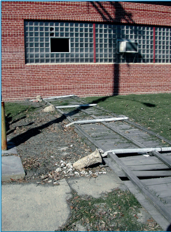
Figure 2-12: Katrina's storm surge flooding knocked down this fence adjacent to a fire station (2005).
