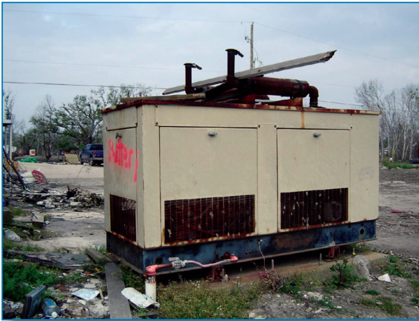
Figure 2-20: Although it was anchored and not displaced by floodwaters, this generator was out of service after being submerged.
