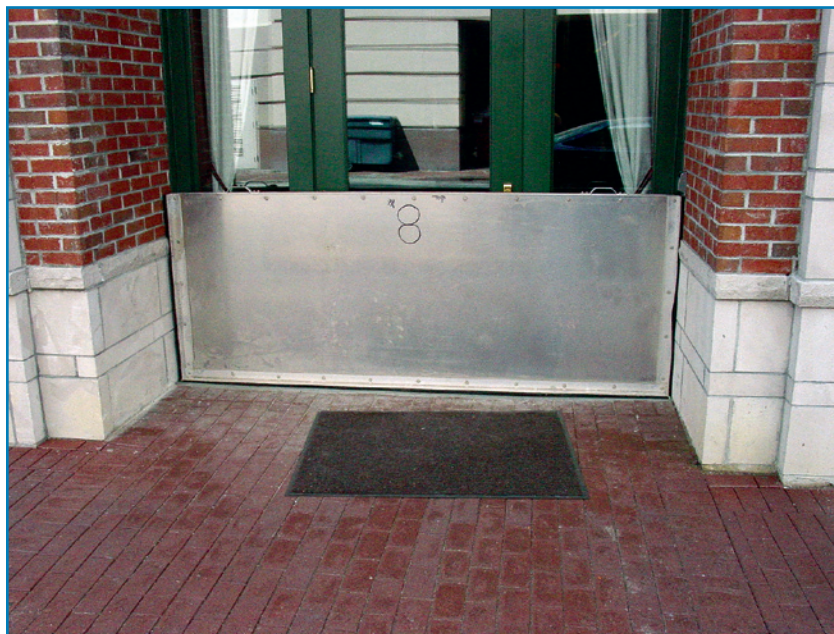
Figure 2-36: Example of an aluminum flood barrier used for flooding less than 3 feet deep. SOURCE: SAVANNAH TRIMS
