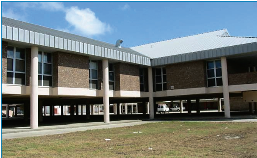
Figure 2-26: School elevated on columns
