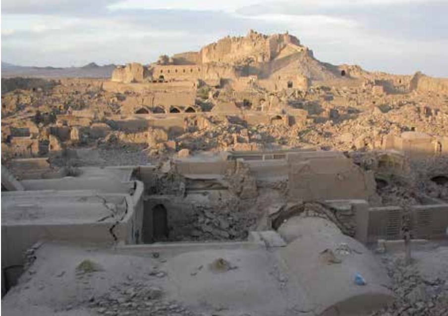
Fig.2 World Heritage Site of Bam; the largest adobe citadel in the world suffered damage during 2003 earthquake.
