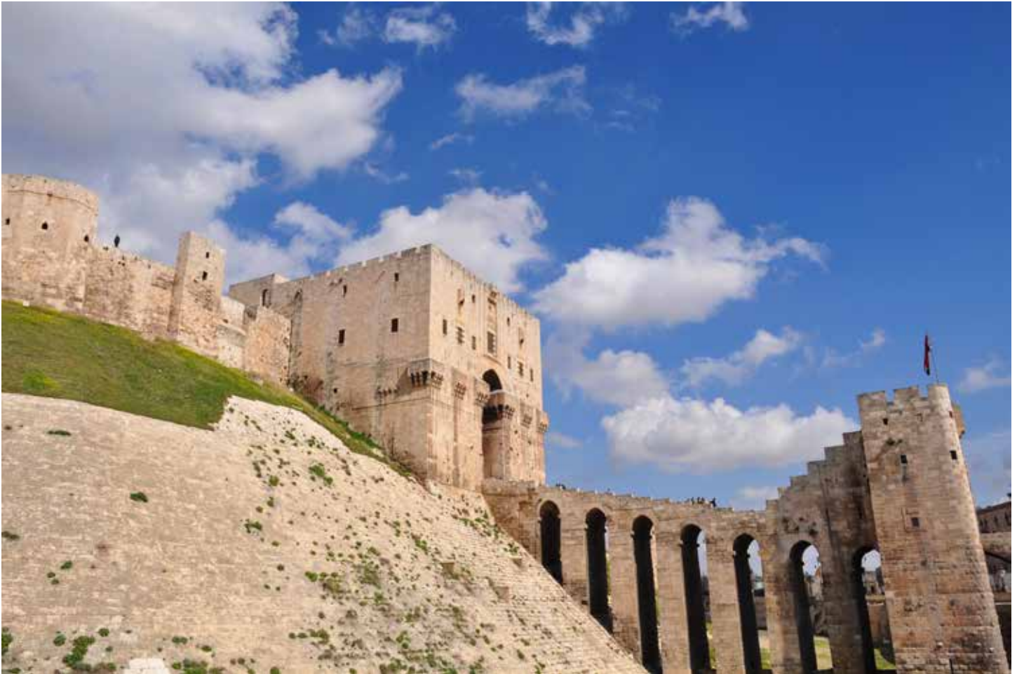
Fig.8 The Citadel at Aleppo, Syria has suffered major damage due to ongoing conflict SOURCE: Silvan Rehfeld, UNESCO. http://whc.unesco.org/en/list/21/gallery/
