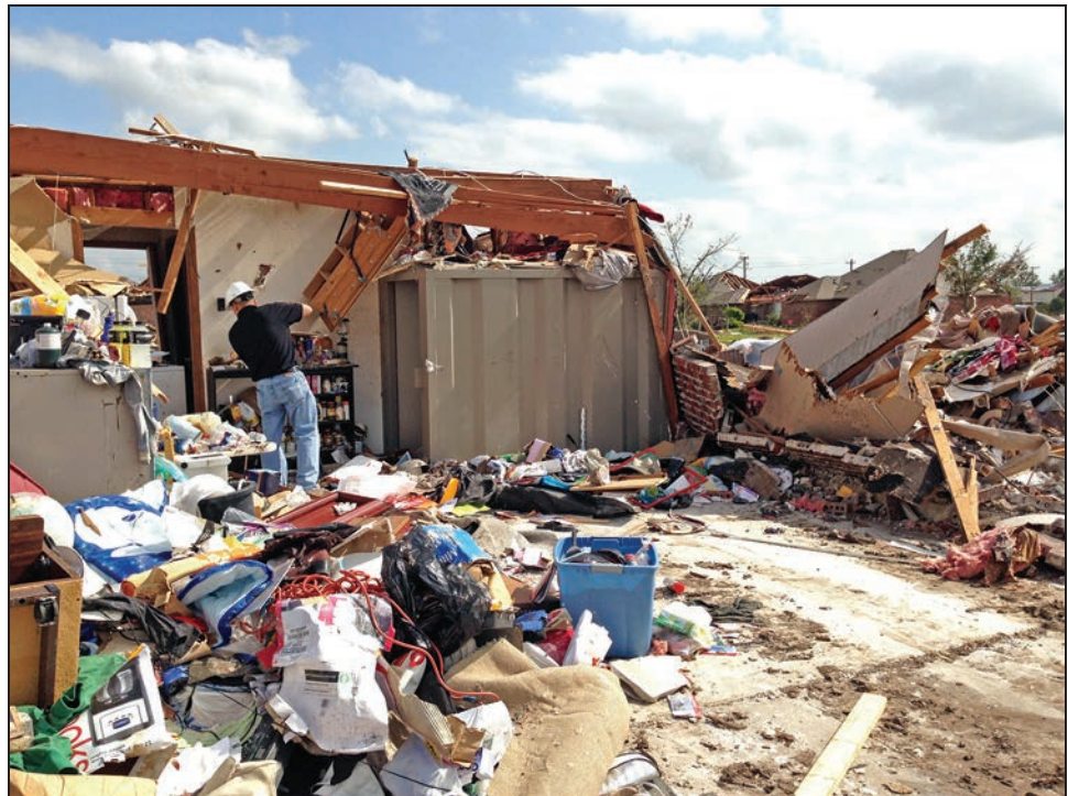
Figure 2. Observation 1: Above-ground shelter that performed well in a heavily damaged area (Oklahoma City, OK)
