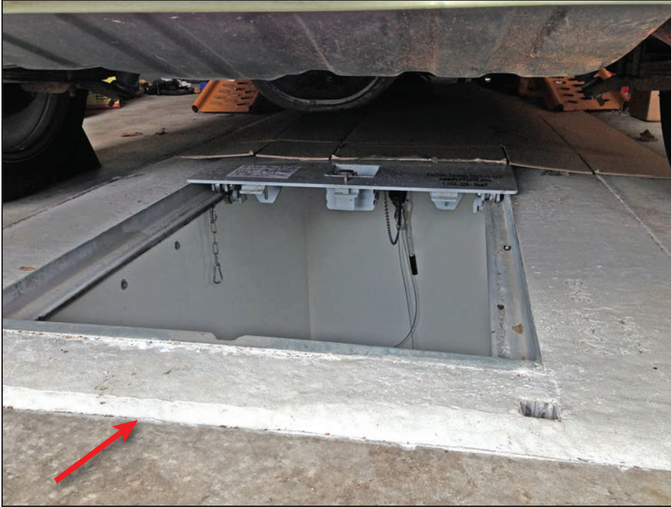
Figure 12. Observation 10: Shelter underneath a car in a garage (Moore, OK). The red arrow shows where the raised lip can help prevent water penetration from minor flooding.
