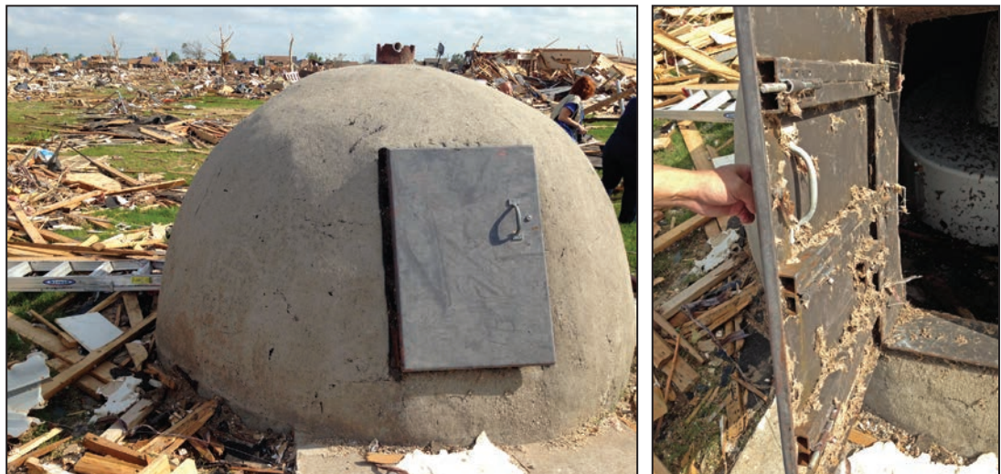
Figure 3. Observation 2: Dome structure within the path of the tornado (left), the inside of the dome structure door was covered with small debris (right) (Oklahoma City, OK)
