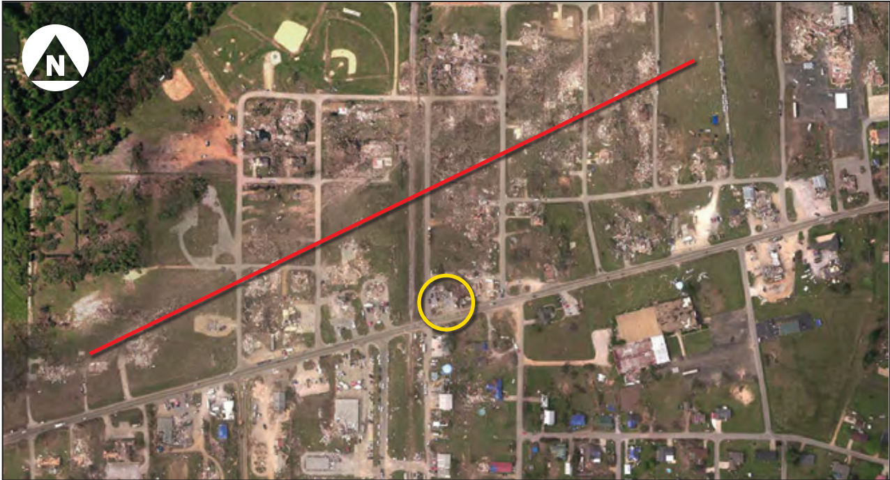
Figure 7-48: Aerial view of the tornado track in the vicinity of the Smithville Police Department (yellow circle). The center of the damage swath is approximated by the red line (Smithville, MS).
