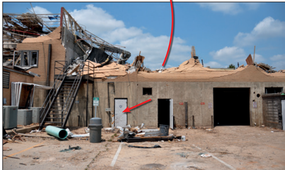
Figure 7-61: The door with the red arrow leads to the EOC area. The inset shows the area above the EOC that collapsed (Tuscaloosa, AL).
