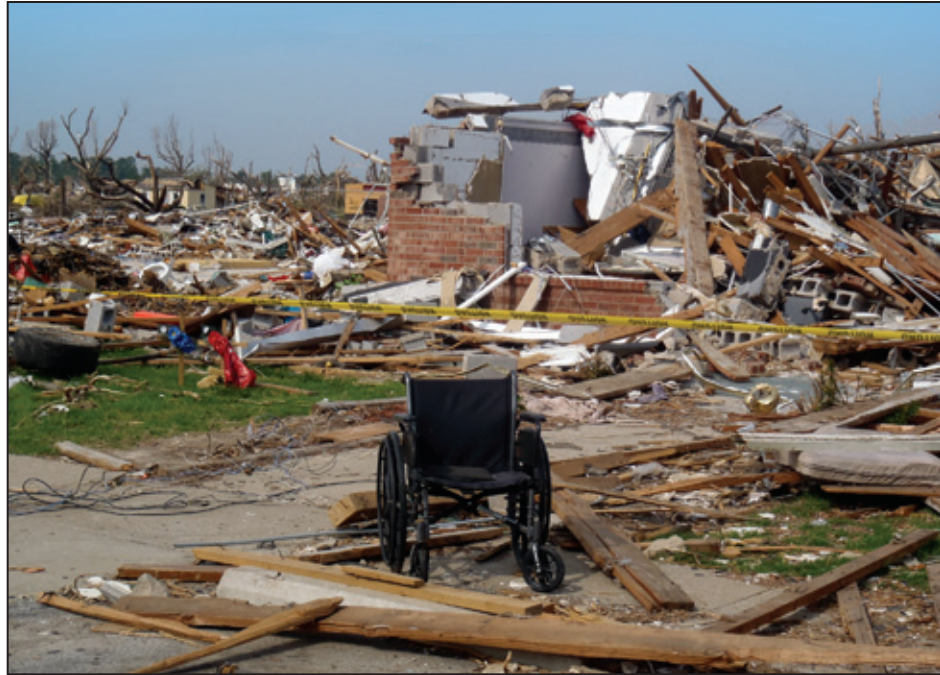
Figure 7-19: Only one wall remained standing at the nursing home (Joplin, MO)
