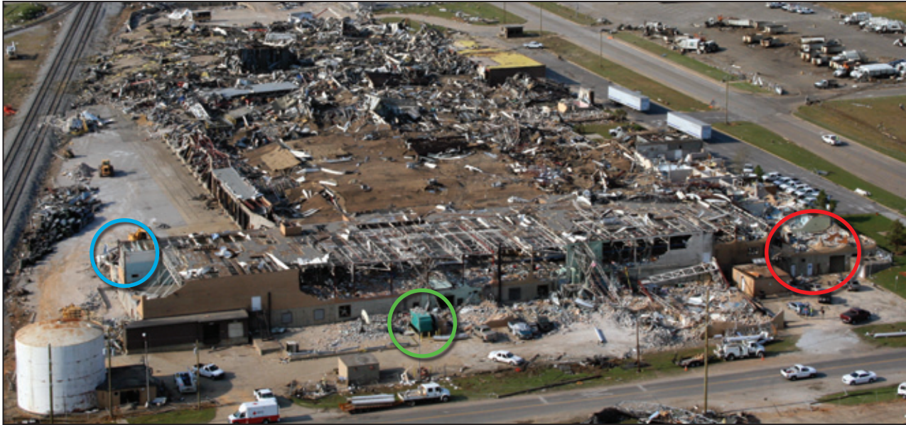
Figure 7-55: Oblique view of Figure 7-54 showing the Curry Building. The green circle indicates the EOC's emergency generator. The red circle shows the ground floor of the southeast corner, the location of the EOC. The blue circle shows the tornado refuge area.
