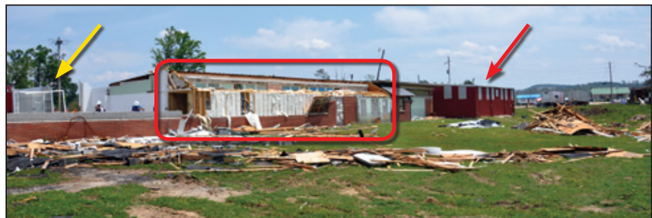
Figure 7-47: View of the back of the building. The old apparatus bay is shown by the yellow arrow and the new bay by the red arrow. Roof structure and wall damage occurred within the red box. The debris in the foreground is from the multipurpose room roof and the old apparatus bay (Wellington, AL).
