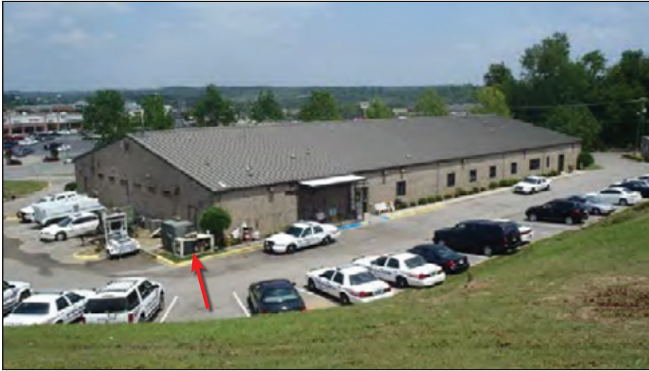
Figure 7-37: Back of the City Hall. The red arrow points to the generator that was disabled by a fallen tree (Fultondale, AL).
