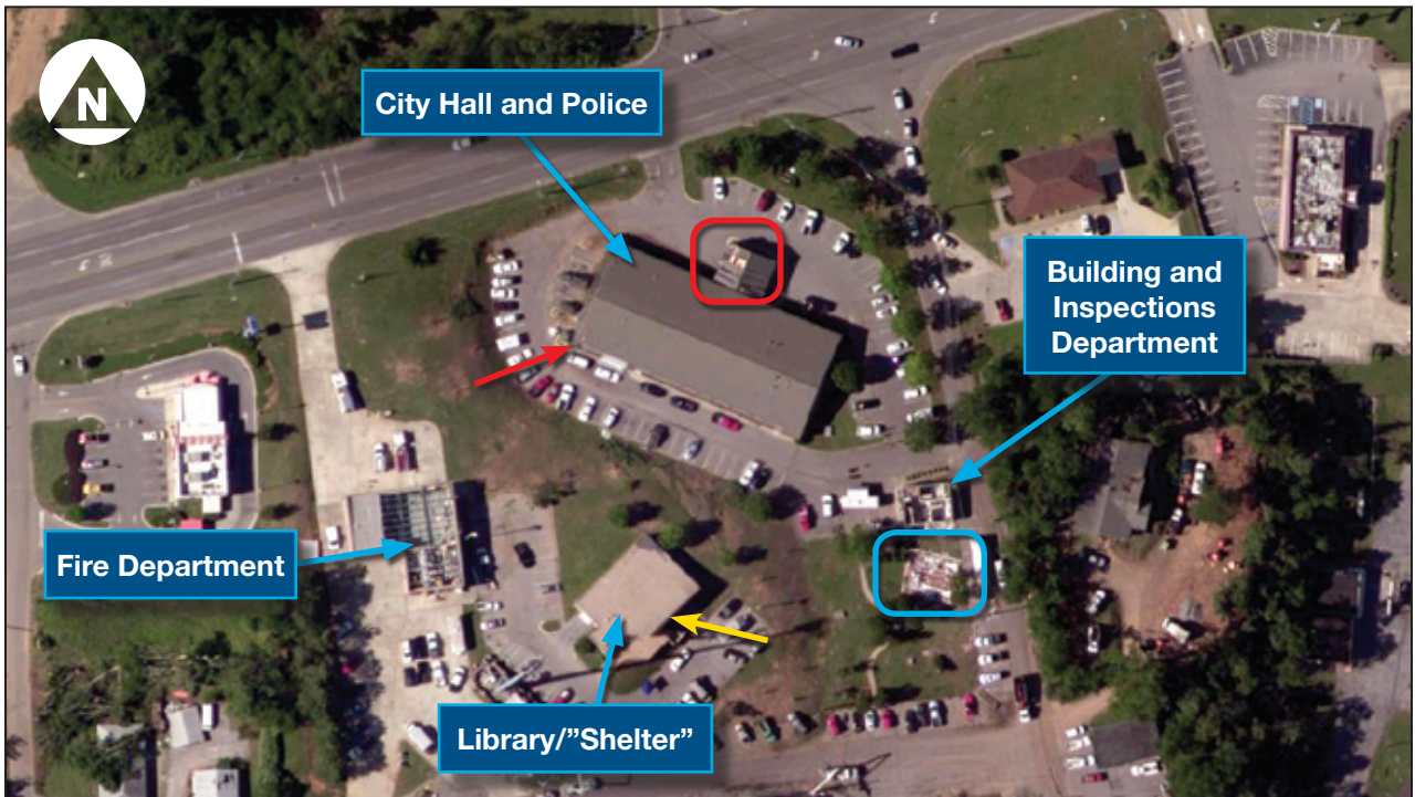
Figure 7-30: Tornado winds damaged an emergency generator (red arrow) and a roof (red box), and lifted a roof (final location shown by blue box). Yellow arrow shows the “shelter” entrance (Fultondale, AL).
