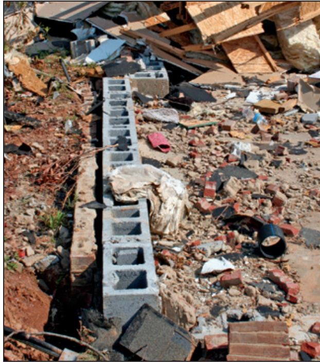
Figure 4-27: Example of wall framing-to-foundation connection failure. Wall and bottom plate separated from foundation where anchorage of collapsed framed wall failed because anchors lacked embedment in grout. Note CMU wall with no reinforcement or solid grout (Harvest, AL). [MAT EF Rating = 2]
