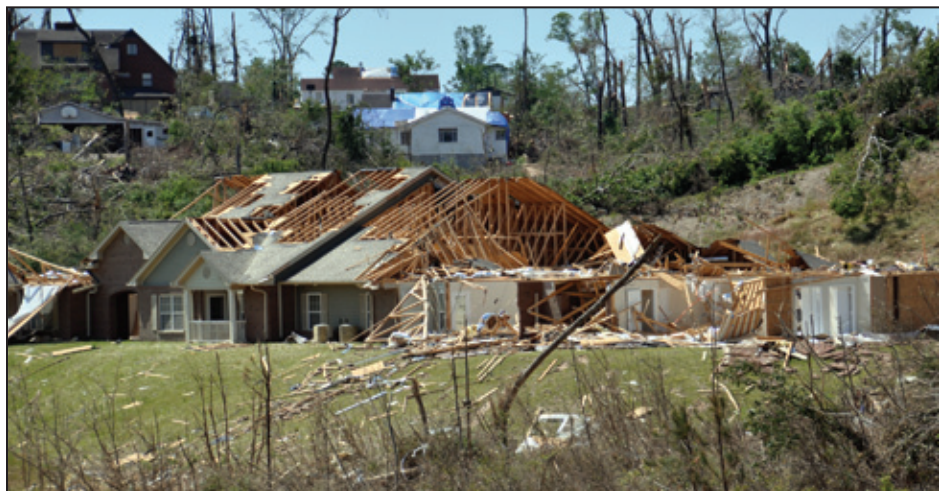
Figure 4-33: One-story Chastain Manor Apartments suffered damage varying from roof decking uplift to collapse of roof structure
