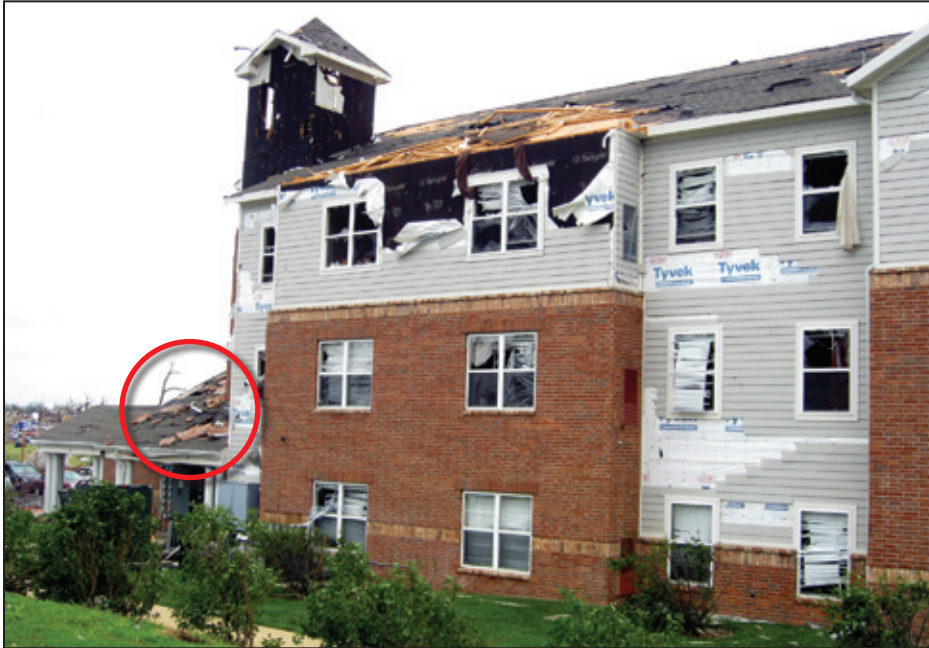
Figure 4-43: West wall and elevator tower where brick fell off and damaged one-story roof (red circle)
