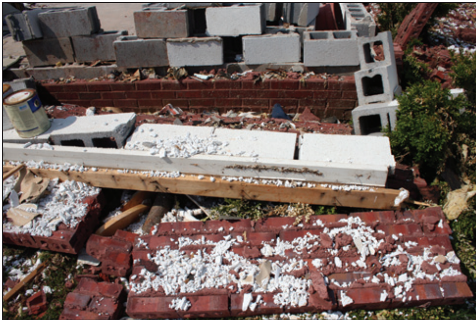
Figure 4-28: Example of wall framing-to-foundation connection failure. Bottom plate remains connected to top row of CMU, but CMU wall failed due to lack of reinforcement for continuous load path (Harvest, AL). [MAT EF Rating = 2]
