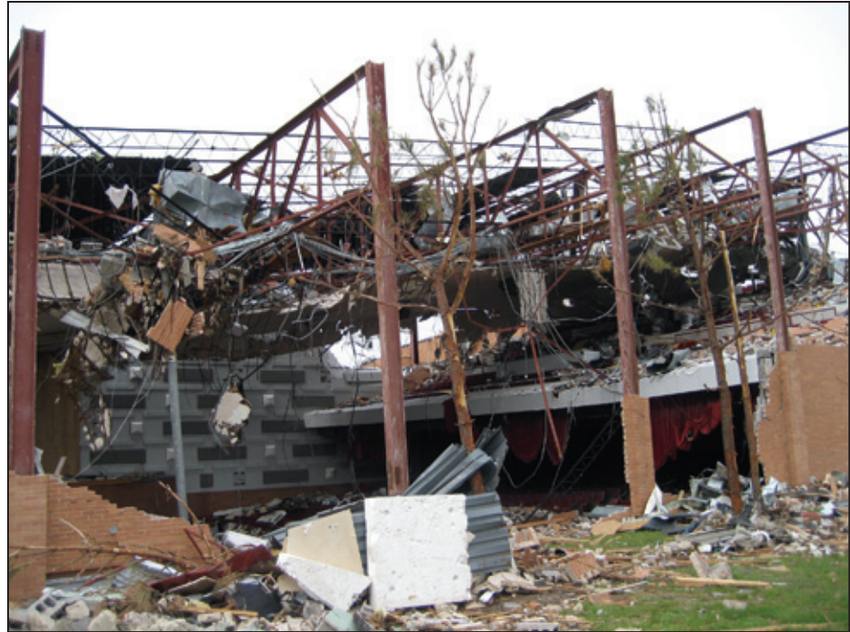
Figure 6-56: North wall of the auditorium (Joplin, MO)
