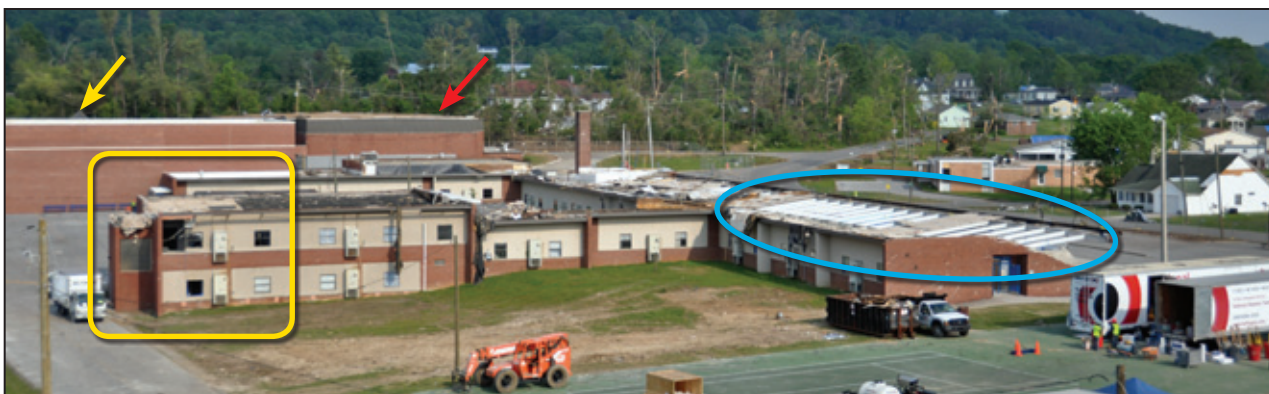
Figure 6-34: View of the Ringgold Middle School (the inset shows the left portion of the school). The 2008 auxiliary gymnasium (yellow arrow) and original gymnasium (red arrow) are shown. Most of the roof deck was lost in the area shown by the blue oval. The yellow box indicates an area where walls and glazing were damaged (Ringgold, GA).
