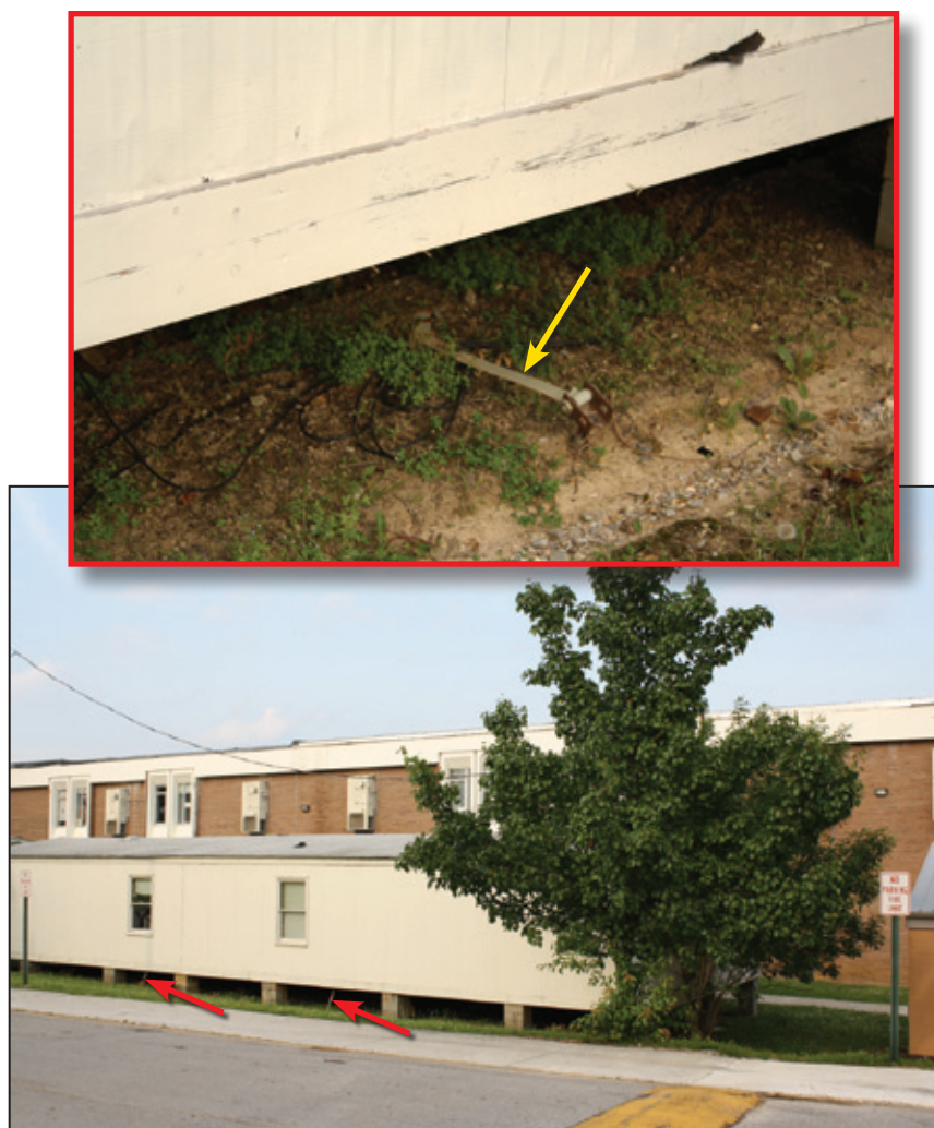
Figure 6-25: View of one of the portable classrooms. The red arrows indicate anchor straps. The strap shown in the inset had corroded through (yellow arrow) (Ringgold, GA).
