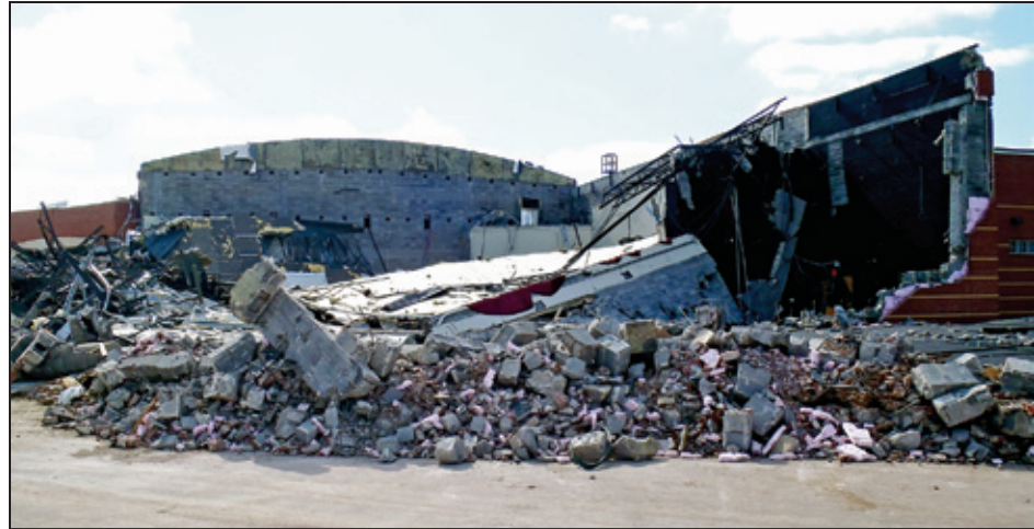
Figure 6-42: View of the collapsed auditorium roof and both exterior walls (Joplin, MO)
