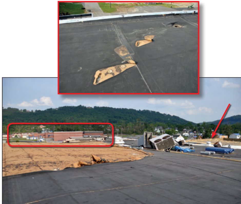
Figure 6-27: View of the two gymnasium roofs. The red arrow shows the 2008 auxiliary gymnasium (see also Figures 6-26 and 6-28). The EPDM (black) membrane is over the original gymnasium. Note the displaced rooftop equipment. The red box shows a portion of the middle school beyond. The inset shows wind-borne debris damage to the EPDM roof (Ringgold, GA).
