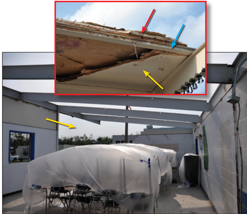
Figure 6-36: View from within a classroom. The yellow arrow shows the area of the collapsed wall that is shown in Figure 6-35. In this area, the deck bulb-tees also blew off. The inset shows an area of this wing where some form-board (yellow arrow), a bulb-tee (blue arrow), and the gypsum deck (red arrow) were still in place (Ringgold, GA).
