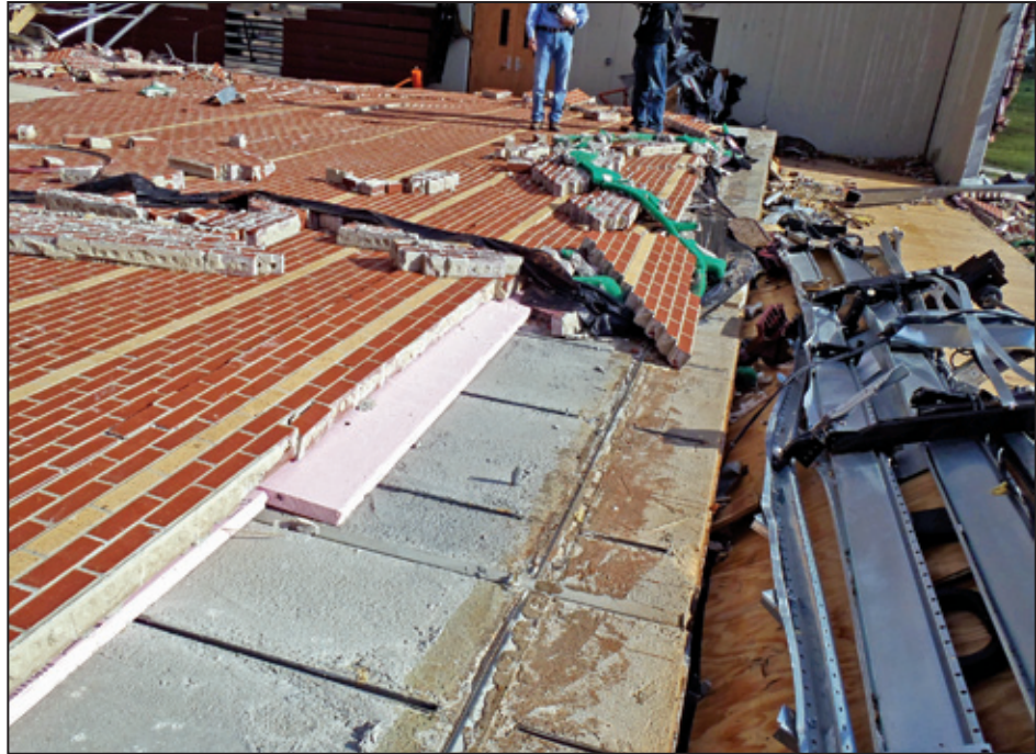
Figure 6-46: Brick veneer/insulation/ precast concrete wall on the gymnasium floor (Joplin, MO)
