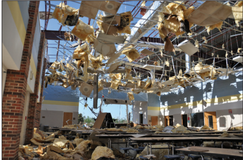
Figure 6-17: View inside the cafeteria (Tuscaloosa, AL)
