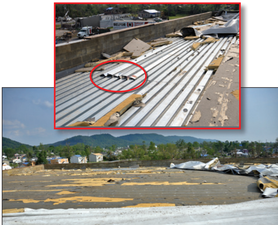
Figure 6-28: View of the roof of the 2008 auxiliary gymnasium (see also red arrow in Figure 6-27); inset shows lifted decking (red circle) (Ringgold, GA)
