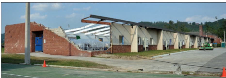
Figure 6-35: This wing lost most of its roof decking, and a portion of the brick veneer and unreinforced CMU collapsed (Ringgold, GA)
