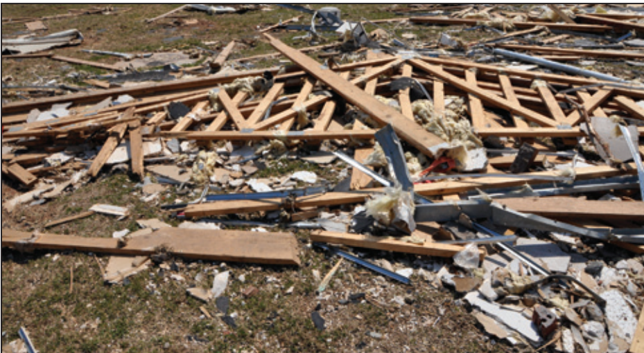
Figure 3-7: Example of medium- to large-sized wind-borne missiles (photograph shows roof trusses displaced from a nearby building in Tuscaloosa, AL)
