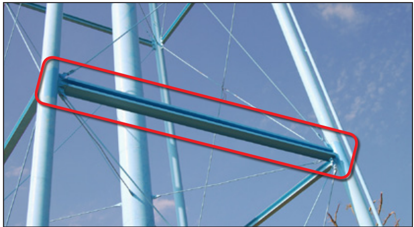
Figure 8-10: Debris impact damage to Smithville, MS, water tank: photograph on left shows where debris struck the water tank itself (red circle) and photograph on right shows the repaired compression strut that was damaged by wind-borne debris (red box)
