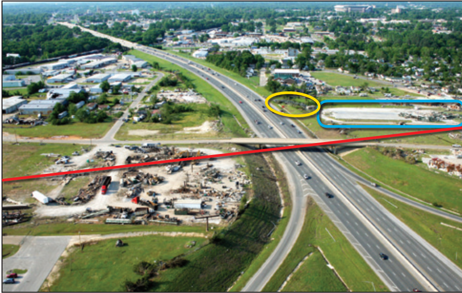
Figure 8-22: View of the collapsed 300-foot cellular tower (yellow oval) and the destroyed metal building southeast of the tower (blue box) in relation to the approximate centerline of the tornado damage swath (red line) (Tuscaloosa, AL)
