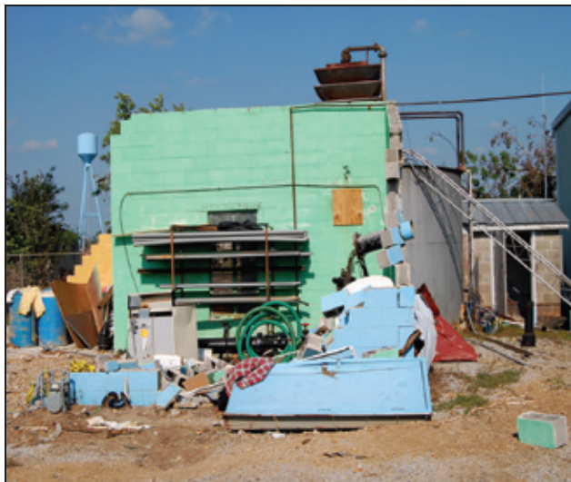
Figure 8-8: Destroyed unreinforced CMU building (left) and damaged metal-framed building (right) (Smithville, MS)
