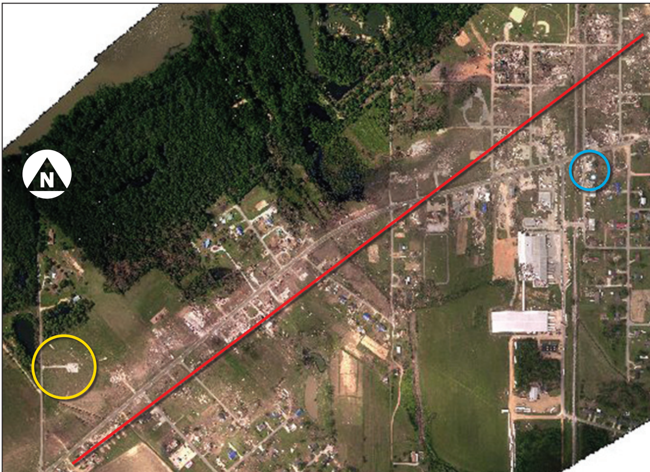
Figure 8-5: Aerial view showing the approximate centerline of the tornado damage swath in Smithville, MS (red line), the Smithville Water Treatment and Distribution System Plant (blue circle), and the 300-foot-tall cellular tower discussed in Section 8.3.2.1 (yellow circle)
