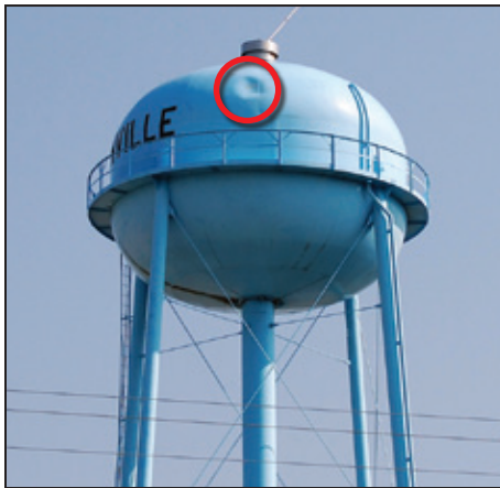
Figure 8-10: Debris impact damage to Smithville, MS, water tank: photograph on left shows where debris struck the water tank itself (red circle) and photograph on right shows the repaired compression strut that was damaged by wind-borne debris (red box)
