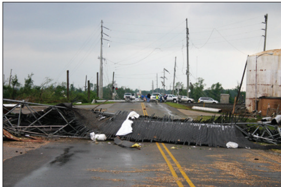
Figure 8-15: View of toppled EMS communications tower taken by EMS personnel after the tornado. Note the wind-displaced material (discussed in text) adhered to the tower (Tuscaloosa, AL).
