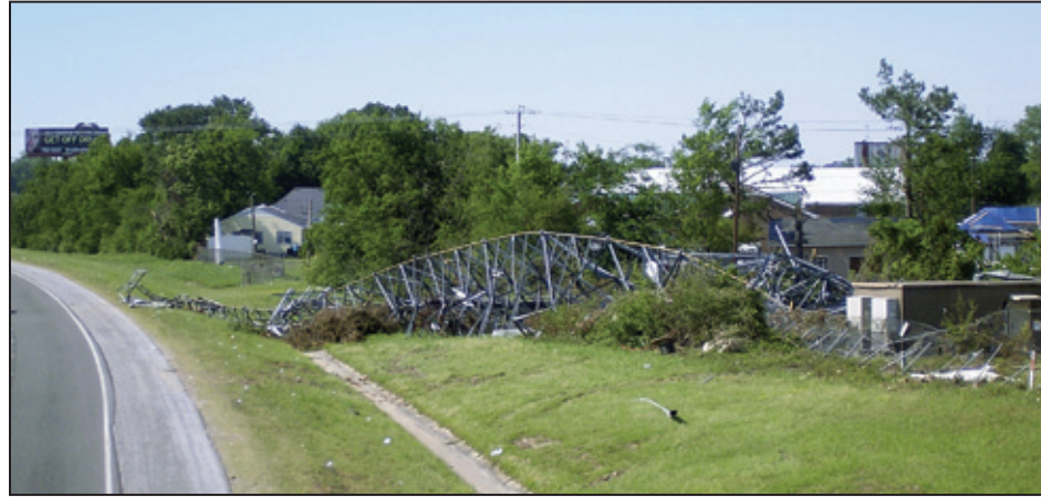
Figure 8-20: View of the 300-foot latticed cellular tower that collapsed during the tornado event (Tuscaloosa, AL)
