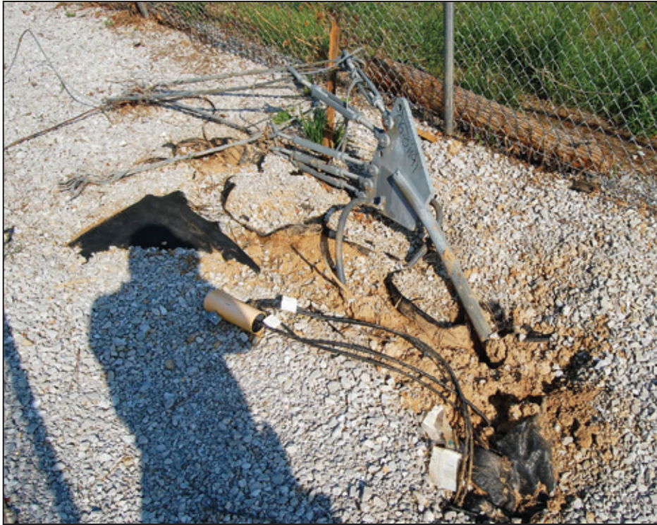
Figure 8-31: The anchor securing one guy was dragged several feet through the ground (Smithville, MS)
