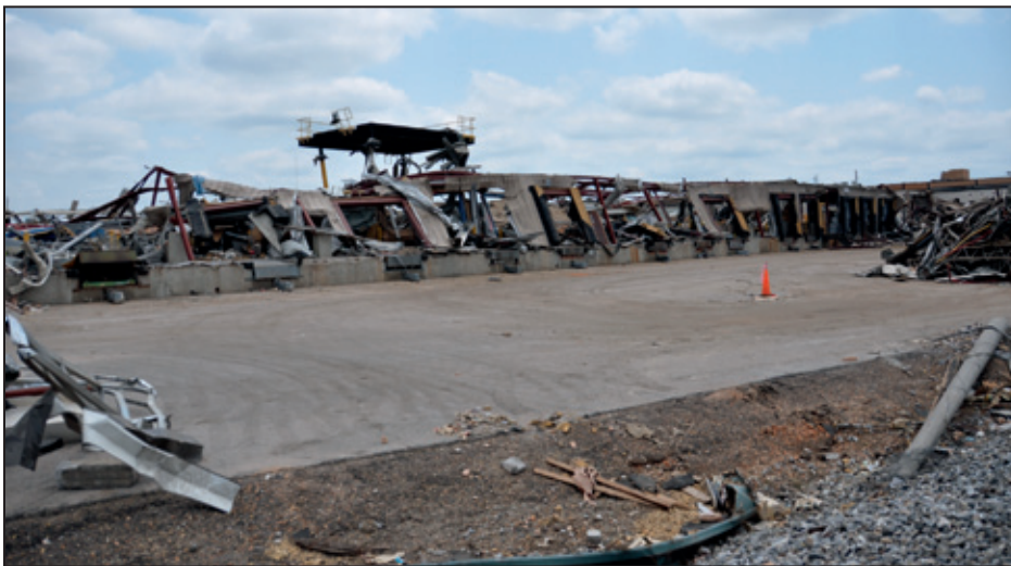
Figure 7-58: View of a portion of a collapsed loading dock area (Tuscaloosa, AL)
