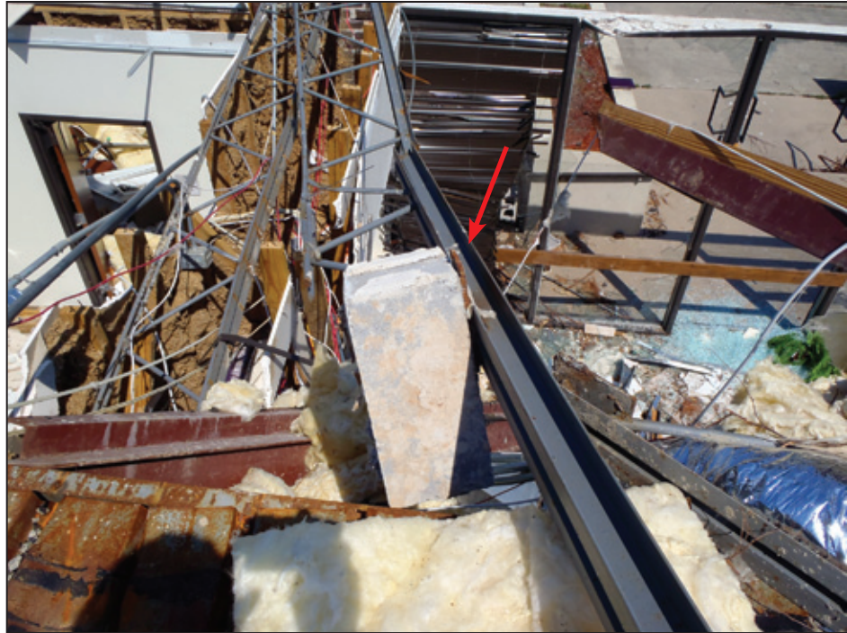
Figure 5-29: Bar joist with embed plate and bond beam cell still attached (red arrow) (Birmingham, AL)
