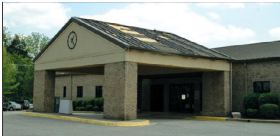
Figure 7-36: The front of the City Hall showing damage to the metal roof covering over the entrance (Fultondale, AL)
