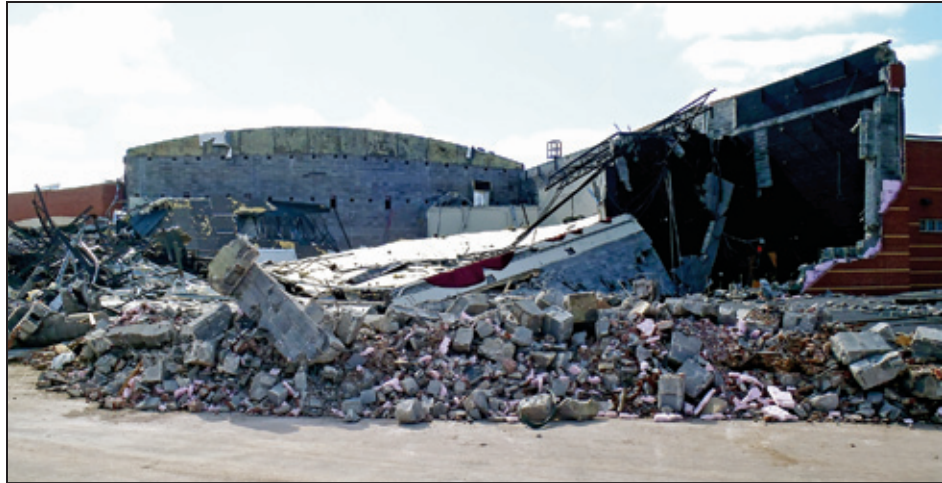
Figure 6-42: View of the collapsed auditorium roof and both exterior walls (Joplin, MO)
