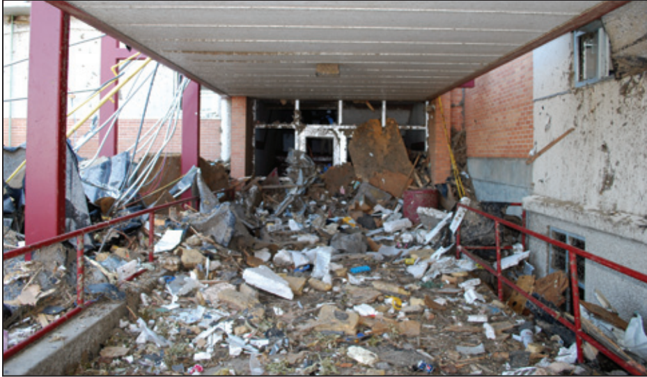
Figure 3-17: Large pile of small- and medium-sized wind-borne debris outside of Joplin High School (Joplin, MO)
