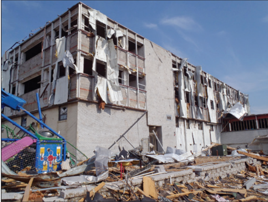
Figure 5-55: East elevation of the Ozark Center for Autism showing damage to glazing and siding (Joplin, MO).
