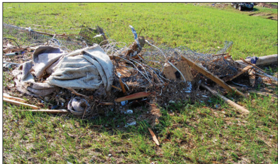
Figure 8-30: Wind-displaced building materials wrapped around the 300-foot cellular tower guy (Smithville, MS)
