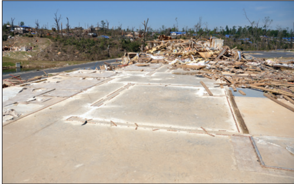
Figure 4-36: Example of DOD 6 showing two-story Chastain Manor Apartments completely destroyed by the tornado with slabs swept clean
