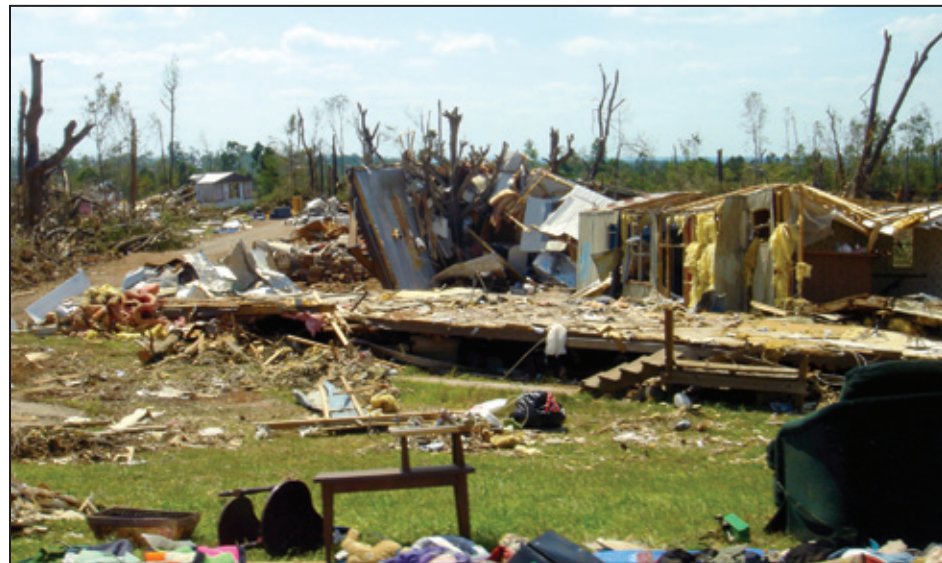
Figure 9-7: Manufactured homes destroyed in Crescent Ridge, AL (location shown in Figure 9-4)
