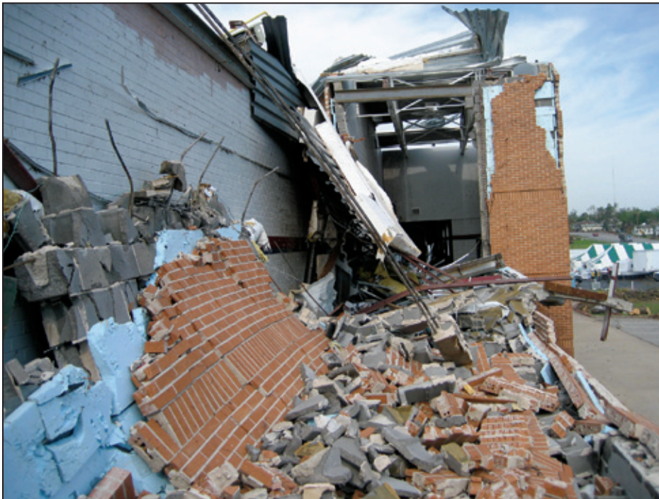
Figure 11-2: Collapse of exterior CMU/ brick veneer wall and roof collapse at the Joplin High School (Joplin, MO). The wall debris fell into the corridor.
