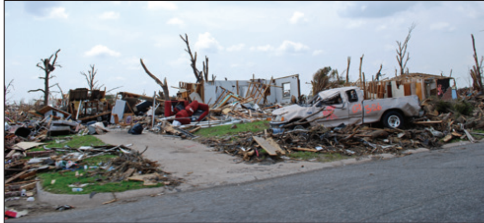
Figure 9-6: The core remnant of a home in Joplin, MO
