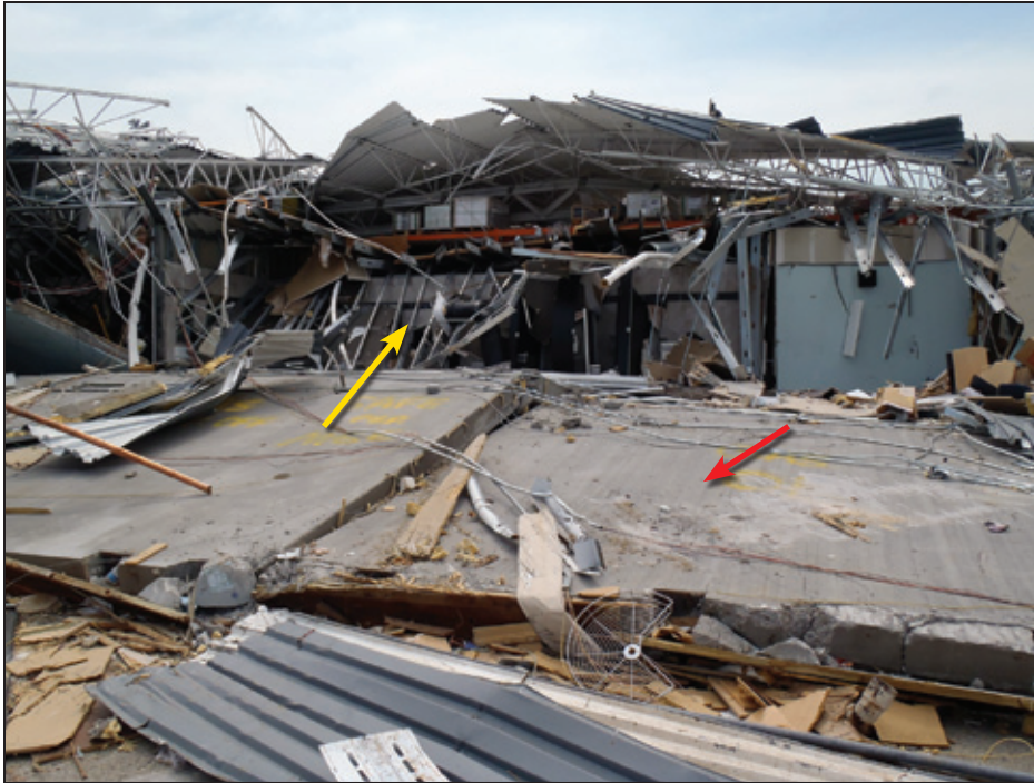
Figure 9-17: Tornado refuge area (training room) of the Home Depot. Note the collapsed tilt-up wall (red arrow) and the wall leaning into the refuge area (yellow arrow) (Joplin, MO).
