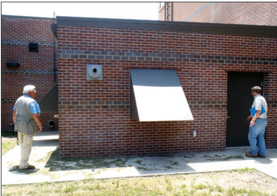
Figure 9-46: Emergency generator building for the community safe room at the Seneca Intermediate School
