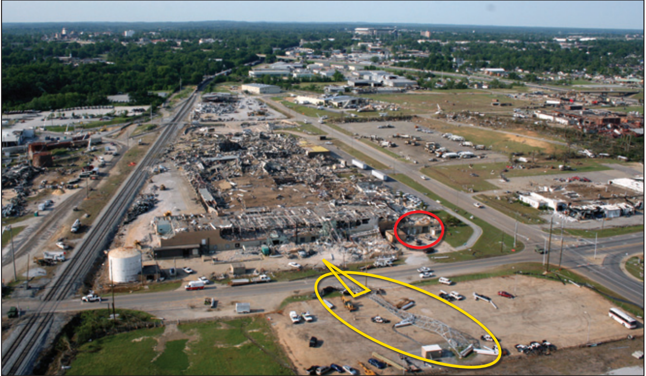
Figure 8-16: View of the collapsed EMS communications tower (yellow oval); the EOC across 35th Street is also shown (red oval) (Tuscaloosa, AL). The communications tower was cut, and the debris that was across the road was removed (yellow triangle).
