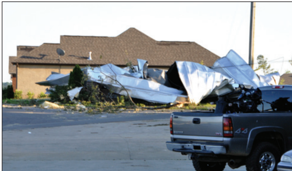
Figure 3-12: Metal sheathing travelled 200 feet as wind-borne debris and landed next to a building outside of the tornado swath (Fultondale, AL)
