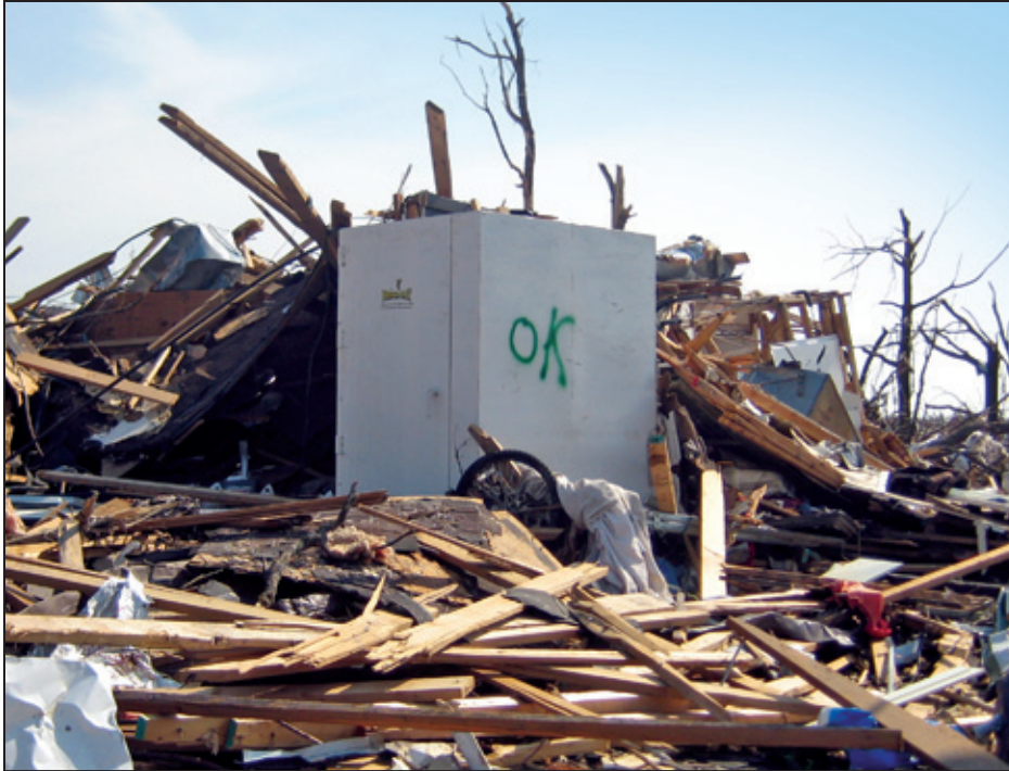
Figure 9-2: Above-ground residential safe room installed in a garage of a home in Joplin, MO, directly impacted by the tornado (rated EF4 based on the MAT's observations)
