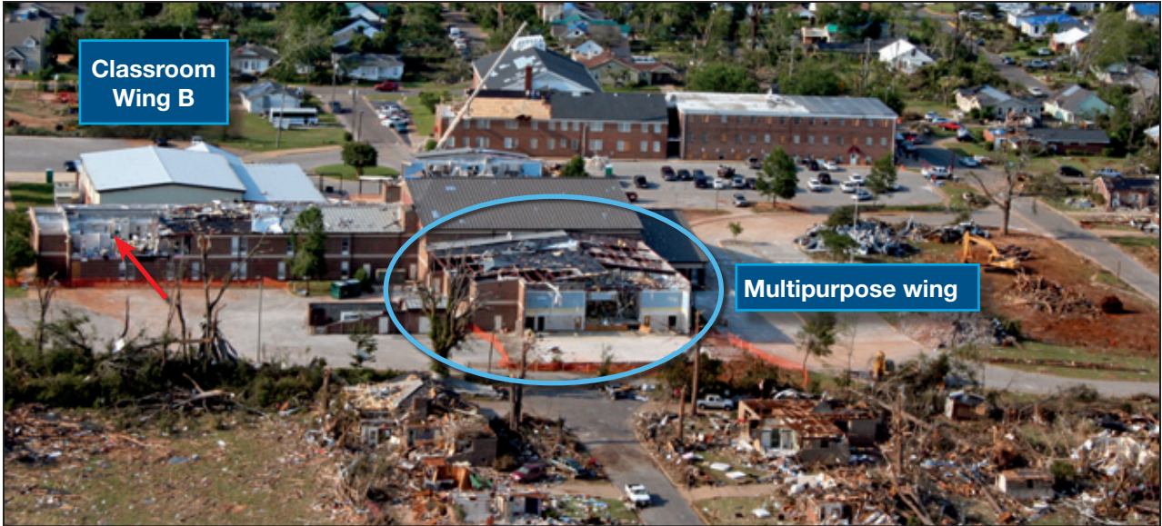
Figure 6-15: View looking north showing wall and roof structure damage to classroom wing B (red arrow) and damage to the multipurpose wing (blue oval) (Tuscaloosa, AL)
