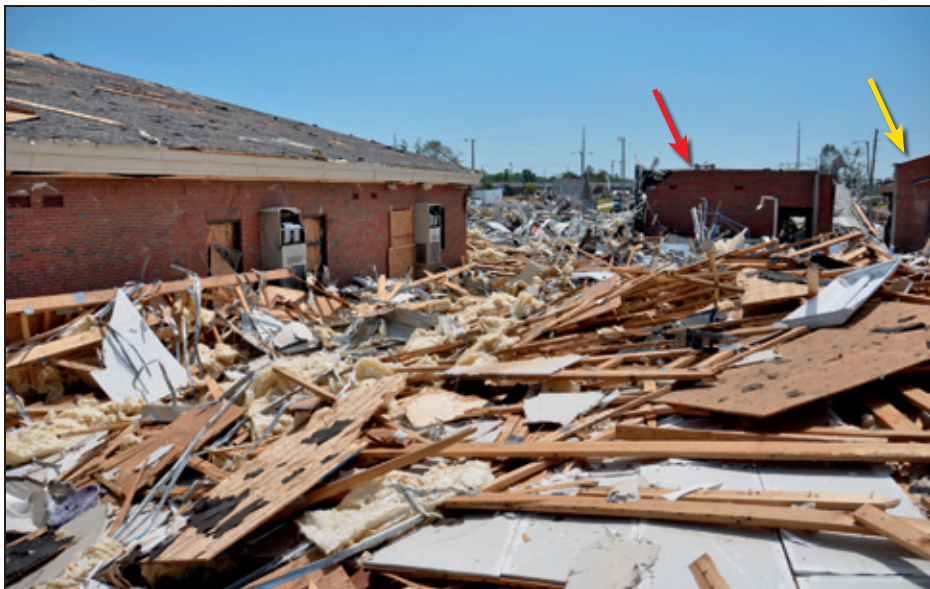
Figure 6-9: Looking down the corridor of the collapsed classroom wing; red arrow indicates a bathroom in the core remnant and yellow arrow indicates a corridor that remained standing (Tuscaloosa, AL)
