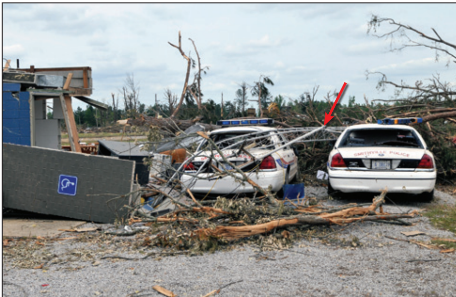
Figure 7-51: Smithville Police Department. Note the collapsed communications tower (red arrow) (Smithville, MS).
