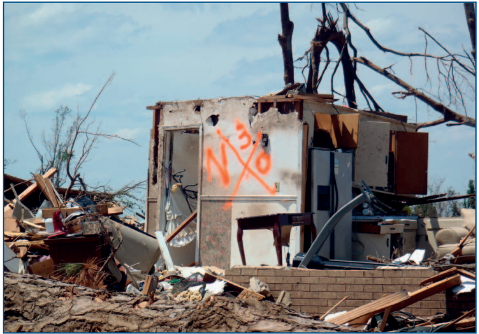
View of remnants of an interior room of a house that survived a strong tornado (Tuscaloosa, AL).
