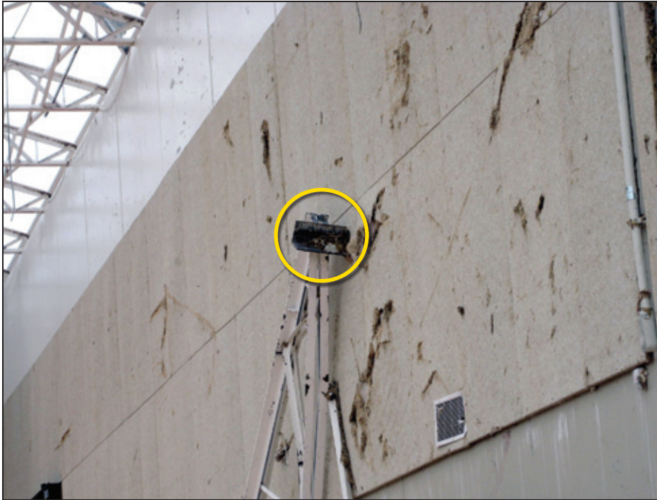
Figure 6-44: View of the end of the collapsed truss (yellow circle) shown in Figure 6-43 (Joplin, MO)
