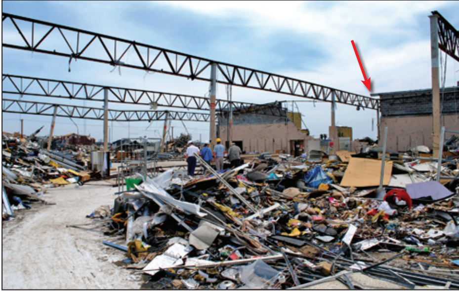
Figure 5-41: Roof structure remaining in south half of Walmart. The red arrow shows the location of a column embedded in the wall (Joplin, MO).
