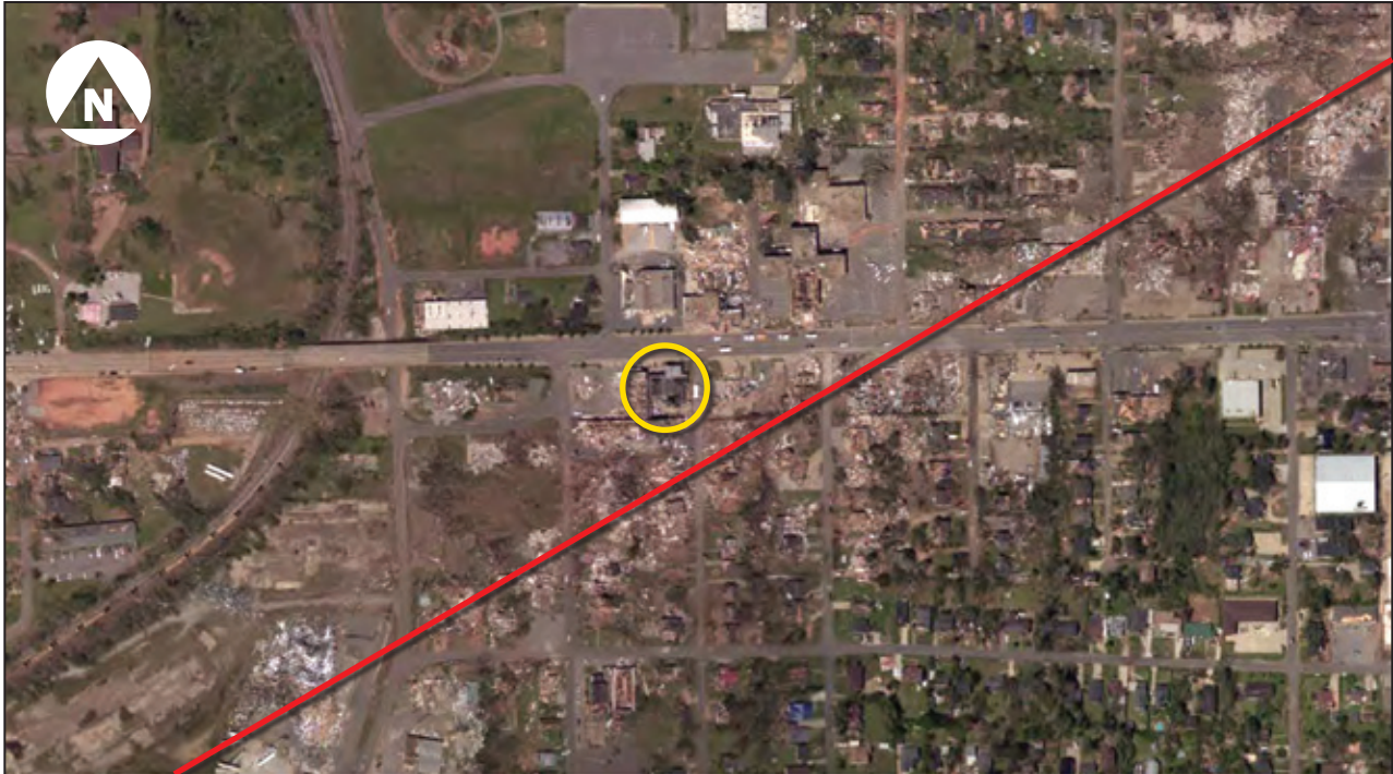
Figure 7-38: Aerial view of the track in the vicinity of the fire station (yellow circle). The center of the damage swath is approximated by the red line (Tuscaloosa, AL).
