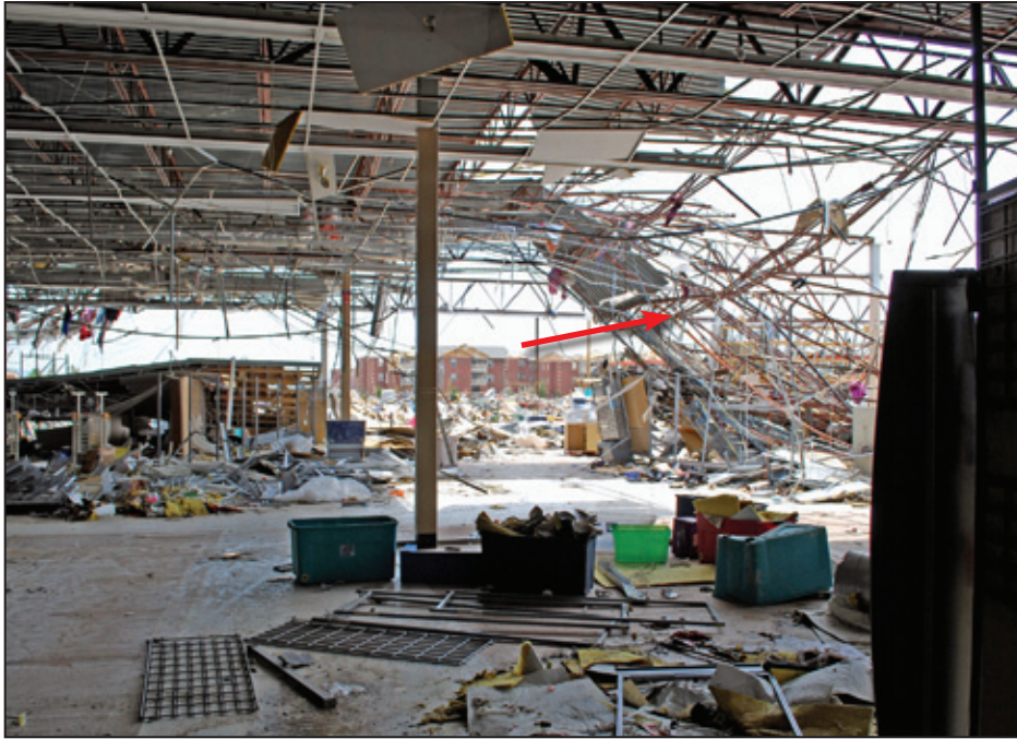
Figure 5-33: Interior of the north half of the Walmart, looking east. Fallen roof structure shown in right side of the picture (red arrow) (Joplin, MO).
