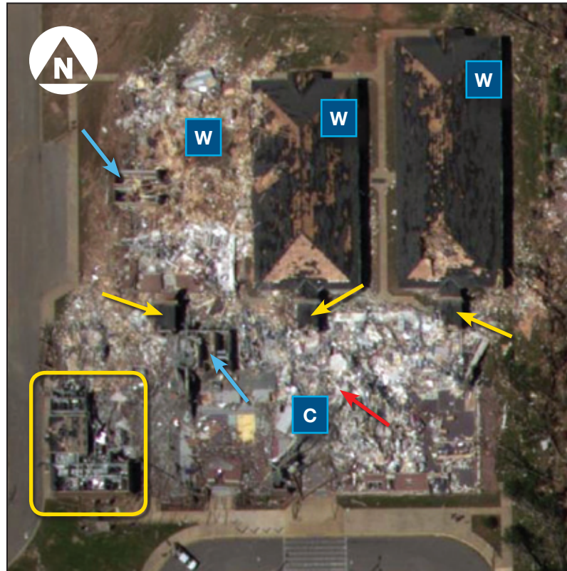
Figure 6-4: Area shown in yellow circle of Figure 6-3. The classroom wings are indicated by “W” and the core area by “C.” The general location of the tornado refuge areas for the two surviving wings is shown by the red arrow. Yellow arrows indicate remnants of corridors between the core and wings. The blue arrows indicate restroom remnants. The yellow box indicates kitchen remnants (Tuscaloosa, AL).
