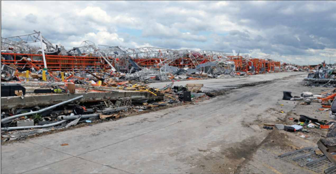
Figure 9-16: Home Depot after the May 22, 2011 tornado (Joplin, MO)
