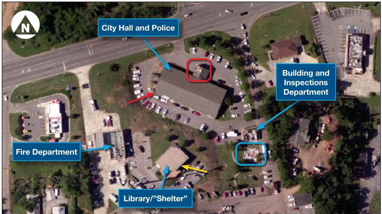
Figure 7-30: Tornado winds damaged an emergency generator (red arrow) and a roof (red box), and lifted a roof (final location shown by blue box). Yellow arrow shows the “shelter” entrance (Fultondale, AL).
