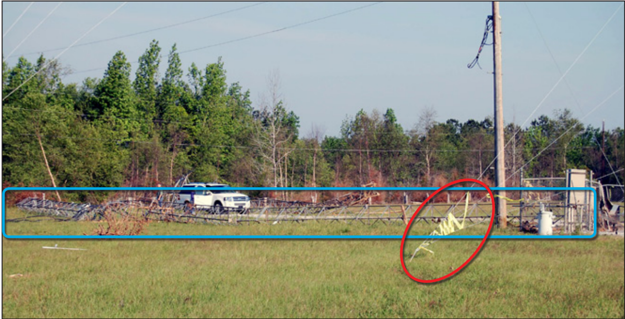
Figure 8-29: Collapsed 300-foot cellular tower (blue box). The triple guy in the foreground (red oval) is one of the three supports for the temporary tower on the site (Smithville, MS).
