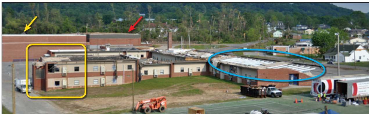
Figure 6-34: View of the Ringgold Middle School (the inset shows the left portion of the school). The 2008 auxiliary gymnasium (yellow arrow) and original gymnasium (red arrow) are shown. Most of the roof deck was lost in the area shown by the blue oval. The yellow box indicates an area where walls and glazing were damaged (Ringgold, GA).
