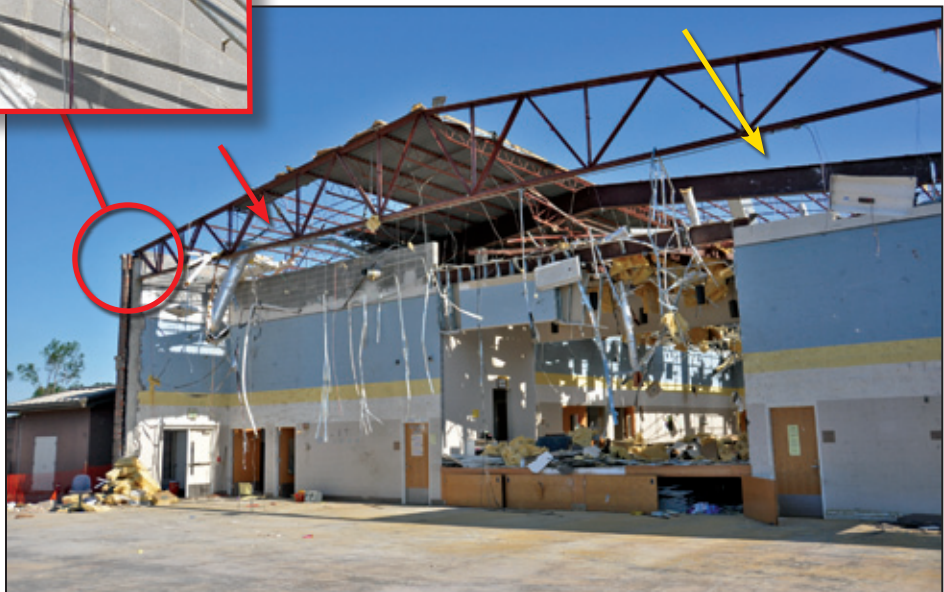
Figure 6-18: View toward the cafeteria (yellow arrow) and kitchen (red arrow) from within the multipurpose room. The inset shows a multipurpose room girder supported by a concrete column that is still in place (Tuscaloosa, AL).
