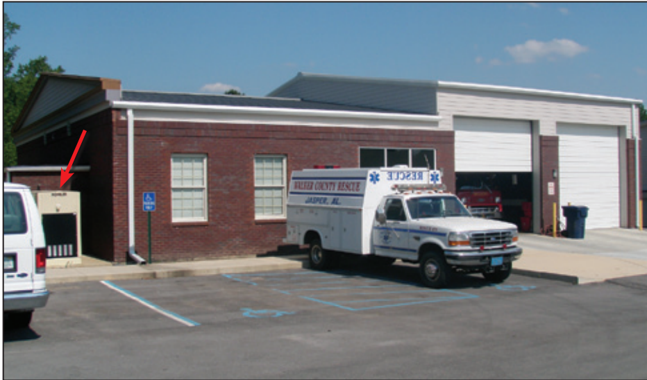
Figure 9-38: A large site-built, below-grade community safe room is housed below this fire station; the red arrow indicates an unprotected generator (Brookside, AL)
