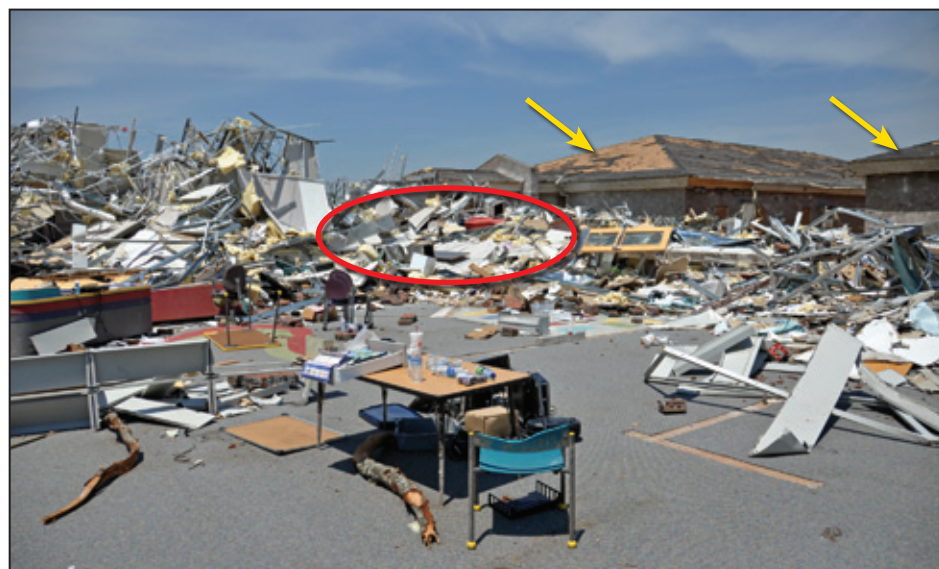
Figure 6-5: View of the central core area. Tornado refuge areas for the two surviving wings were in the collapsed area (red circle). The yellow arrows indicate the two surviving wings (Tuscaloosa, AL).
