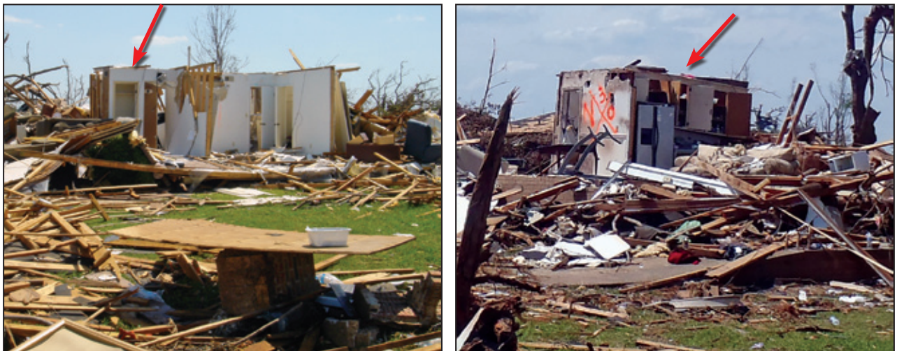
Figure 9-5: Core remnants of homes sometimes survive a tornado as shown in this photograph of site-built homes where a closet (red arrow in left photograph) and a bathroom behind a kitchen (red arrow in right photograph) remained standing after the tornado (Crescent Ridge, AL)
