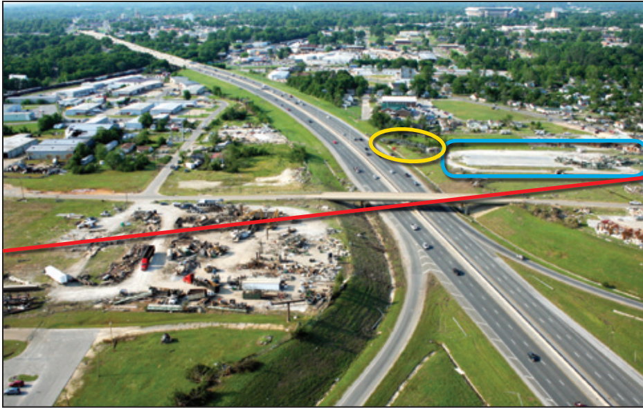
Figure 8-22: View of the collapsed 300-foot cellular tower (yellow oval) and the destroyed metal building southeast of the tower (blue box) in relation to the approximate centerline of the tornado damage swath (red line) (Tuscaloosa, AL)
