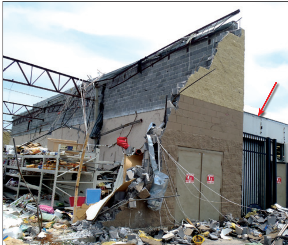
Figure 5-43: Partial collapsed wall in southern half of store (note deck support angle at top of wall); area of limited damage shown by red arrow (Joplin, MO)
