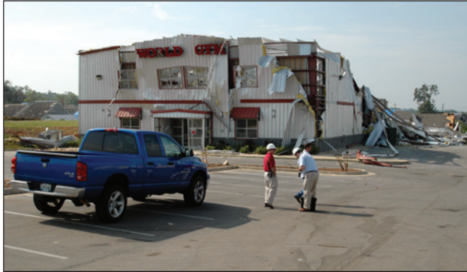
Figure 5-47: Front (north side) of fitness center building (Tuscaloosa, AL)
