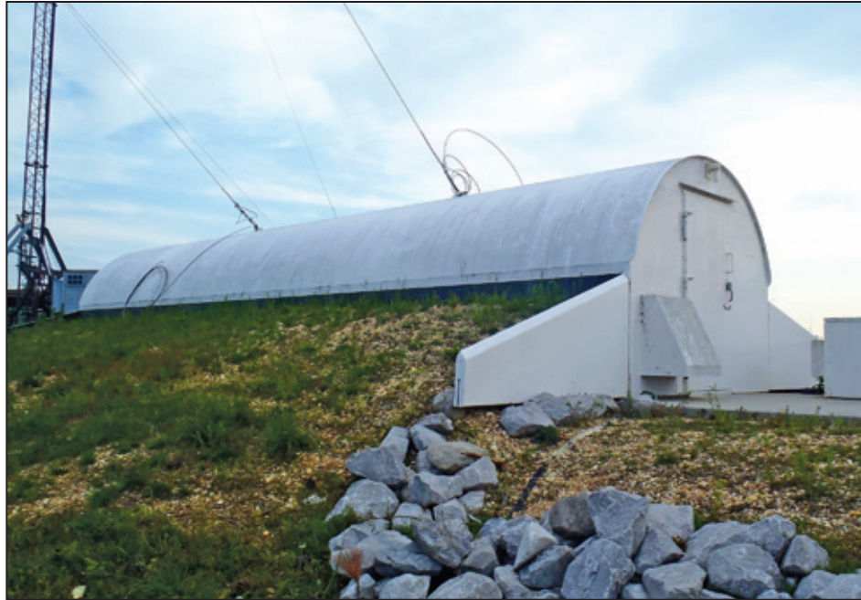
Figure 9-36: FEMA-funded community safe room; guy wires for the temporary communications tower should not be attached to the structure (Phil Campbell, AL)
