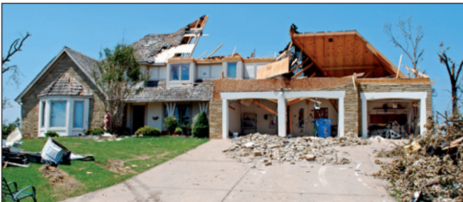
Figure 4-10: Example of how garage door failure (DOD 4) initiated progressive failure, including loss of the garage roof (DOD 6) (Joplin, MO) [MAT EF Rating = 2]
