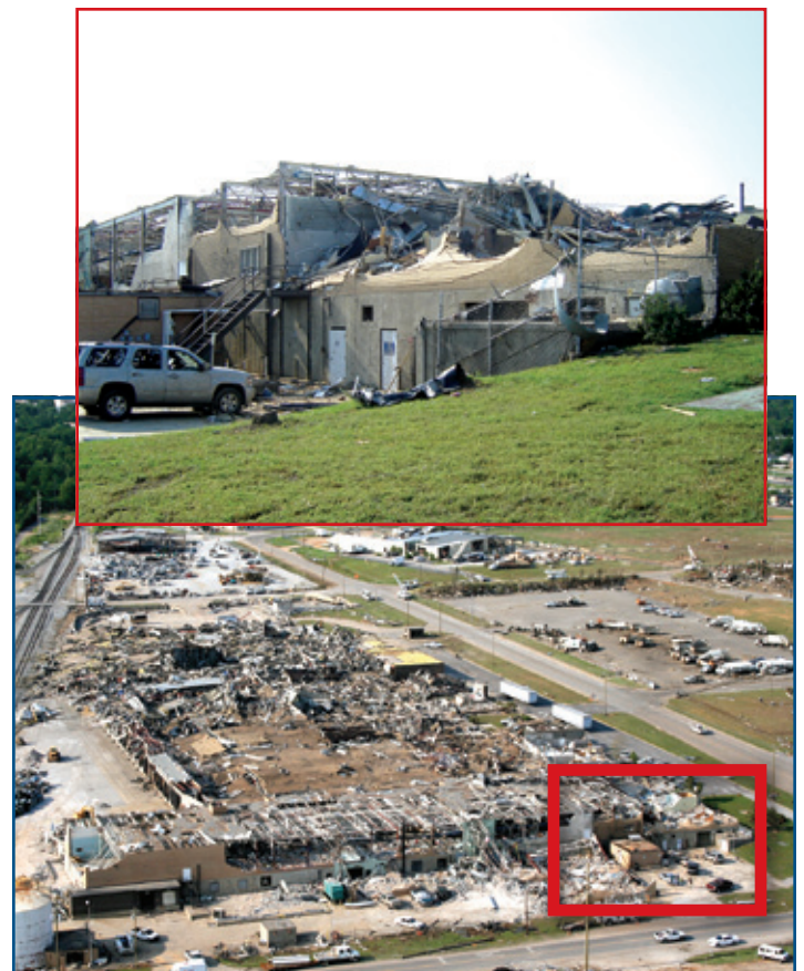
Figure 1: An EOC in Tuscaloosa, AL, that saw a loss of operations but remained intact even though the story above it collapsed (Tornado 2011)
