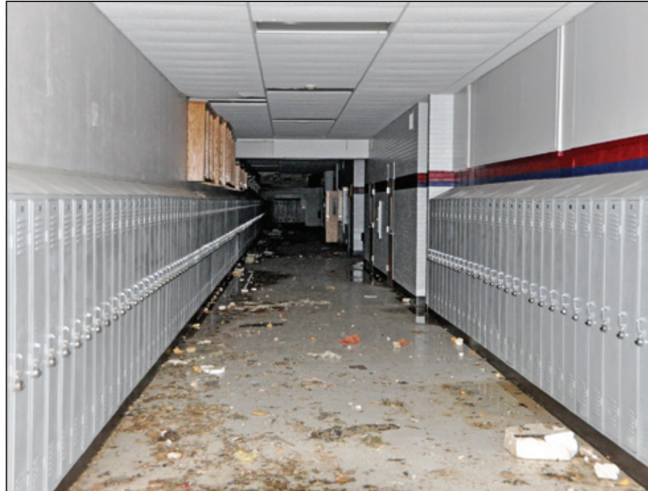
Figure 6-50: View of a corridor designated as tornado refuge area. The debris was blown into the corridor during the tornado (Joplin, MO).
