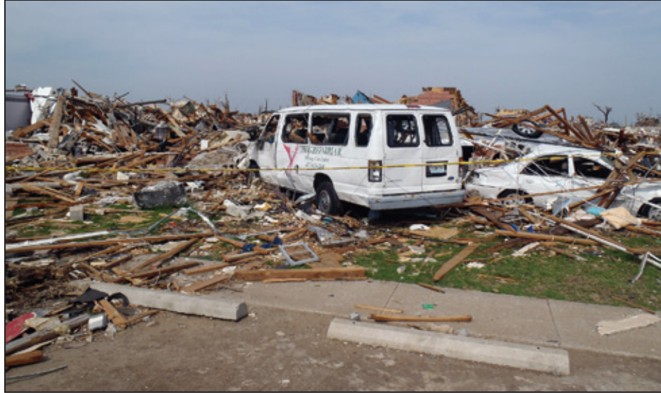
Figure 3-15: Large quantity of wind-borne debris covering the lawn of a nursing home in Joplin, MO
