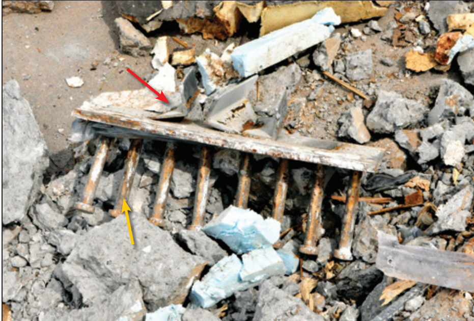
Figure 5-14: Example of weld plate and joist failure. The joist seat was torn from the joist (red arrow) and the anchor studs from embed plate were torn out of the concrete (yellow arrow) (Joplin, MO).
