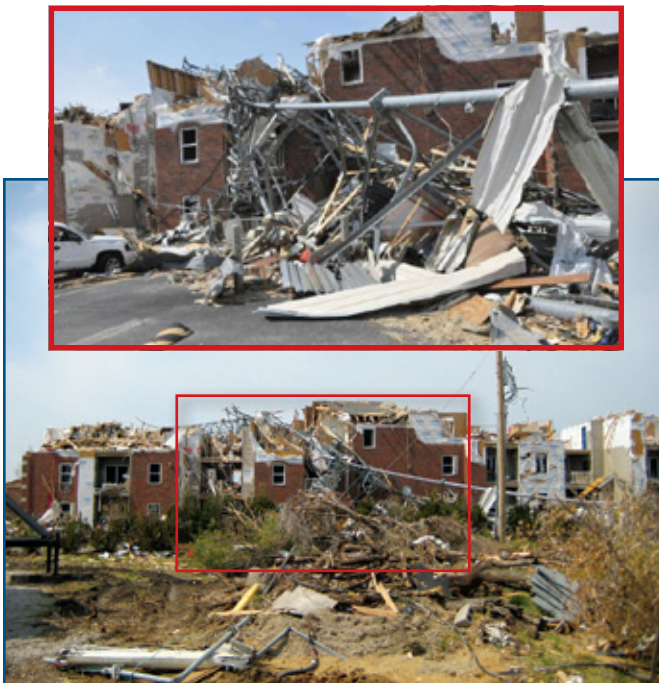
Figure 4: Collapse of a large communications tower onto a building in Joplin, MO (2011 Tornado)
