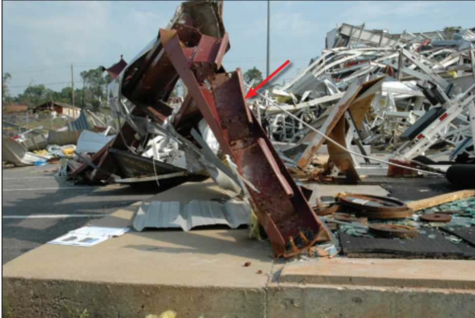
Figure 5-48: The anchor bolts of this base plate connection performed well while the weld along the base of the steel column failed (red arrow) (Tuscaloosa, AL)
