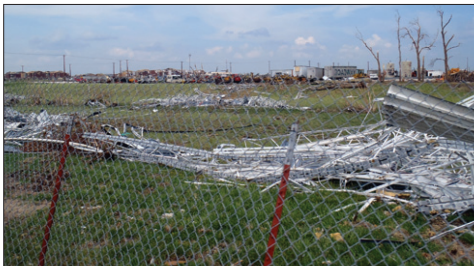
Figure 5-5: Field east of Home Depot with roof debris (Joplin, MO)
