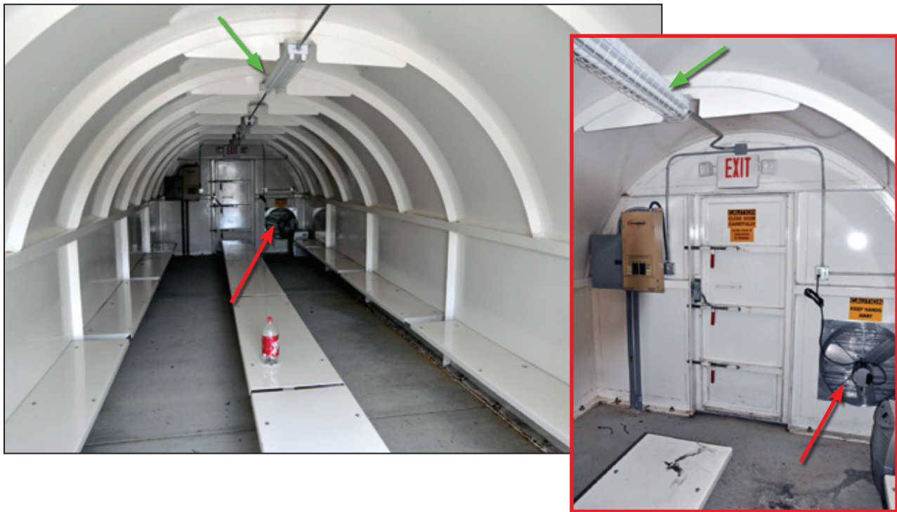
Figure 9-37: Interior of the community safe room shown in Figure 9-36 featuring seating, emergency lighting (green arrows), and ventilation (red arrows); inset is a close-up of the entrance door (Phil Campbell, AL)
