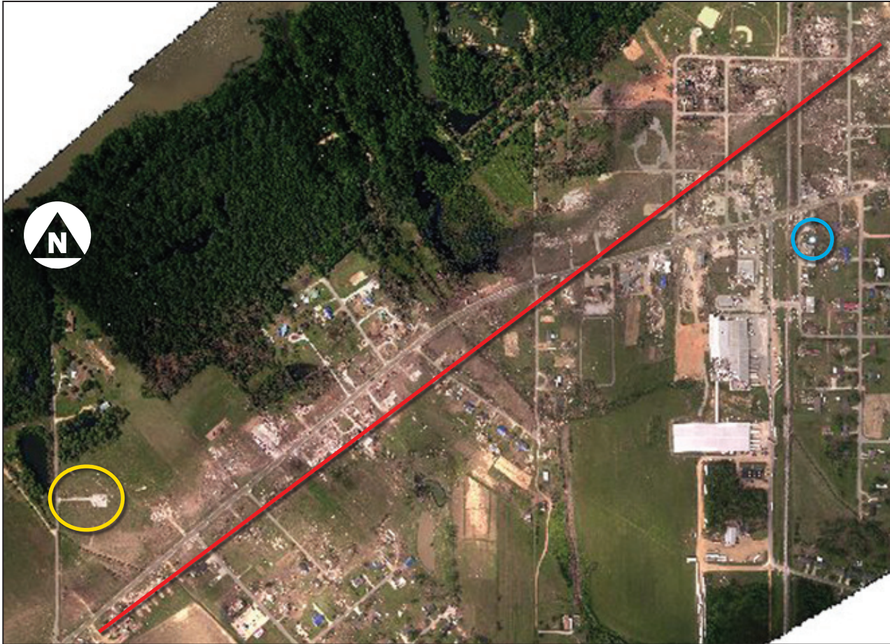
Figure 8-26: Aerial view of the 300-foot guyed cellular tower (yellow circle) in relationship to the approximate centerline of the tornado damage swath (red line) in Smithville, MS. The Smithville water tower shown in Figures 8-5 through 8-7 is northwest of the guyed tower and circled in blue for reference.
