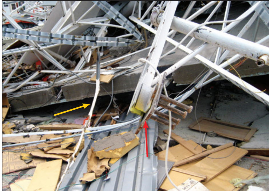
Figure 5-16: Example of a weld plate failure. Note the attached joist (red arrow) and the joist pocket at the top of the wall panel (yellow arrow) (Joplin, MO)
