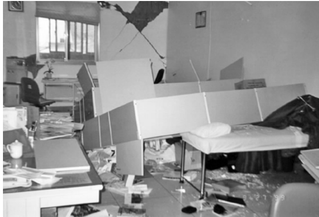
FIGURE C13.1-5 Toppled Storage Cabinets
